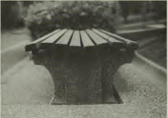
The original bench slat attachment detail on these contoured benches is both elegant and difficult to maintain. It is critical to develop a practical method of attachment that is consistent with the historic character of the benches.
