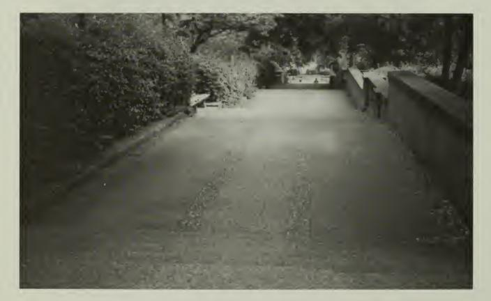
Above and above right: While the colors are not seen in these pictures, the tonal and textural differentiation created by polychromy in the concrete aggregate is nonetheless visible. It is critical that the colors and types of aggregates used in the historic concrete in the park be matched exactly in any new or repair concrete work.
