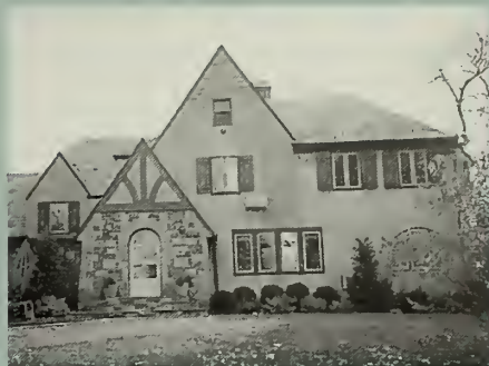
Inappropriate replacement windows dramatically affect the appearance of a historic home that once featured steel casement windows.
