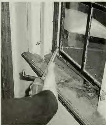
Figure 6. Pull bars were used to realign the sash from the inside. These custom made tools were especially useful on single sash units where the worker was unable to reach through an adjacent opening to apply pressure from the outside.
