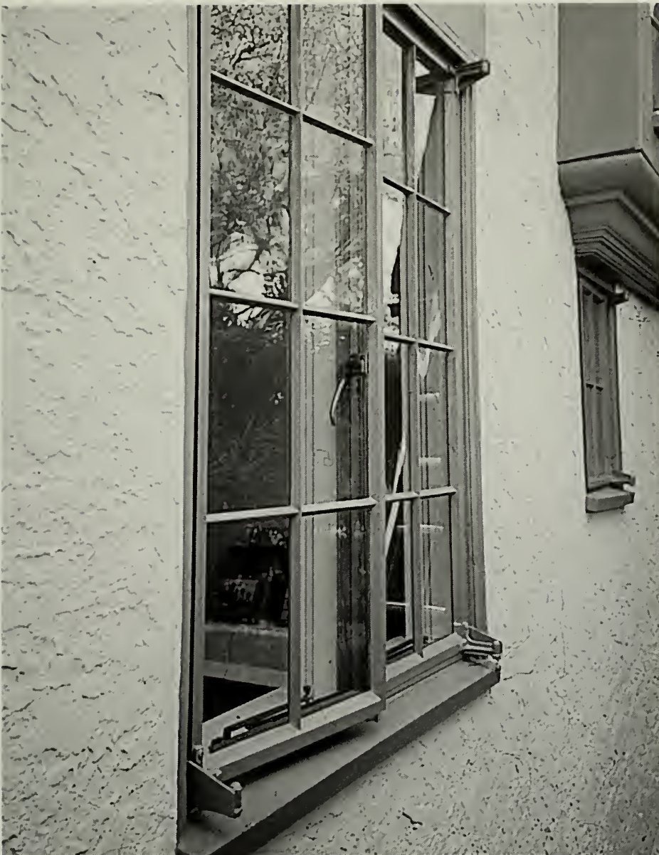
Figure 11. The completed work reveals the aesthetic appeal of the historic casement window – qualities appreciated both past and present.
