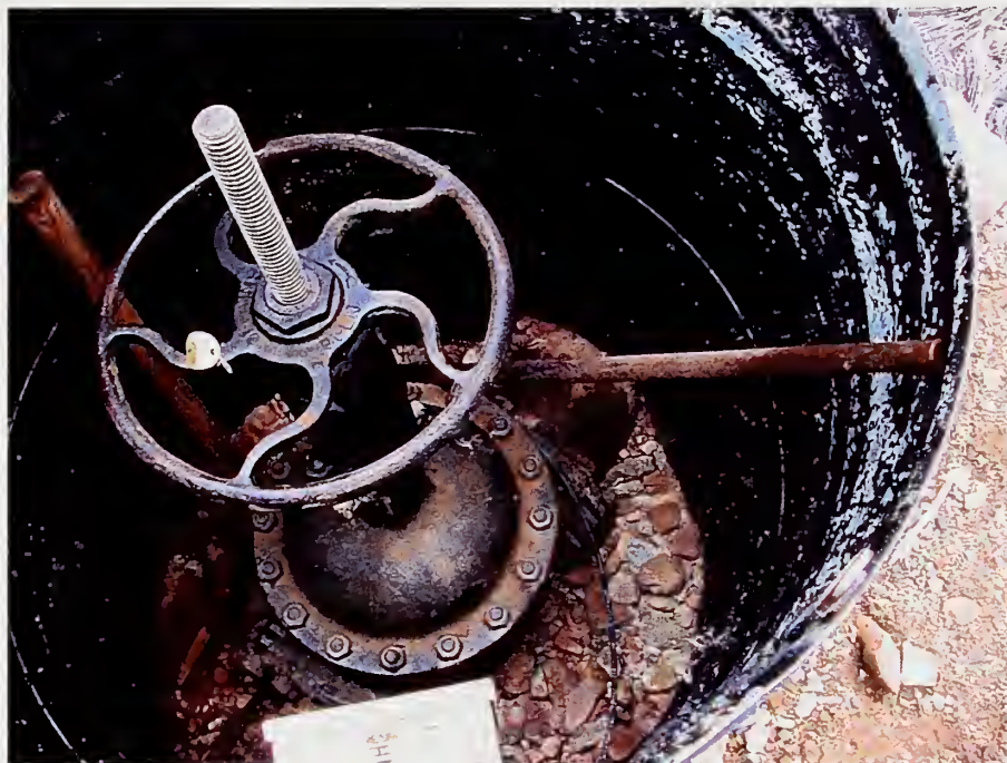
Figure 1. Typical valve box. Cast iron valve is electrically isolated from aluminum pipeline by insulated flange kits on each side of the valve. Cables are attached to the pipeline flanges and terminate in insulator bonding box (lower portion of figure). Isolation of the valve from the pipeline results in the aluminum pipeline being divided into electrically isolated sections.
