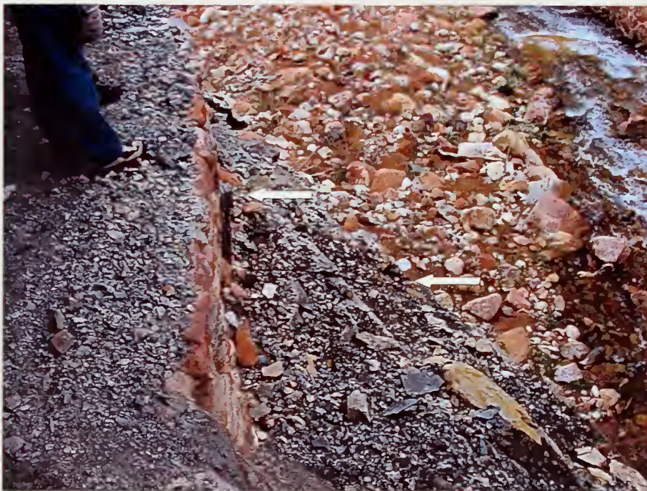
Figure 4. Test station at pipeline stationing 563+03. The test station (top arrow) is of a different design and materials than the original cathodic protection system materials. The test station does not have a rheostat or shunt and appears to connect an anode to the pipeline. The anode cable is exposed between test station and lower arrow, and is susceptible to damage.
