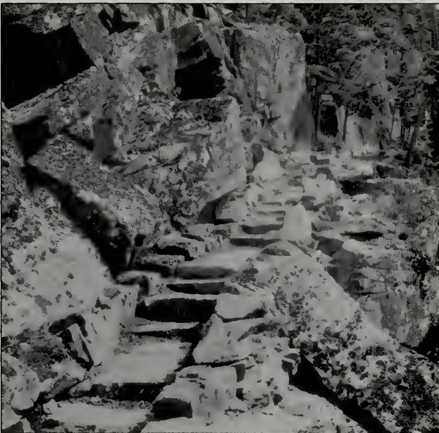
Fig. 42 Circa 1920 photograph of the Beachcroft Path, a memorial path funded by Mrs. C. Morton Smith, which provided an easy ascent of Picket Mountain [Huguenot Head] with long sections of rock paving, and fairly uniform, overlapping cut granite steps set firmly with extensive retaining walls. The trail was built in 1915 and later improved and endowed with a maintenance fund in 1926.
