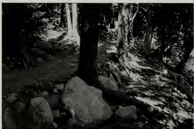
Fig. 144 Rehabilitated section of the Jordan Pond Trail in 2003 where tread was raised by building a wall with stones and roots then surfaced with gravel for an easy walking tread.
