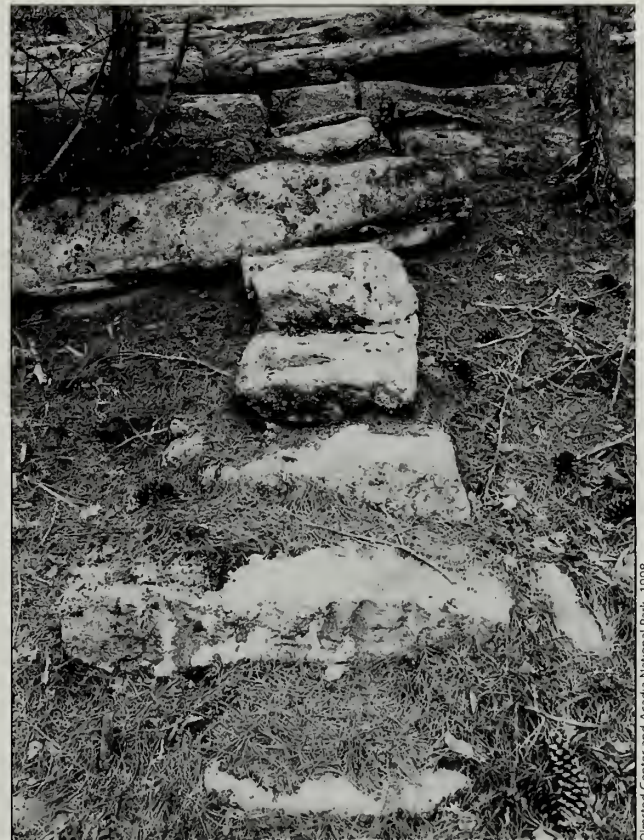
Figs. 30, 31 Waldron Bates improved the walking tread by piling loose stones into rudimentary retaining walls for a level, cross-slope surface and adding rough, uncut steps up steep slopes and between rock ledges. Bates-style work is preserved on the Eagles Crag Foot Path (#343) above and Potholes Path (#342) below, which were constructed in 1905 and 1906.
