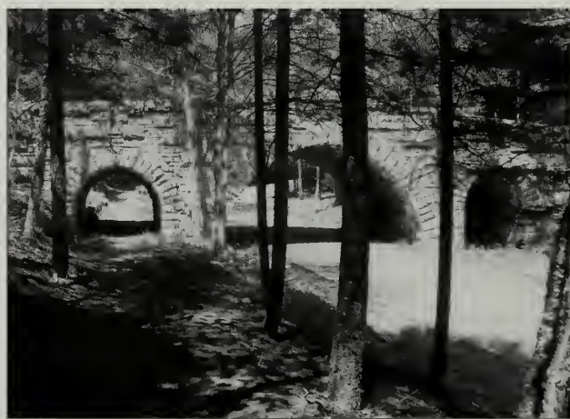
Fig. 75 Triple arched Stanley Brook Bridge allows Rockefeller's carriage road to cross over the Seaside Path (left), Stanley Brook Motor Road (center), and Stanley Brook (right). Steps connect the Seaside Path and carriage road (not shown).
