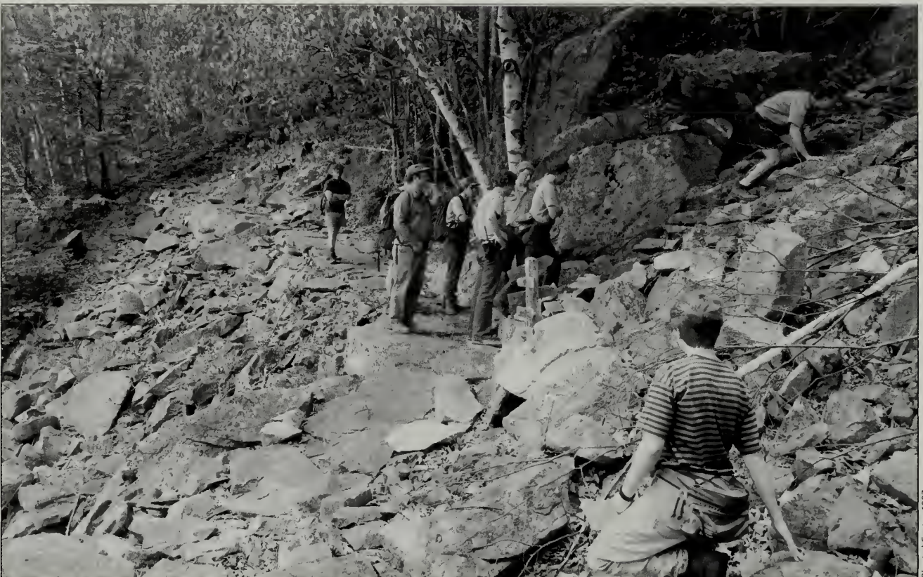
Fig. 52 The Orange and Black Path [on the section that is now the Champlain East Face Trail], laid out under the direction of Rudolph Brunnow in 1913, led walkers through geologically interesting areas including fissures, talus slopes, ledges, and boulders. A remarkable section of stone pavement curves in a 90-degree arc across a talus slope, with enormous slabs. A stone bench was destroyed by a rockslide in the 1970s.
