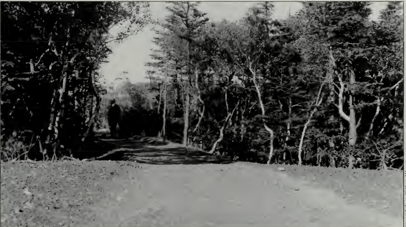
Figs. 100, 101 CCC photographs from circa 1937. The upper photograph shows the trail surface after it has been "swamped out," plants and roots removed, and the rough grade set with stone rubble. The lower image shows the path after it has been surfaced with screened gravel.
