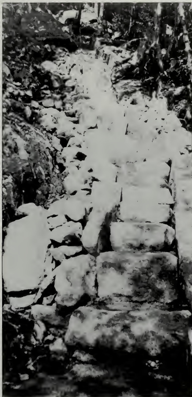
Figs. 111, 112, 113, 114 Improvements to the Ladder Trail by the CCC in 1934 and 1935. The upper photograph shows the crew quarrying stone for steps with hammer and chisel. The second image (left) shows a nearly complete section of rebuilt steps. The third image shows the crew moving large stepping stones with a gurney. The lower image shows the completed trail entrance.
