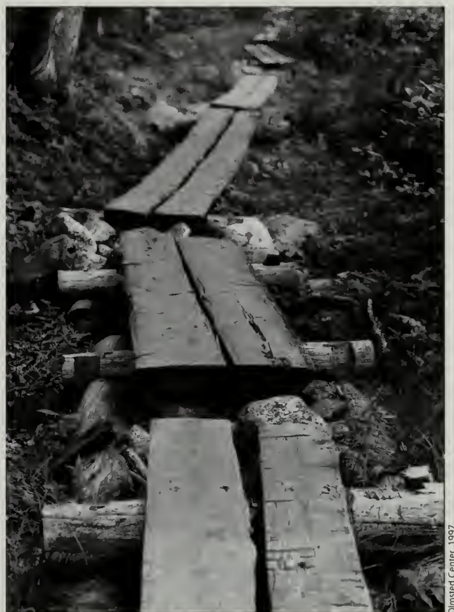
Figs. 131, 132 Boardwalks were laid over the Jordan Pond Path on the western side of the pond in the 1980s to minimize erosion caused by an increasing number of hikers.
