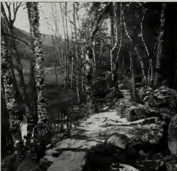
Fig. 38 The Kane Path, built along the western shore of The Tarn, connected the Ladder Path and Canon Brook Path with the Sieur de Monts Spring area. Large flat stones, currently described by the trails crew as “stone pavement,” became a popular construction technique for a level, rustic, elegant, and durable walking tread. Circa-1916 photograph.
