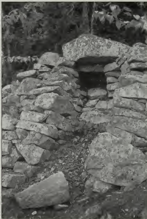
Figs. 102, 103 On the Perpendicular Trail, the CCC built inside drainage ditches lined with stones (left) to direct water into catch basins and under the trail by closed culverts (right).
