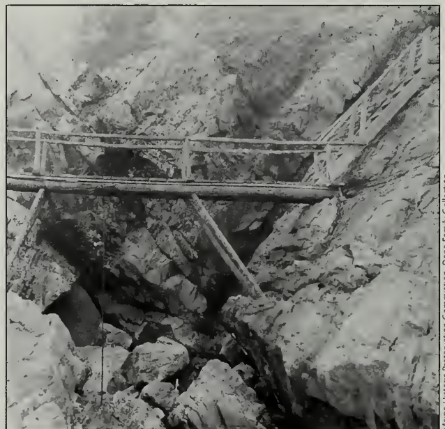
Fig. 64 Circa-1908 photograph of a bridge built of cut boards and rough-hewn logs along the rocks near Seal Harbor.
