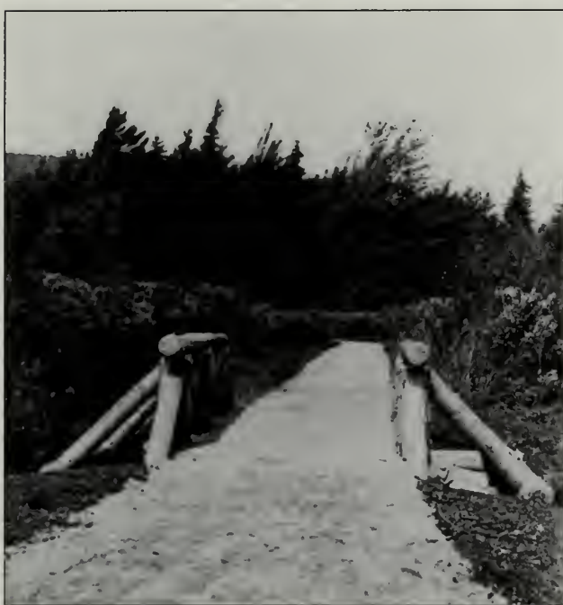
Figs. 104, 105 Typical CCC-style bridges constructed in the Great Meadow near Sieur de Monts Spring. Cedar logs were set on a dry-laid granite block foundation (above). The bridges were then surfaced with gravel to provide an uninterrupted walking tread (below).
