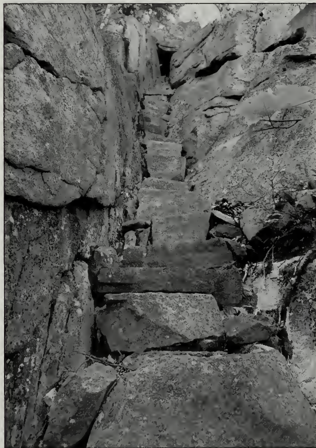
Fig. 54 Steps on the Orange and Black Path [on the section that is now the Champlain East Face Trail], wedged between boulders to wind through ledges and fissures.
