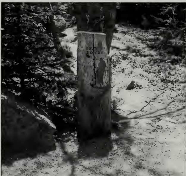
Fig. 135 Cedar post signs, introduced to the trail system by Gary Stellpflug in the 1980s, reduced theft and vandalism of trailhead signs. Very successful and durable, cedar post signs have been installed on all marked trails in the park.
