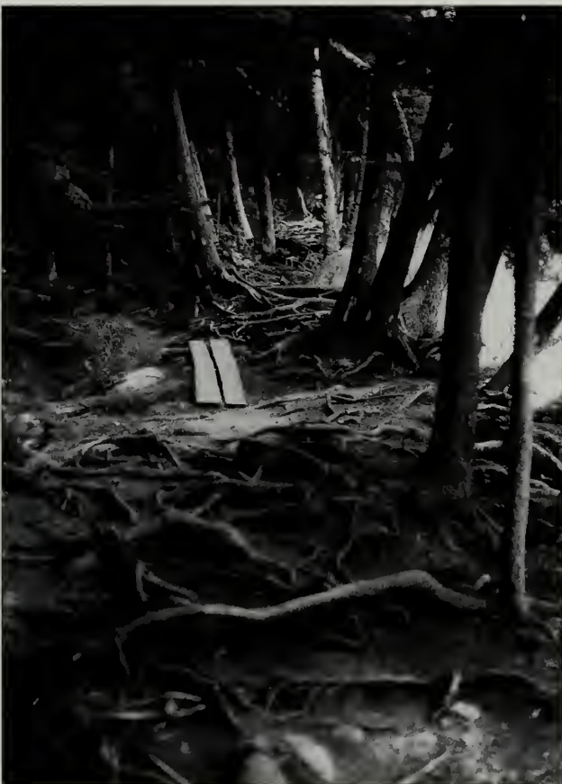
Figs. 131, 132 Boardwalks were laid over the Jordan Pond Path on the western side of the pond in the 1980s to minimize erosion caused by an increasing number of hikers.
