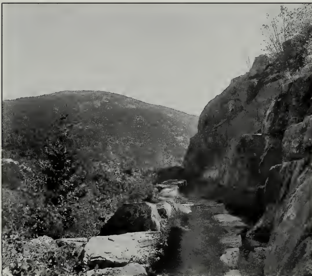
Fig. 45 Like earlier path builders, Dorr routed the Emery Path through rock formations. The path leads walkers comfortably along exposed ledges of what Dorr named the "Sieur de Monts Crag." Large stones, part of the outer retaining wall shown above, rest upon a crib of iron pins, invisible to walkers as seen in circa 1920.
