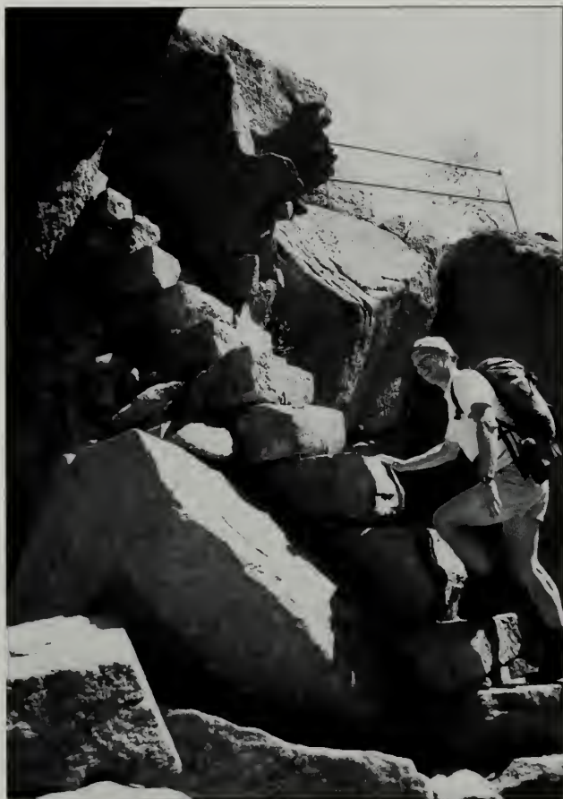
Fig. 53 The hanging steps on the Orange and Black Path. The iron railing above lines an overlook; iron pins hold the slab laid steps.
