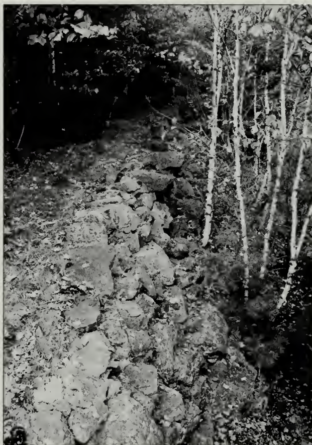
Fig. 81 The Gurnee Path, between Bar Harbor and Hulls Cove, was funded by Augustus Gurnee and endowed with a maintenance fund by his three daughters. Completed in 1926, path construction included extensive retaining walls and rubble fill to create a level walking tread. A wooden railing and benches were placed along a high ledge overlooking Frenchman Bay. The path is no longer marked but easy to follow.
