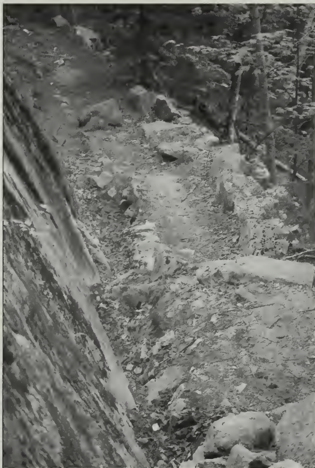
Figs. 102, 103 On the Perpendicular Trail, the CCC built inside drainage ditches lined with stones (left) to direct water into catch basins and under the trail by closed culverts (right).
