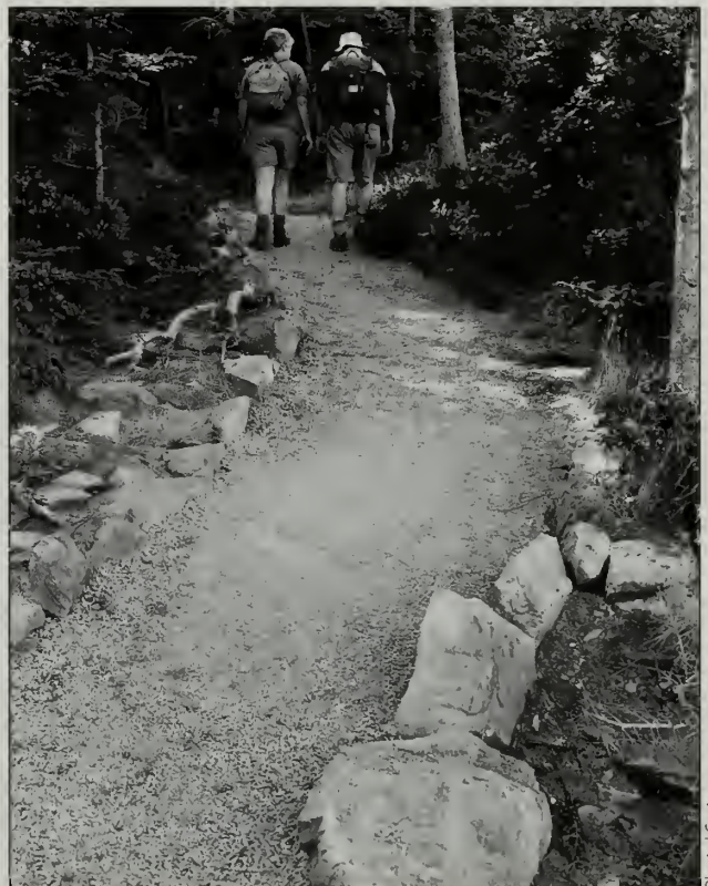
Figs. 141, 142 An eroded section of trails is repaired with checks, wall, and rubble infill (above). The stonework is covered with gravel and the edges revegetated (below) in 1997.
