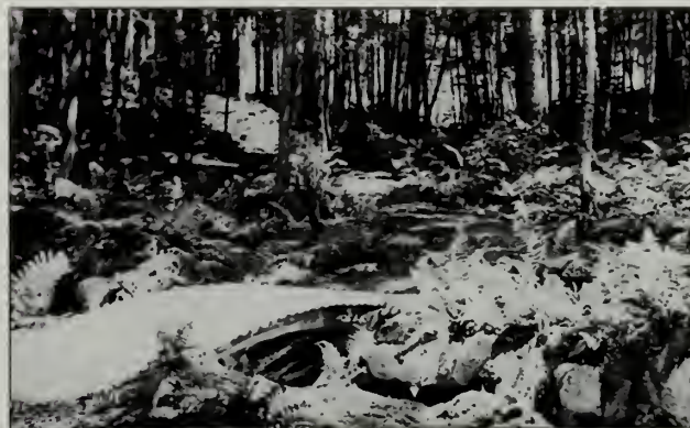
Figs. 104, 105 Typical CCC-style bridges constructed in the Great Meadow near Sieur de Monts Spring. Cedar logs were set on a dry-laid granite block foundation (above). The bridges were then surfaced with gravel to provide an uninterrupted walking tread (below).
