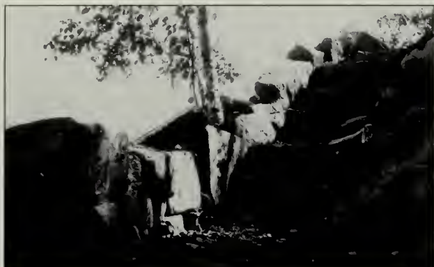
Fig. 115 A circa-1934 photograph of the Perpendicular Trail illustrating the large stone used for steps and coping to prevent heaving by ice and frost. The steps and coping are still in good condition.
