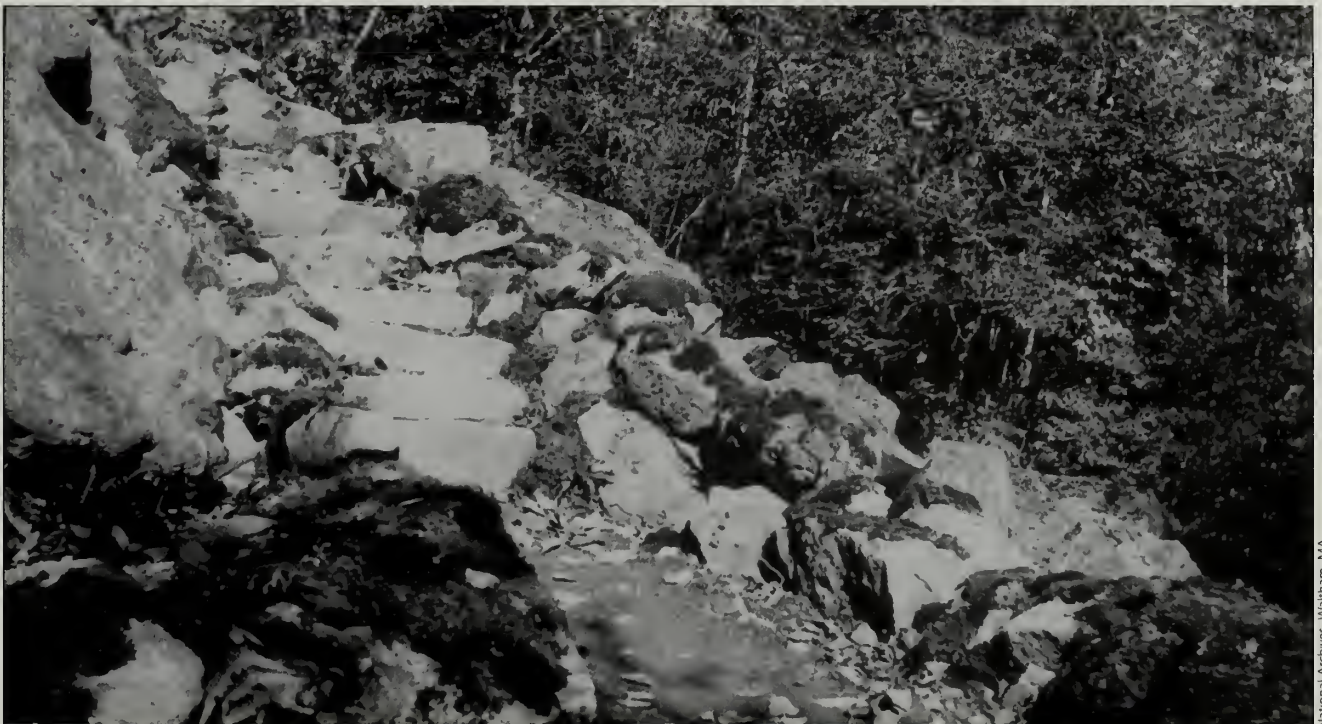
Fig. 96 On the Perpendicular Trail, CCC crews in the 1930s covered stones with transplanted moss and ferns to blend new construction with the natural surroundings.
