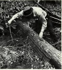
Heavy rains bring high water in the tiny branches that feed trout streams, and the water flows over the road when the culvert is full, causing erosion (top) on Hoods Creek. To keep the silt from getting into Hoods Creek, wire silt trap (above) will trap leaves and strain the silt from the water before it reaches the main stream.
