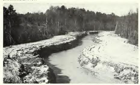
Downstream from the straightened section shown on the cover, a ruined Marbury Creek in Barrow and Oconee counties near Winder shows the scars of recent channelization in 1966. First, bulldozers removed trees on the banks 30 to 100 feet back on each side, followed by dredging of the stream bed with draglines, and spreading of the dredged material by bulldozers.
