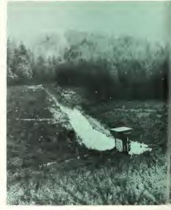
Today, Jones Creek disappears into a 420 foot long cuivert through the base of the dam at the end of a raw channelized ditch. Since no water is permanently impounded by the dam, the temperature of the water below it is not warmed too much for trout, the usual result of building an upstream lake on a trout stream. However, adult trout upstream migrate downstream through the pipe and are unable to return later to spawn, a serious blow to fishing in the once productive upper section.
