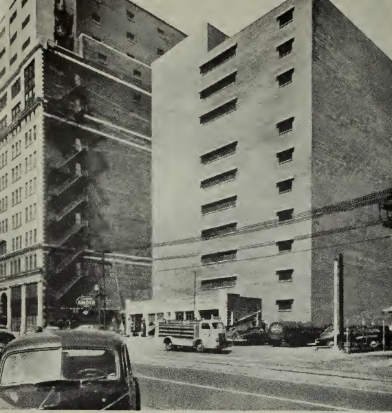
Southern Furniture Exposition Building in High Point, to which a 66,000 square foot addition to cost $460,625 is being built. Two formal and two informal furniture shows annually draws buyers from all over the U. S. to the South's furniture center.
