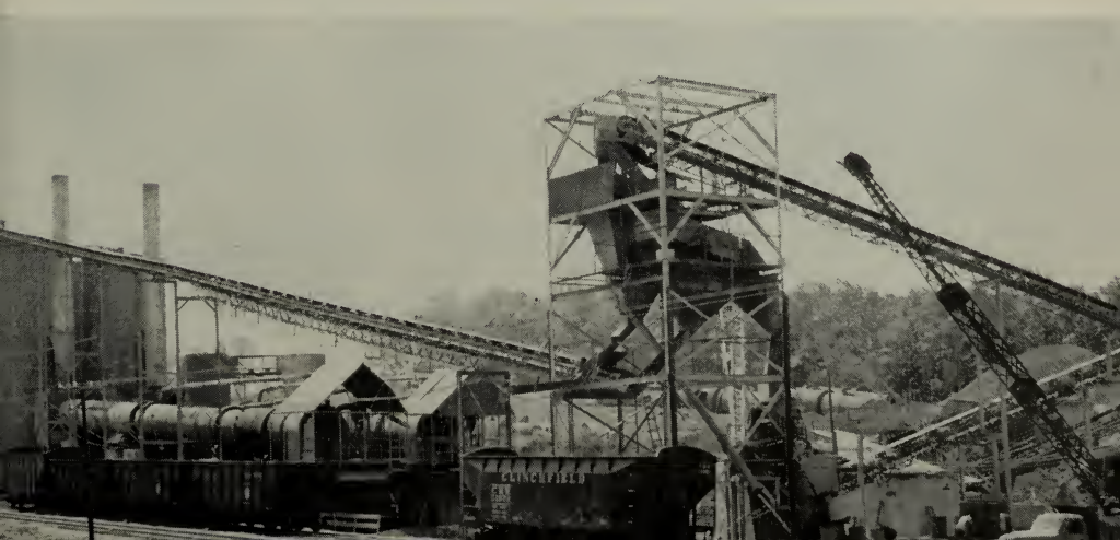
Manufacture from mineral products—A modern lightweight aggregate plant.
