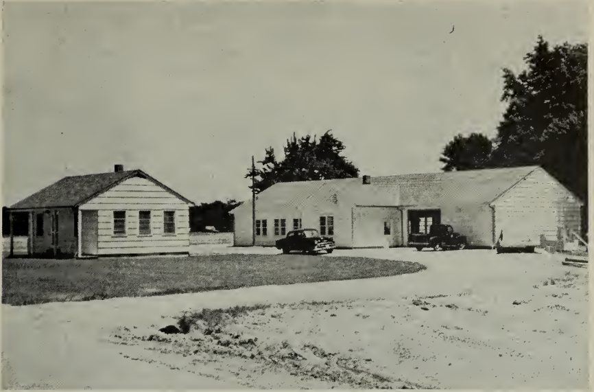
Office and packing shed constructed at the newly purchased Little River Nursery in Wayne County, authorized by the General Assembly of 1953. Production capacity of the Nursery will be between 20 and 25 million forest tree seedlings per year when fully developed.
