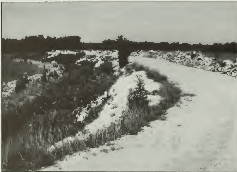
Figure 23. Top and side view of the Burcham's dike. Leach.
