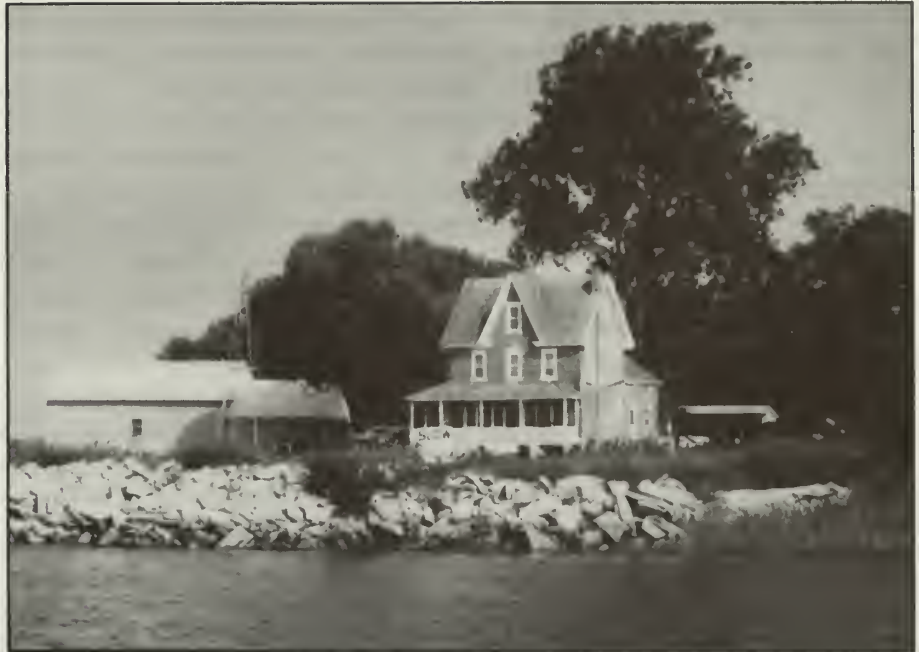
Figure 22. Front view of Burcham House with dike in the foreground. Sebold.
