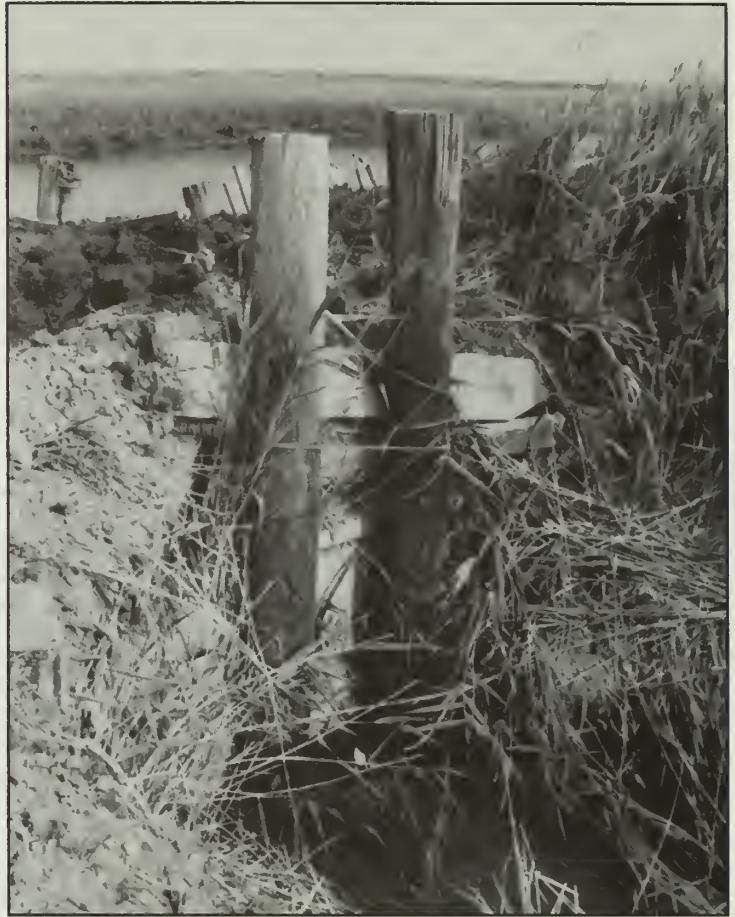
Figure 19. Example of the supports that surround a modern clapper valve sluice gate. Sebold.
