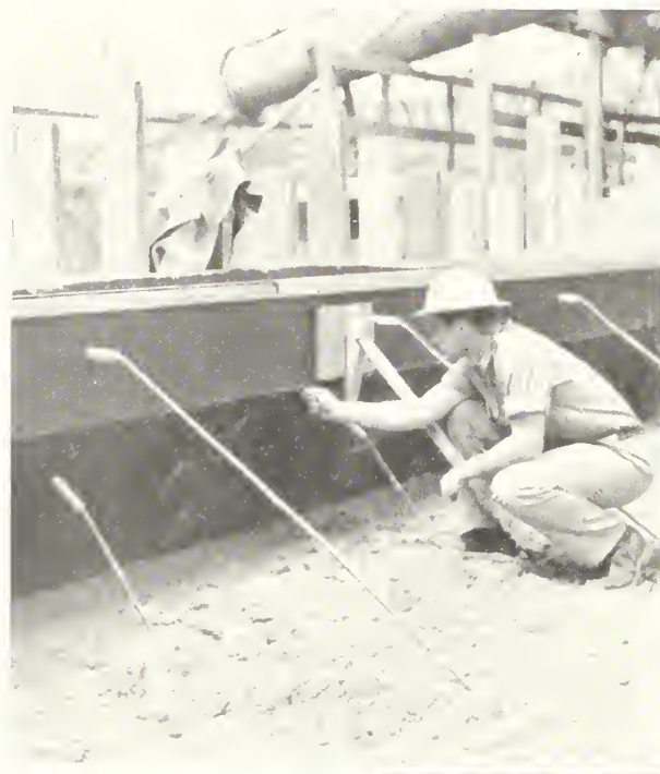
Built up form, lined with absorptive form lining—two layers of concrete in place. Note form rods in pipe braces
