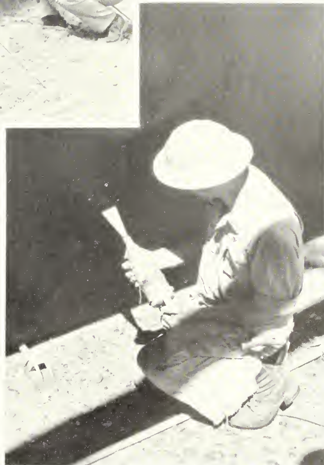
Portable electric drier used for removing moisture from absorptive form lining immediately prior to concrete placement
