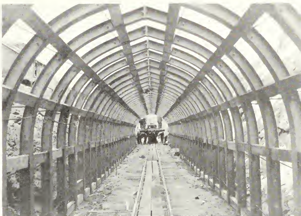
Tunnel supports control loose rock. The jumbo is used for drilling tunnel
