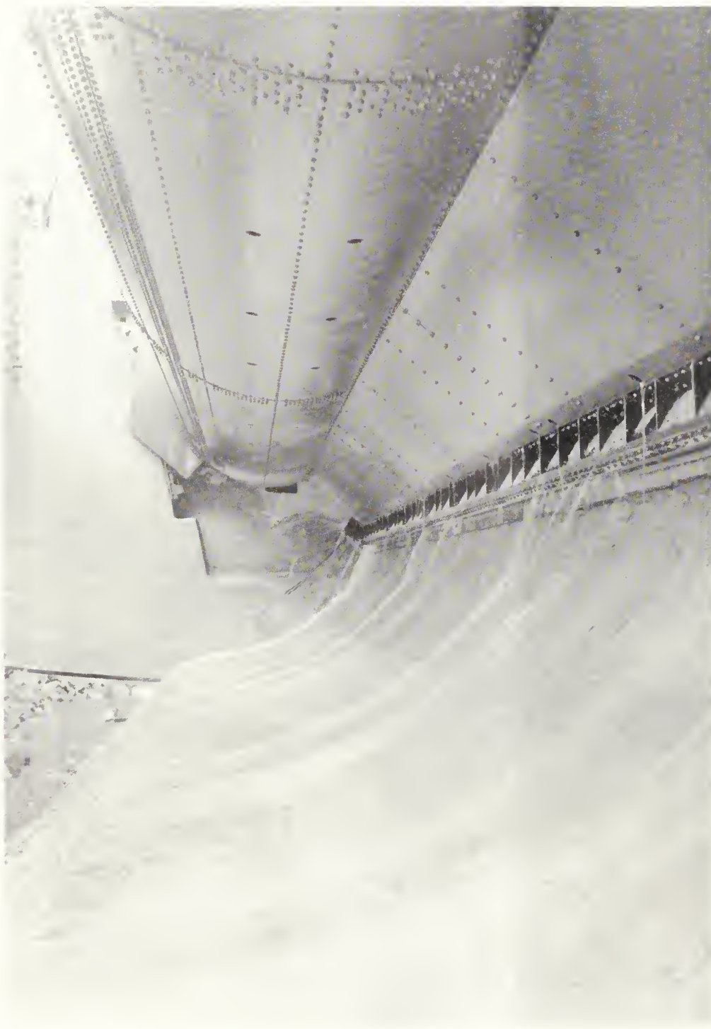
West roller gate of diversion dam closed tight, showing slight leakage
