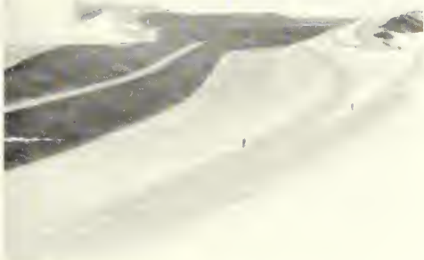
The deepest cut, 100 feet, in the Sand Hills section. Operation of the All-American Canal has answered "No" to the question, "Will blown sand fill up the big ditch?"
