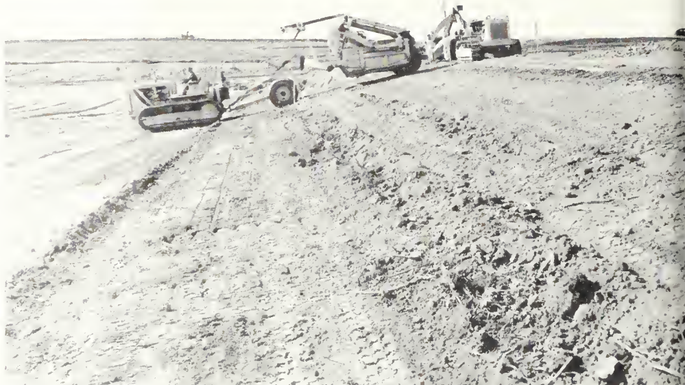
Constructing 8-foot fill 2 miles east of Buford, N. Dak.
