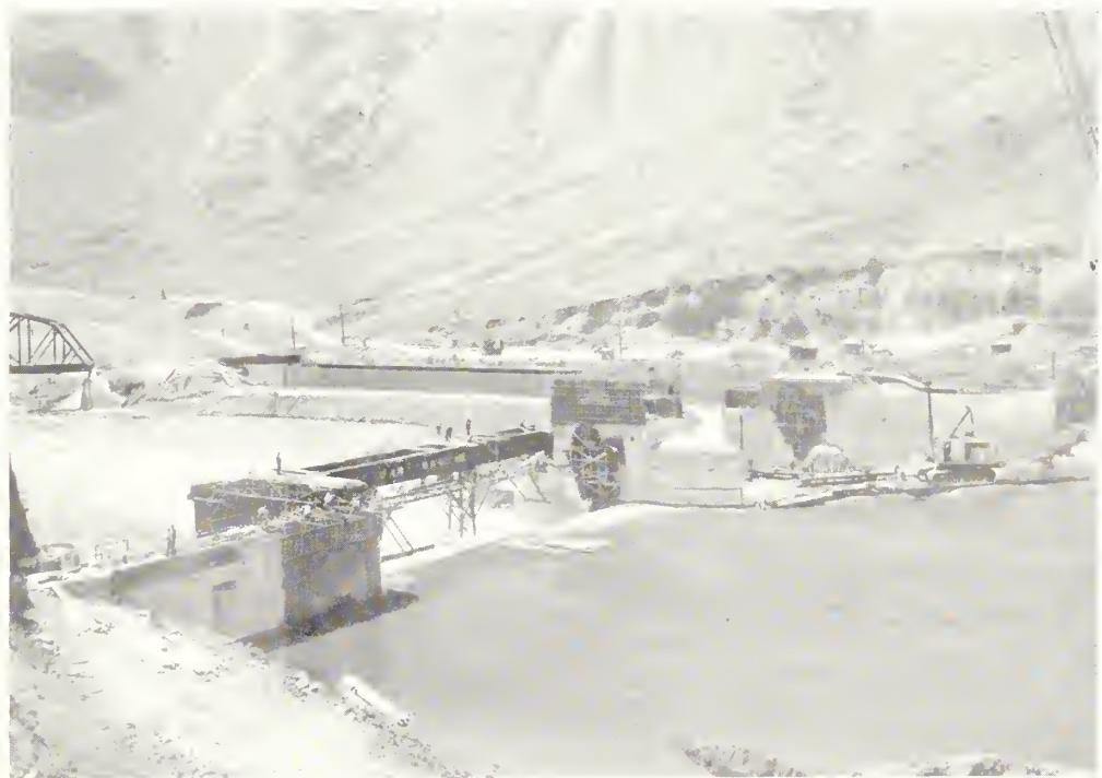
Roza diversion dam from service road on east side. Left to right: Pier 3, service bridge girders, piers 2 and 1, and canal headworks. Bench flume in background
