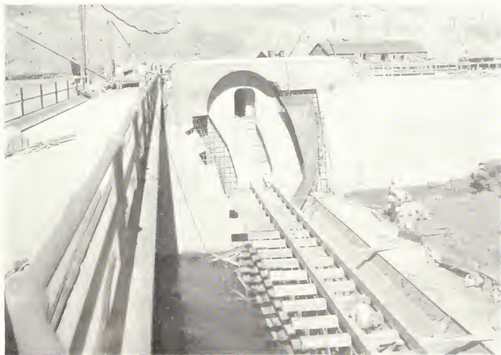
Falsework for the installation of roller gate between piers 1 and 2
