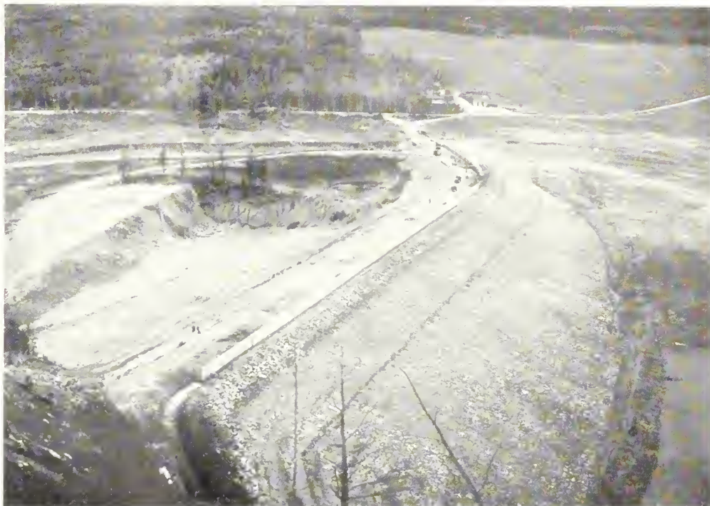
Construction of concrete parapet and curb walls on Moon Lake Dam
