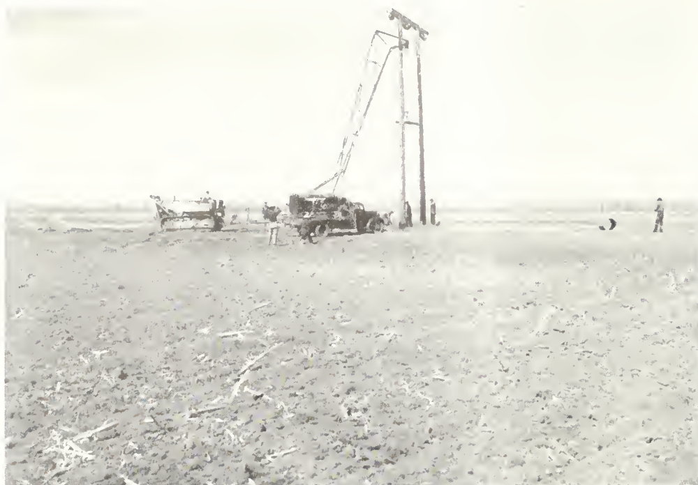
Greeley-Fort Morgan transmission line. Pole-setting operations; Structure No. 459 being placed in position ready for guying and backfilling holes
