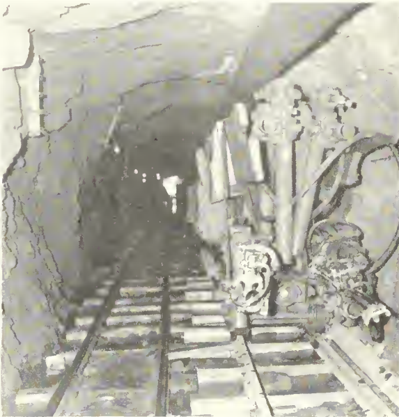
Looking into the Duchesne River Tunnel. Upper shows four water Leyner drills on passing track
