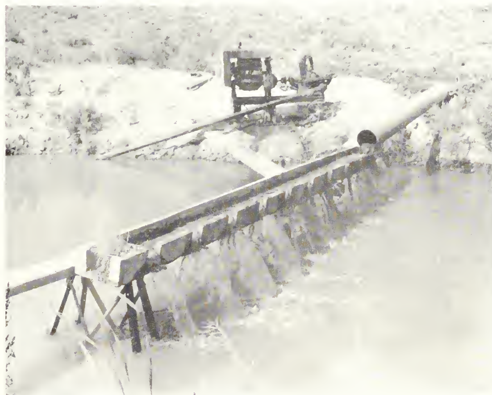
Rectangular openings in the wooden trough distribute the silt. Note the engine and pump with intake pipe in background
