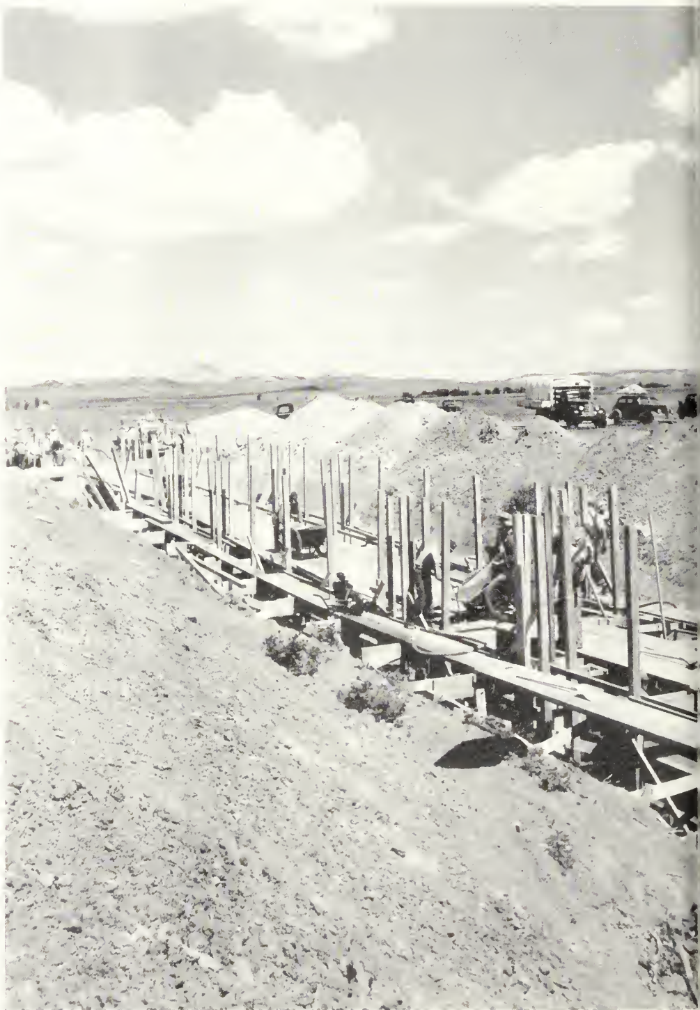
Pouring concrete for the 6- by 5-foot culvert
