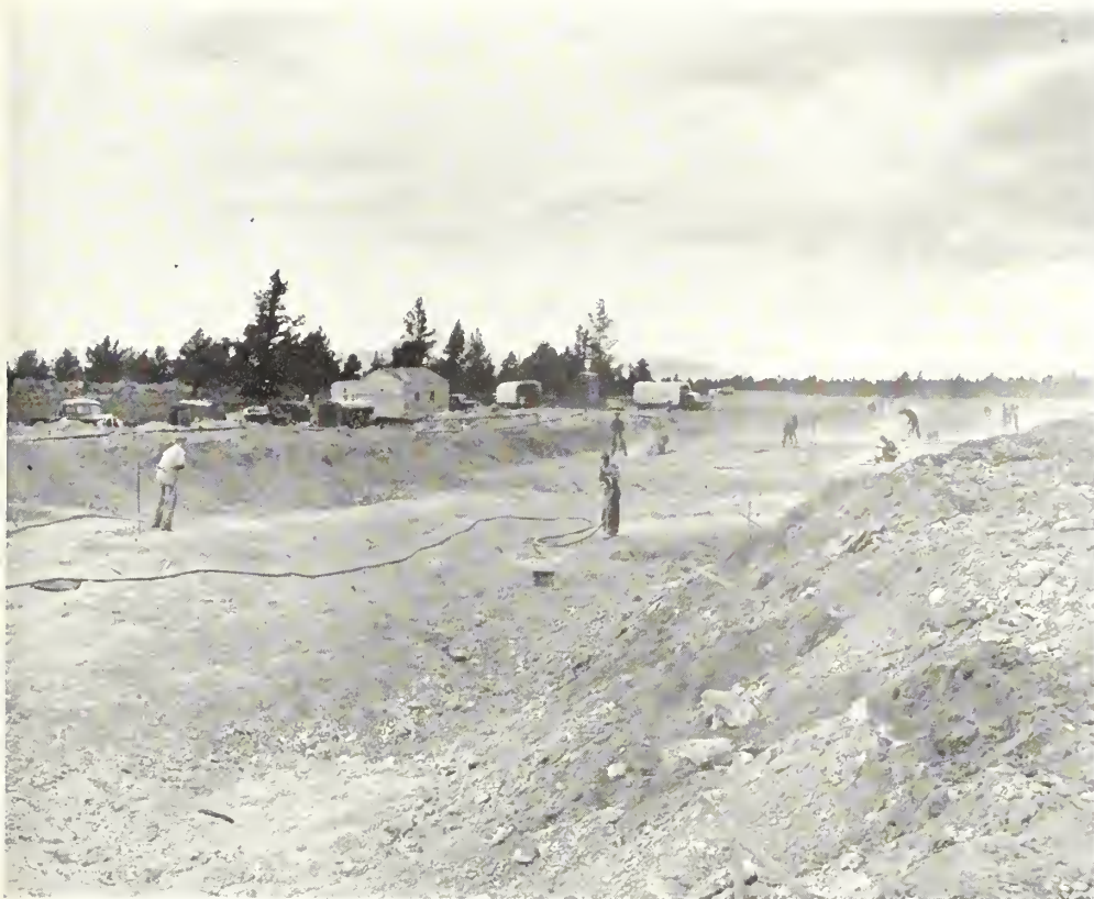
Drilling rock in the North Unit Canal of the Deschutes project, following stripping of earth cover
