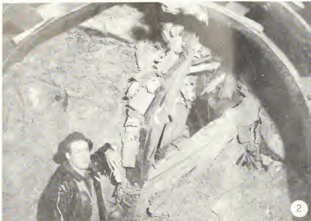
Alpine heading of tunnel showing failure of 6-inch steel supports where material on left side moved in 6 feet in 3 days
