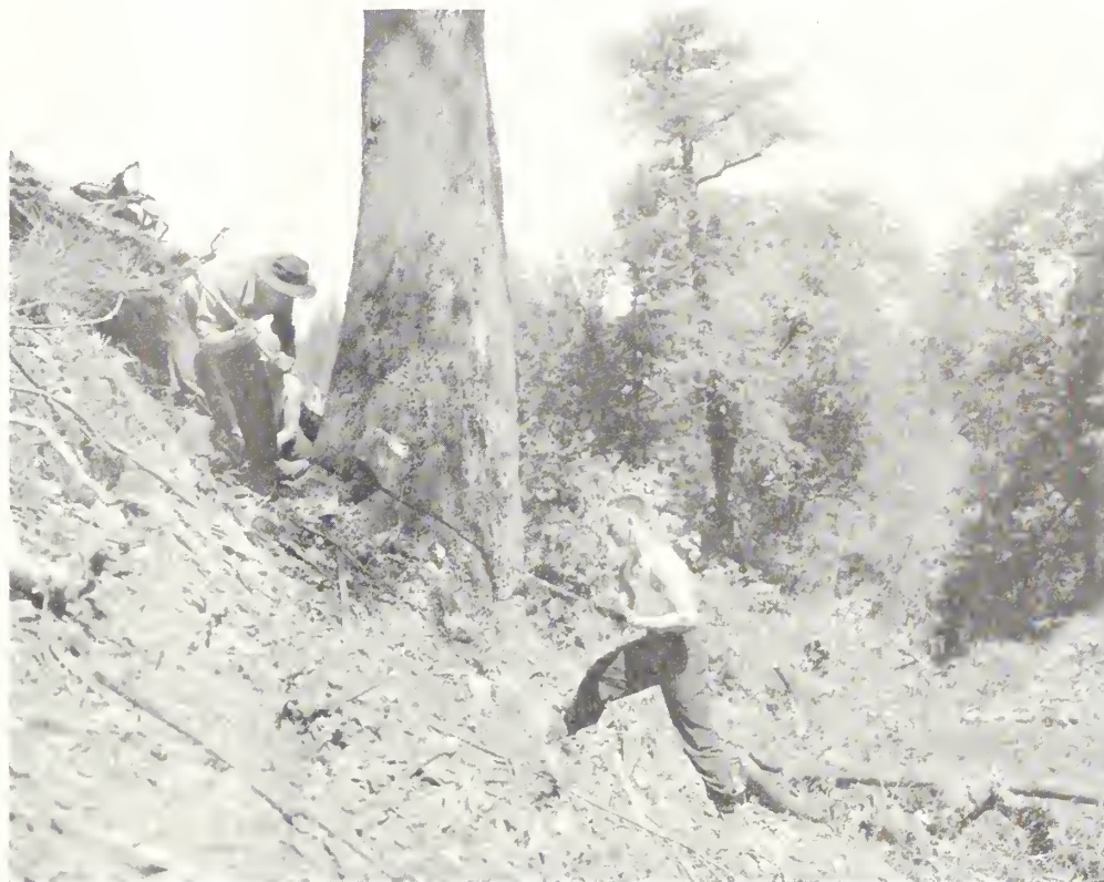
CCC enrollees felling a large oak in clearing operations along McCloud River. Two are working a cross-cut saw while another drives the wedge
