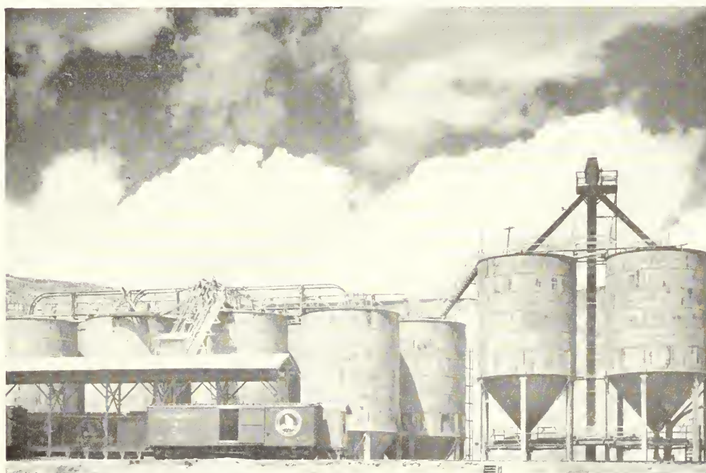
Cement storage silos and unloading platform, Grand Coulee Dam.
