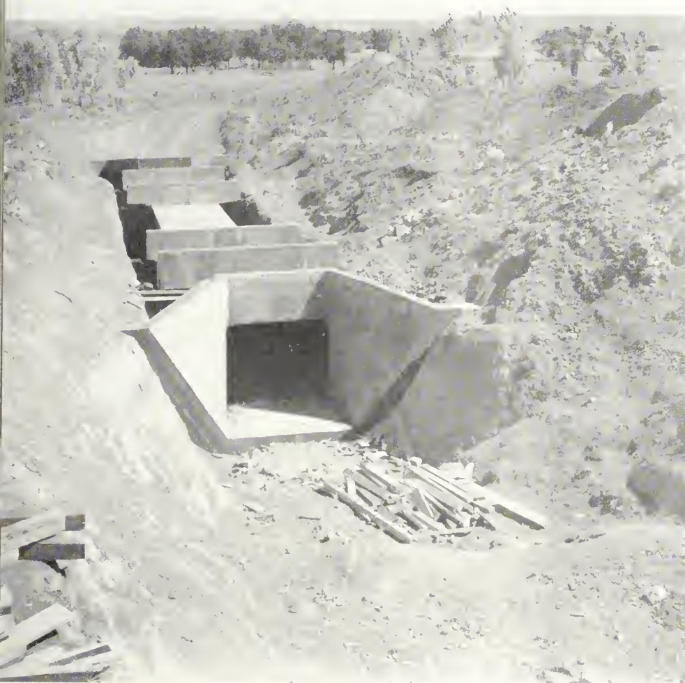
View of 6- by 5-foot culvert
