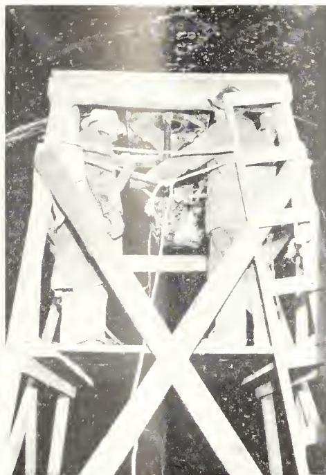
Drilling jumbo showing drill bolted to metal plate working in the arch of Tunnel No. 3
