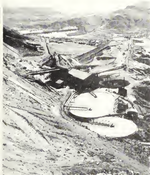
Gravel processing plant where sand and gravel are screened, washed, and stock-piled
