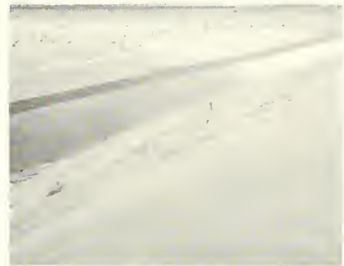
The bulge on the canal berm marks the maximum movement of drifting sand into the canal. No trouble has been caused so far, and it will be many years before wind-blown sand must be removed.
