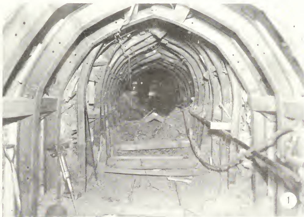
Replacing 4-inch steel supports with 6-inch sections shown in foreground. Alpine-Draper Tunnel
