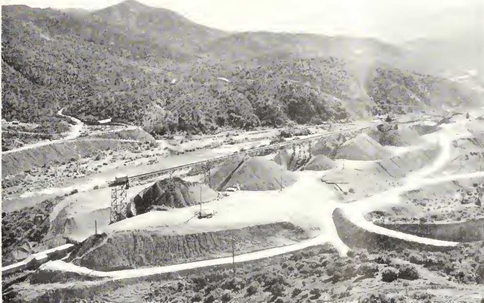
Aggregate storage bins at Coram. A portion of the aggregate conveyor system is in the background
