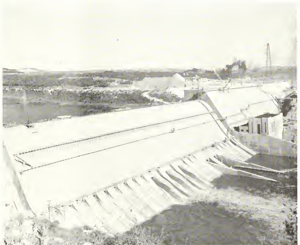
Downstream face of Marshall Ford Dam. Discharge of water is seen through five of the 8-foot 6-inch diameter outlets. Three of the outlets opened are of "Beaver Tail" type and two the regular circular type of openings
