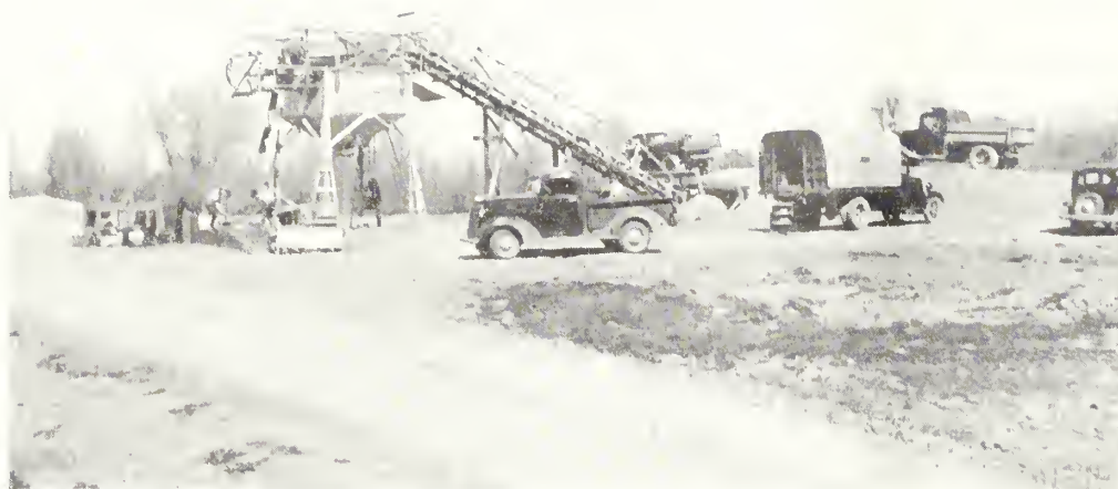
C.C.C. equipment at gravel screening plant
