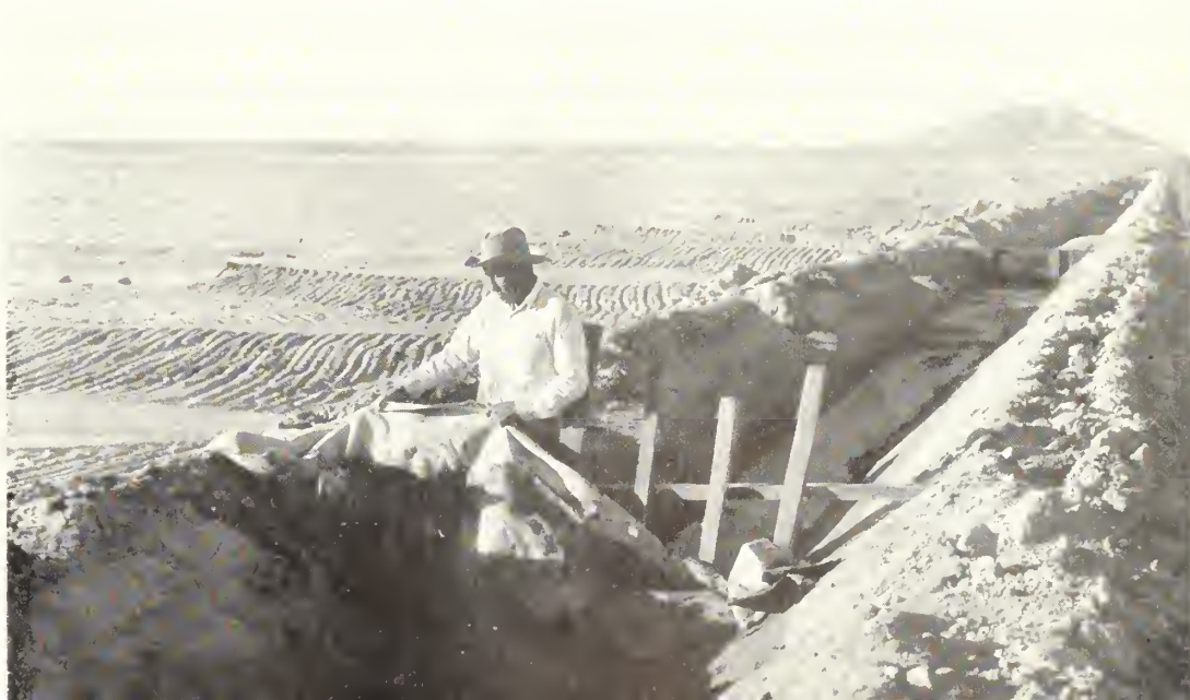
Pima Indian on the Gila River Reservation installing a tampon in an irrigation ditch, Arizona
