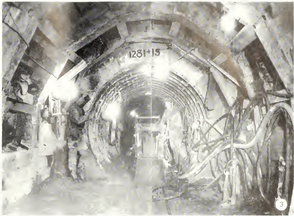
Alpine-Draper Tunnel showing 12- by 12-inch 7-segment timber sets and 4- by 6-inch spiling. Concrete used as spreader between posts at base to prevent twisting of timber
