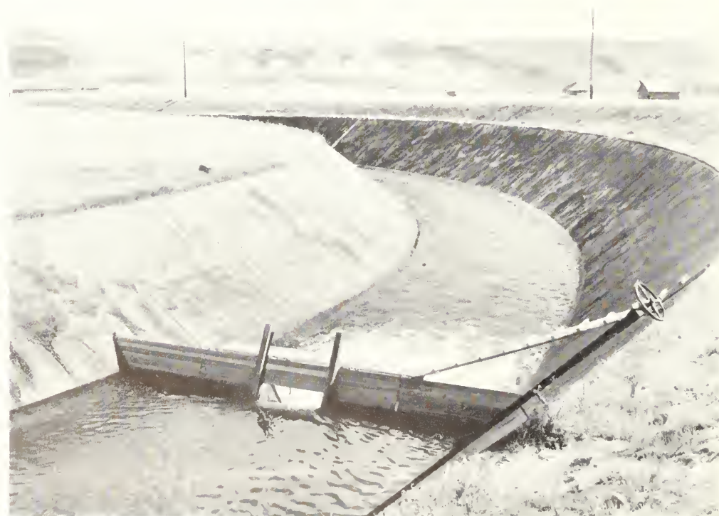
First water coursing through the Yakima Ridge Canal. The temporary weir was needed to handle the small head at the start.
