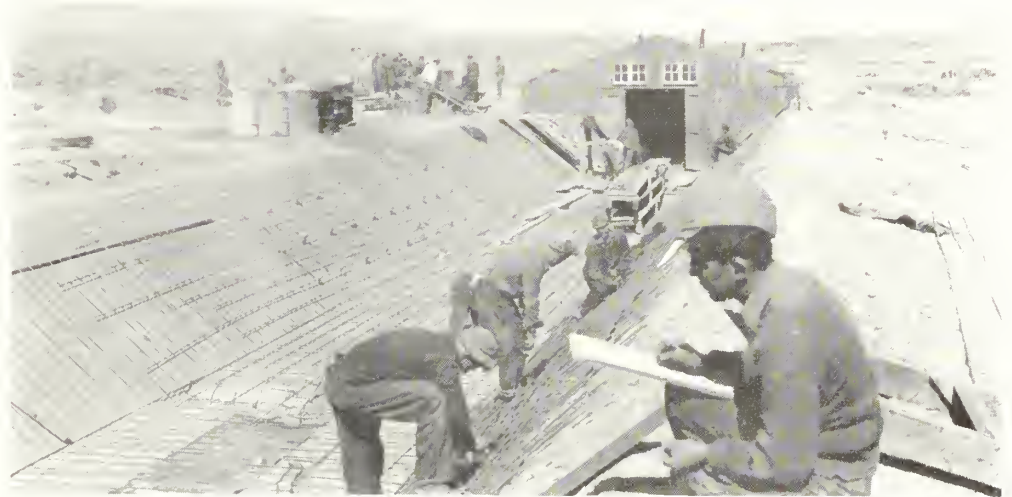
Movable shelter for concrete protection in use on Alkali Creek inclined drop reconstruction
