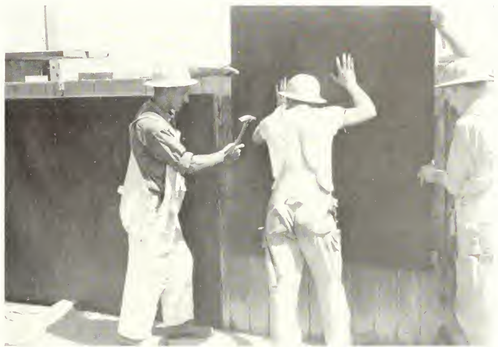
Placing absorptive form lining on upstream face form
