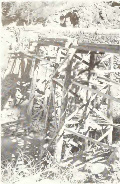
Temporary timber substructure erection for replacement of a portion of the Tieton Main Canal
