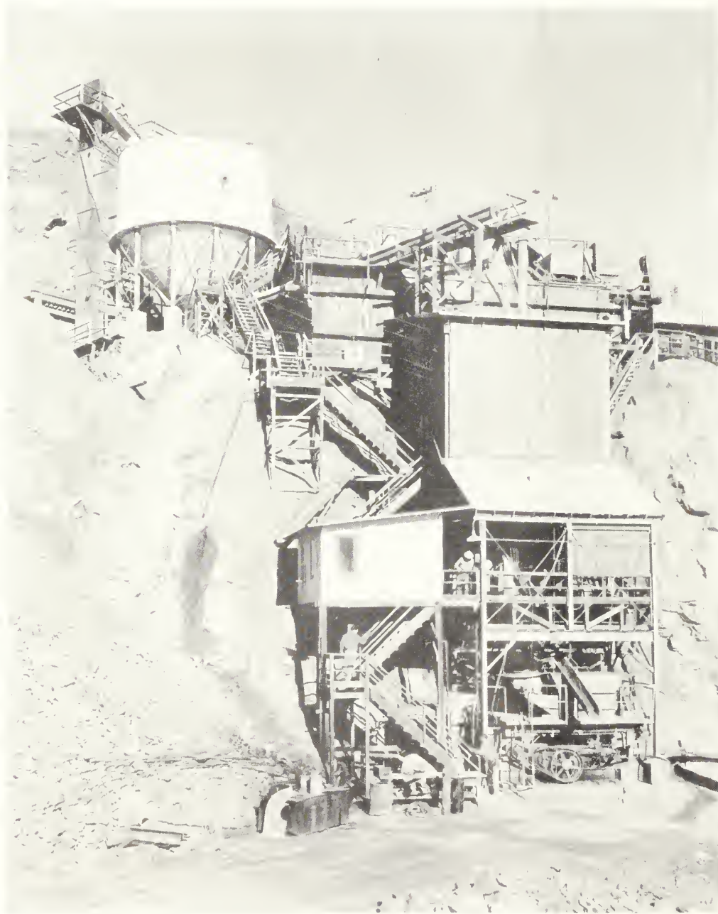
Concrete batching and mixing plant at Parker Dam power project
