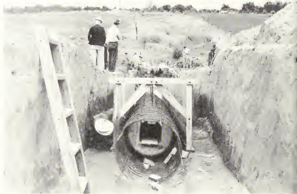
Orchard tracts pipeline under construction, showing method of suspending forms and reinforcing steel
