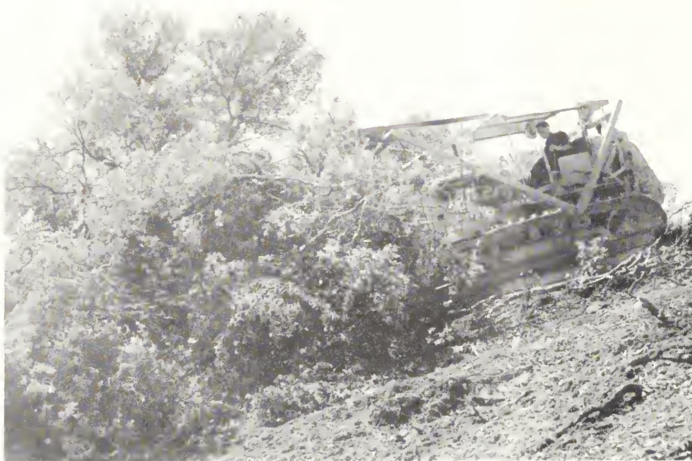
Clearing reservoir by CCC on Squaw Creek slopes. Tractor is used to remove and pile brush for burning
