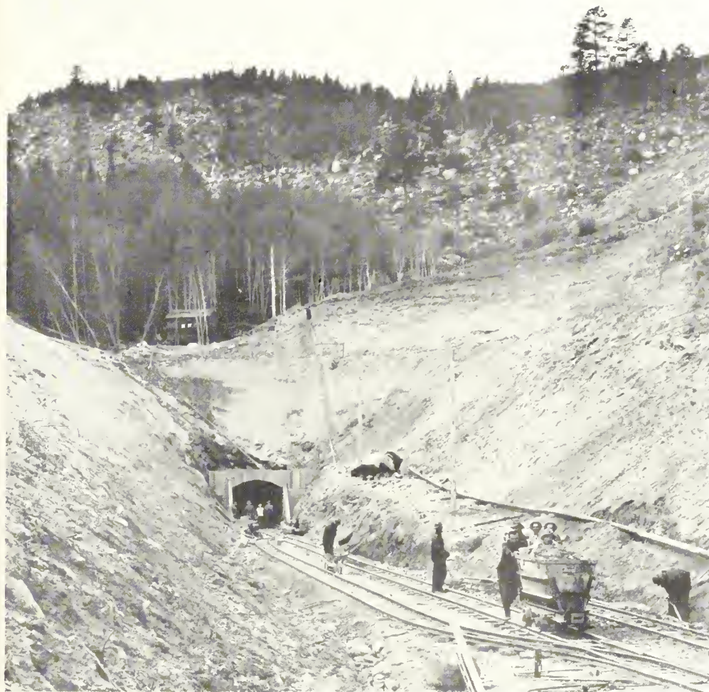
East Portal of the Continental Divide Tunnel. Excavation operations in the preliminary stages, and pushing of a loaded car by hand
