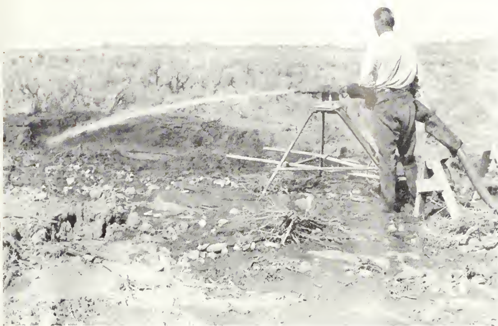
The jet is played to cut and mix the earth with the water
