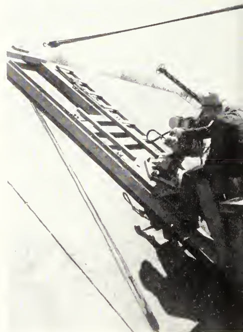
Core drilling on canal sideslope showing drilling head fastened to sliding plates, rails, and raising rope block
