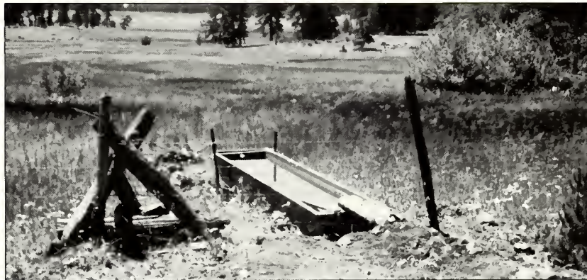
Figure 3-2—Spring development with water piped to a watering trough.
