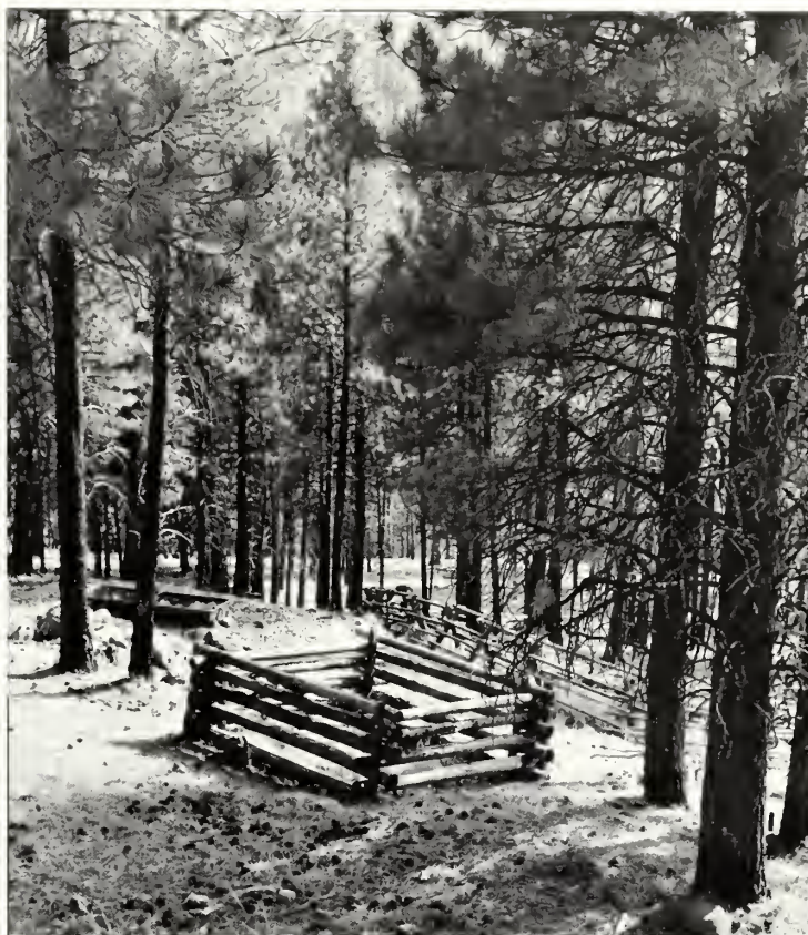
Figure 8-8—Spring development with fenced water source and water piped to a trough.
