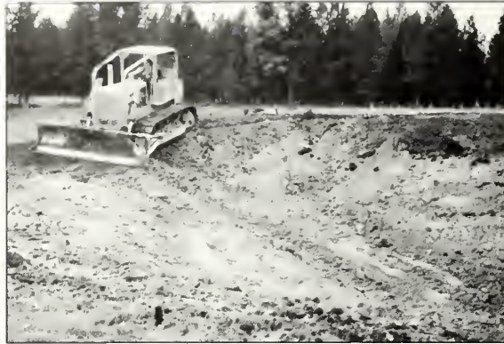
Figure 8-10—Constructing a stock pond with a bulldozer.
