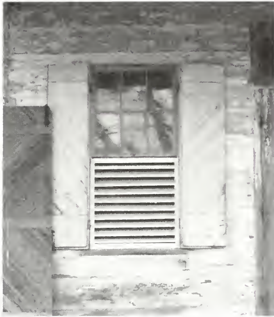
Figure 24 View of front window, W-2, with temporary ventilator. (NPS-SERO-CRS, 2001)
