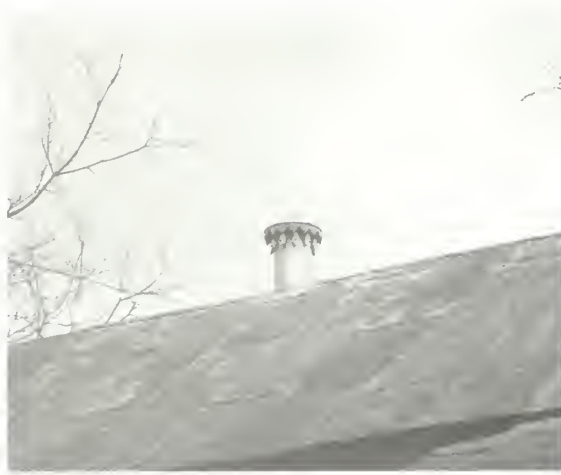
Figure 20 View of south shed of roof with original ventilator (c. 1900). (NPS-SERO-CRS, 2001)
