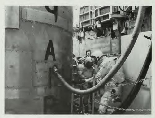
The Titan II ICBM Missile Site 8 (571-7) in Pima County, Arizona, was listed in the National Register in 1992. This view shows a simulated vapor detection check by propellant transfer technicians. (David K. Stumpf, 1992)
