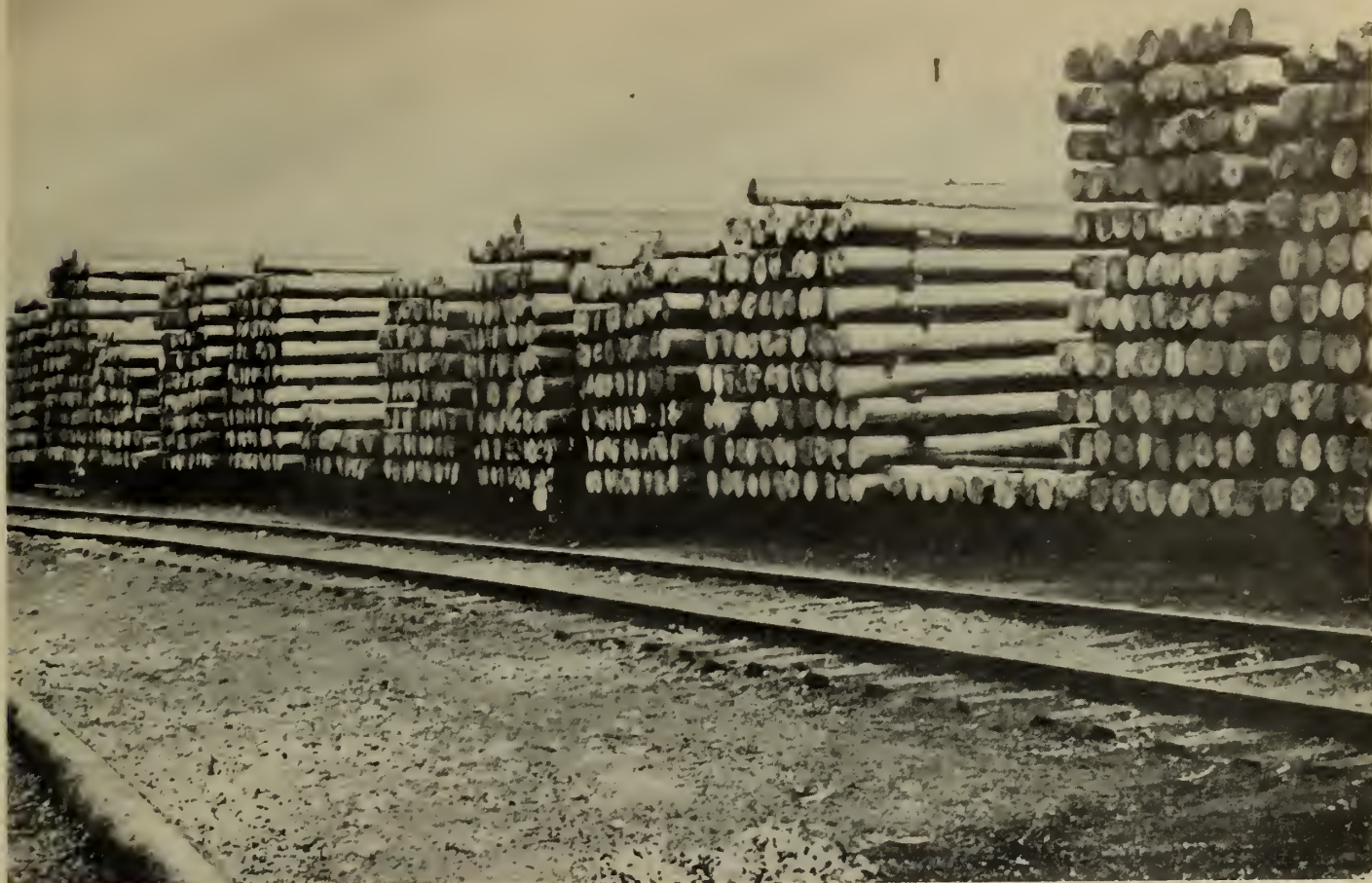
SEASONING - Stocks of Southern Pine poles air-season on the Southern Wood Preserving Company yard before preservative treatment with creosote. The poles are
