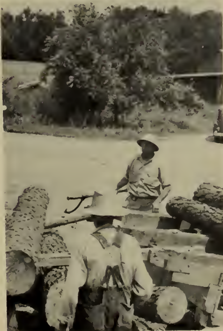
SAWMILL SCENES - W. F. Dew, in photo above, shows Gordon County Ranger J. C. McDearis, left, and Sam Thacker, Management Forester for District 7, right, operation of his water powered sawmill. A turn of the giant wheel, lower left, harnesses the swiftly flowing water to the sawmill machinery. Logs are unloaded at the mill in photo below, center. The mill itself, below, right.
