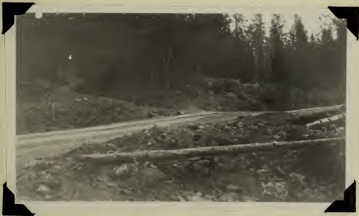
Slide, East Forest, July 25. Repair nearly completed.
