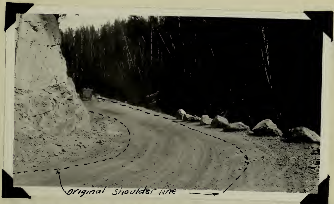
Road Widening at Virginia Cascades.
