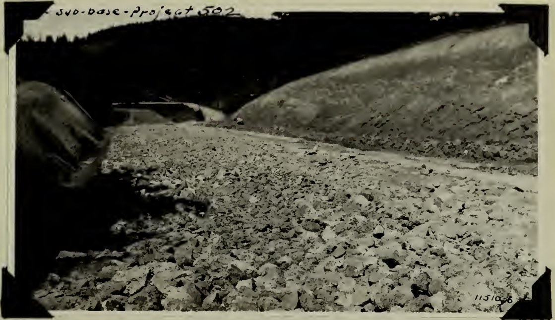
Rock sub-base, Project 502.
