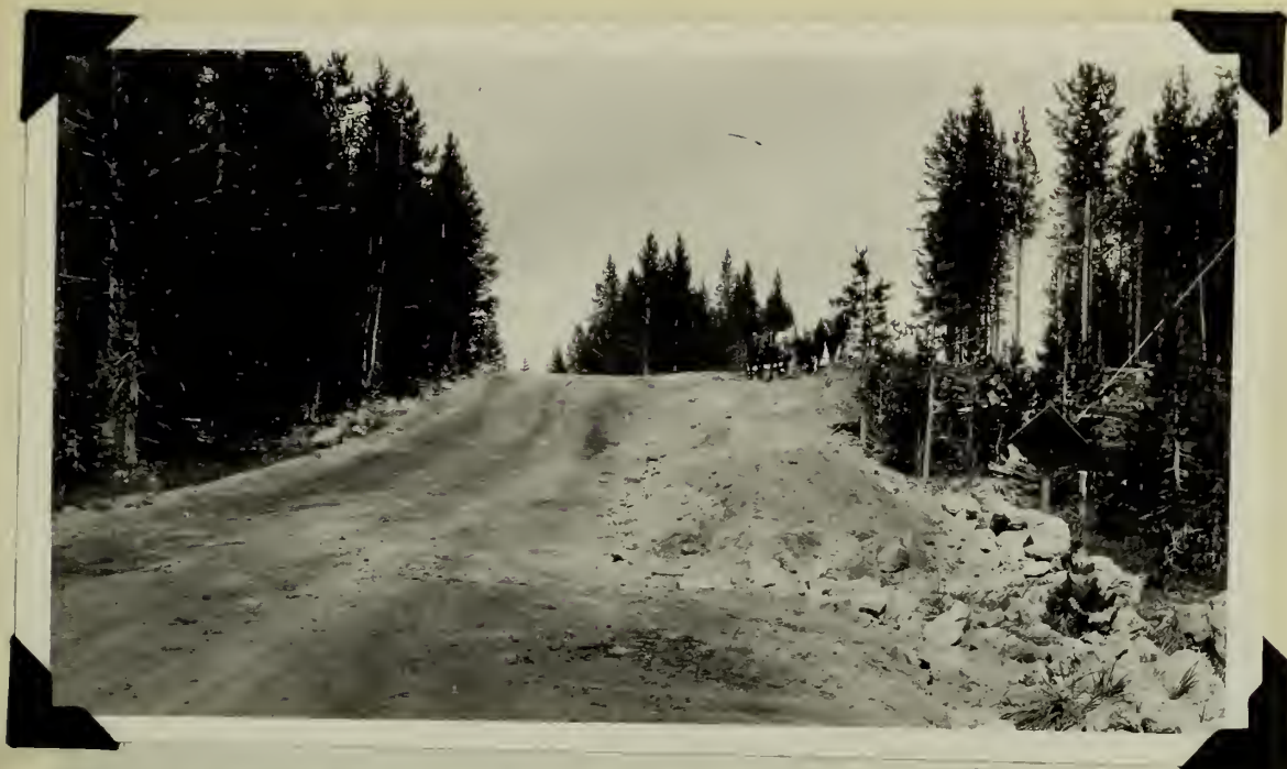
Eliminating dangerous curve, Canyon-Norris Road.
