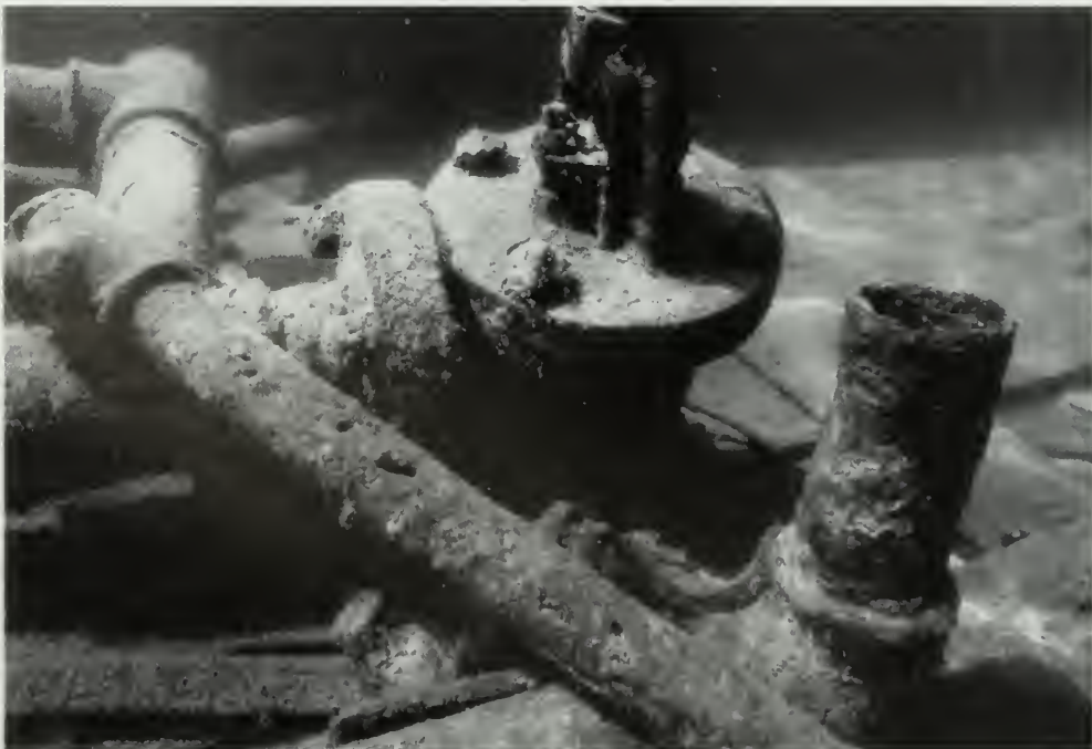
Figure 5.45. Close-up view of globe valve. NPS photo by Brett Seymour.
