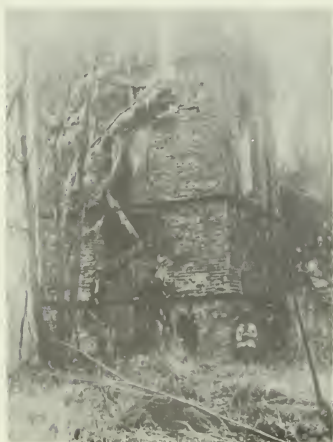
Three sets of steel straps, put in place through the efforts of the National Society of Colonial Dames, held the ruined tower together for about fifty years.
