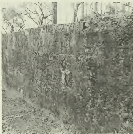
A close look at the fort shows the layers of tabby and the oyster shells that make up the material. Carolinians commonly excavated old Indian shell mounds for the thousands of bushels of shells required in tabby construction.
