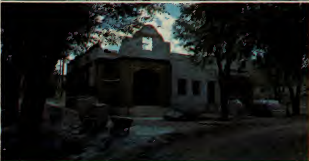
(Right) (1) Tom Romero, Governor of Pojoaque Pueblo, and a citizen at the Pueblo Plaza where Indians operate or lease land for businesses. (2) View of Tesuque Pueblo bridge construction. (3) Reconstruction at Tao Pueblo. (4) BIA project—school under construction, Tesuque Pueblo.
