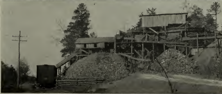
BARITE — This mineral is used in paints and other products to give body or base. Above—Excavating barite ore. Below—Barite washing plant.
