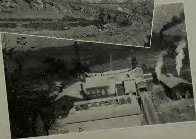
CEMENT —One of the raw materials used in the manufacture of Portland cement is limestone. Top—Soft limestone being scooped up by a steam shovel in Bleckley County. Next below—A cement factory near Perry. Next below—Hard limestone quarry near Rockmart. Bottom—Portland cement plant at Rockmart.
