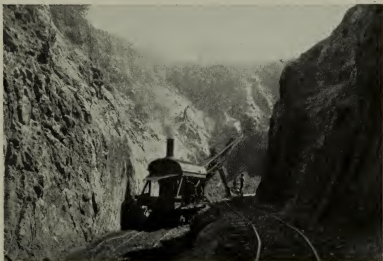
IRON ORE— Brown iron ore mine in Bartow County with steam shovel digging ore from the earth.
