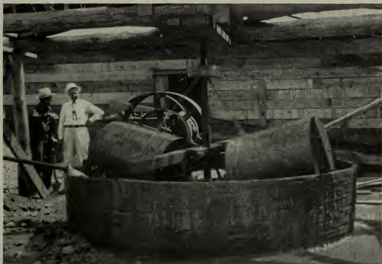
Plant in which three products are recovered, graphite, kyanite, and mica ore. The round mullers grind the stone containing the minerals.
