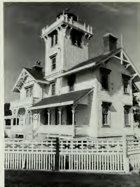
The Point Fermin Lighthouse was the first substantial aid to navigation established at San Pedro and Los Angeles Harbor. Built in 1874, the structure combined the light tower with a residence for the keeper. The Victorian-style station has wooden board and batten siding. Comparing the current condition of the light with the photograph taken in 1917 demonstrates the historic integrity of this lighthouse. (James P. Delgado, National Park Service)
