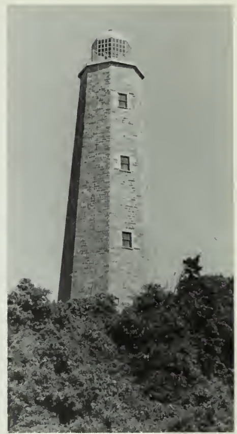
The First Cape Henry Lighthouse sits on the Chesapeake Bay in Virginia Beach, Virginia. Constructed in 1792, it was the first lighthouse to be erected by the Federal government. The 90-foot, sandstone octagonal tower lined with brick was in constant use until 1881. (National Park Service)
