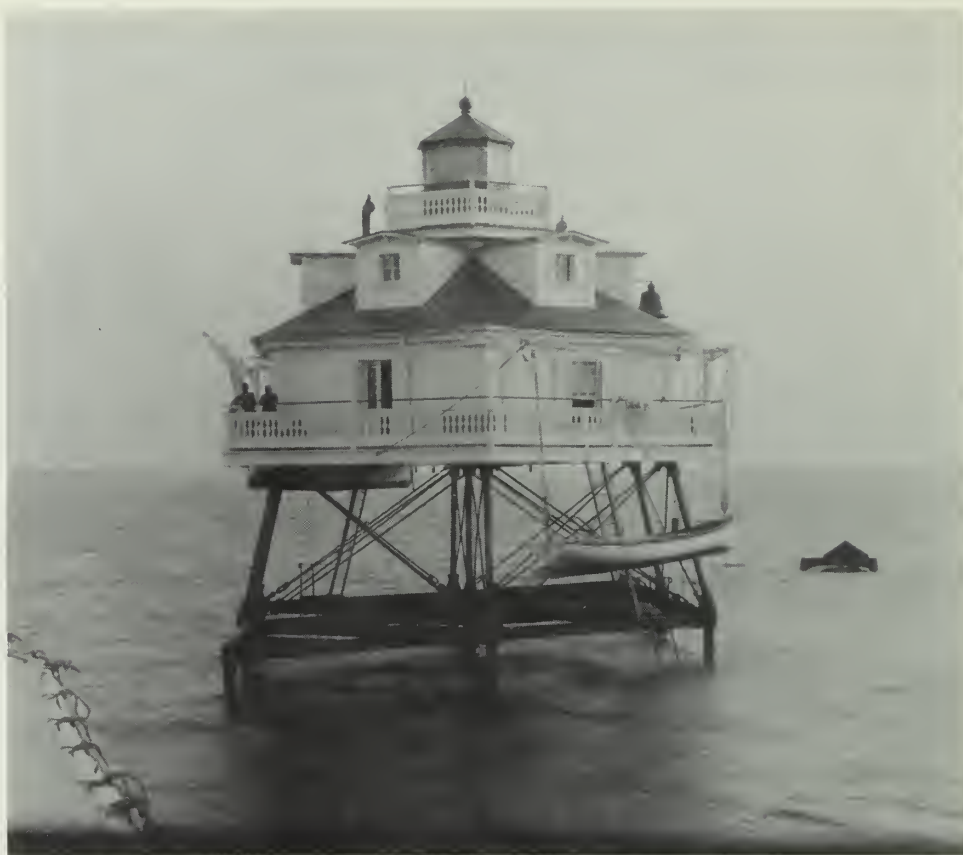
Thomas Point Shoals Light Station, standing in Maryland's Chesapeake Bay, is a hexagonal screwpile, offshore light. Screwpile refers to the nine metal pilings, tipped with two blades arranged in screw fashion, which support the structure. This method of anchoring an aid to navigation was most appropriate for the sandy, muddy bottom of the bay. In this historic photograph, taken in 1885, ten years after the completion of the light, its roof is topped with dormers and a steel octagonal cupola containing the light. (U.S. Coast Guard)
