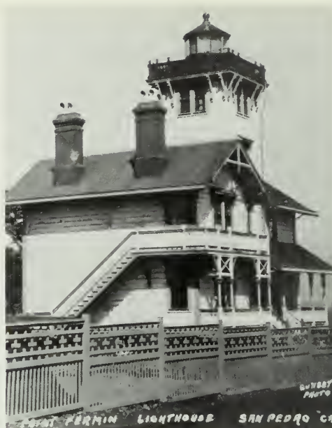
The Point Fermin Lighthouse was the first substantial aid to navigation established at San Pedro and Los Angeles Harbor. Built in 1874, the structure combined the light tower with a residence for the keeper. The Victorian-style station has wooden board and batten siding. Comparing the current condition of the light with the photograph taken in 1917 demonstrates the historic integrity of this lighthouse. (James P. Delgado, National Park Service)
