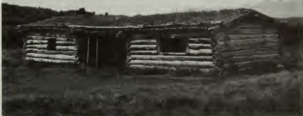
The Cunningham cabin was a typical Jackson Hole homestead. The “dogtrot-style” log cabin has a sod roof. National Park Service
