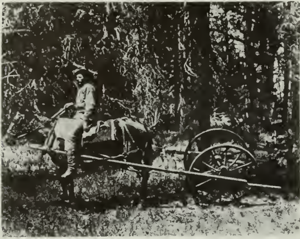
This odometer was used in one of the Hayden Surveys of Yellowstone. The Reynolds Survey of 1860 used a similar odometer in Jackson Hole, until the wheels were lost in a river crossing. U.S. Geological Survey, William Henry Jackson #1290
