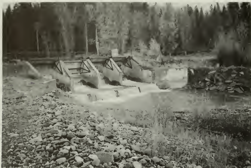
Diversion dams served several farms and ranches, and were usually operated by a cooperating association. This dam, typical of many in Jackson Hole, is on Spread Creek. Grand Teton National Park
