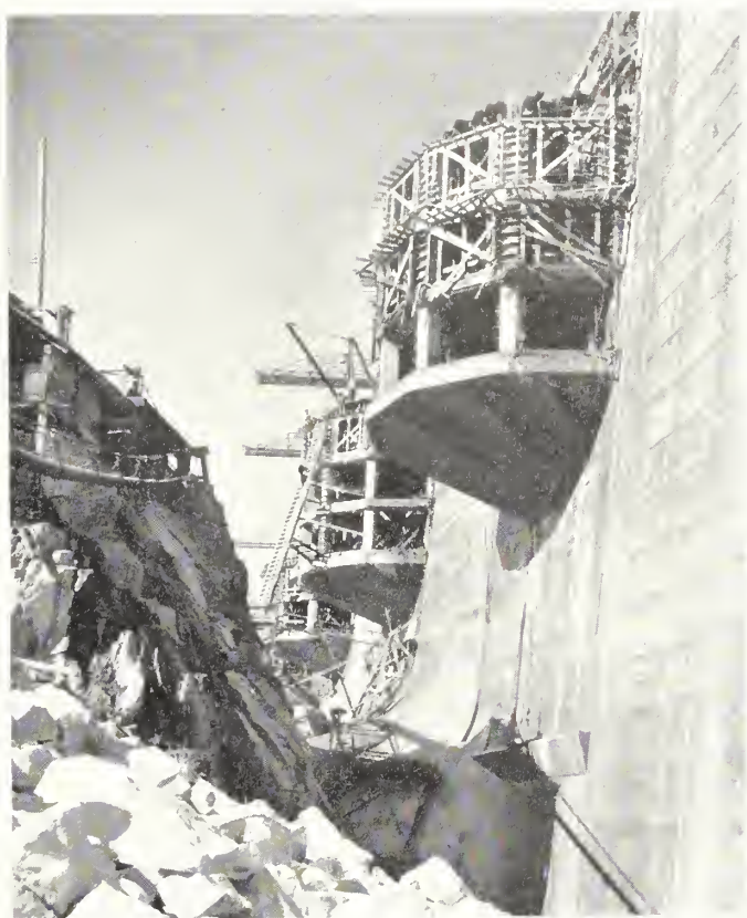
Ground view of trashracks of outlet works on blocks 59, 61, and 63 (in foreground).
