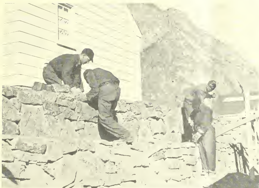
C. C. C. ENROLLEES BUILDING GRANITE RETAINING WALLS IN TOWN OF COULEE DAM—CAMP BR 48, COLUMBIA BASIN PROJECT, WASHINGTON
