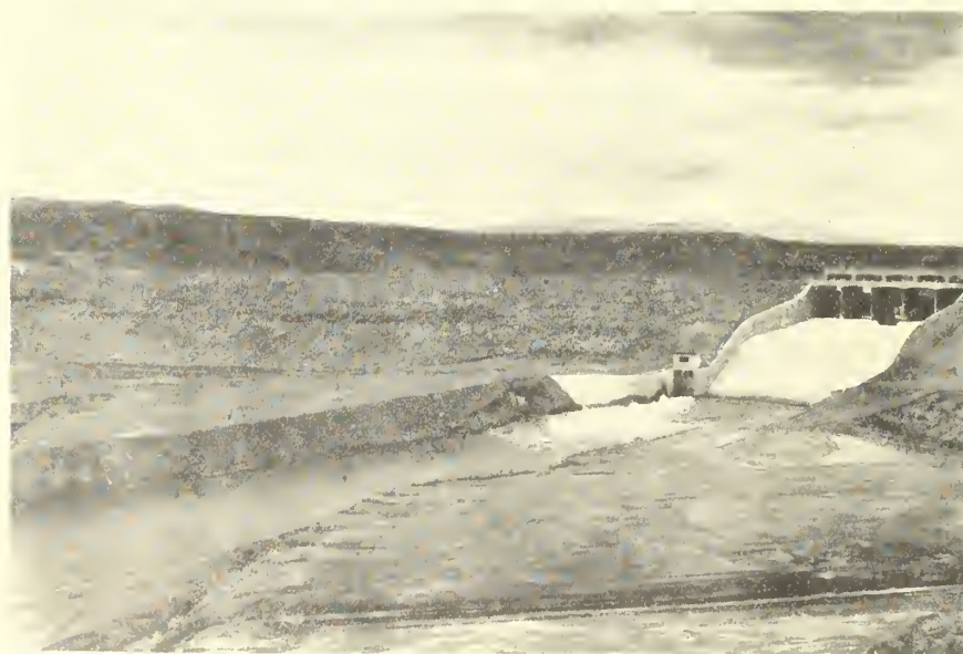
VIEW FROM EAST SIDE, 1,500 FEET BELOW RYE PATCH DAM, LOOKING UPSTREAM AND SHOWING SPILLWAY GATE STRUCTURE, CONTROL HOUSE, AND DOWNSTREAM FACE. OUTLET WORKS DISCHARGING 465 C. F. S.
