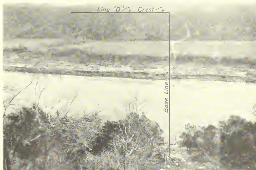
LOOKING ACROSS THE COLORADO RIVER, ALONG THE BASELINE OF MARSHALL FORD DAM. THE BLACK LINE ANGLING TO THE LEFT AND TERMINATING AT THE OBSERVATION TOWER MARKS THE PROPOSED EARTH AND ROCKFILL DIKE SECTION. VIEW TAKEN PREVIOUS TO ANY CLEARING OF GROUND.
