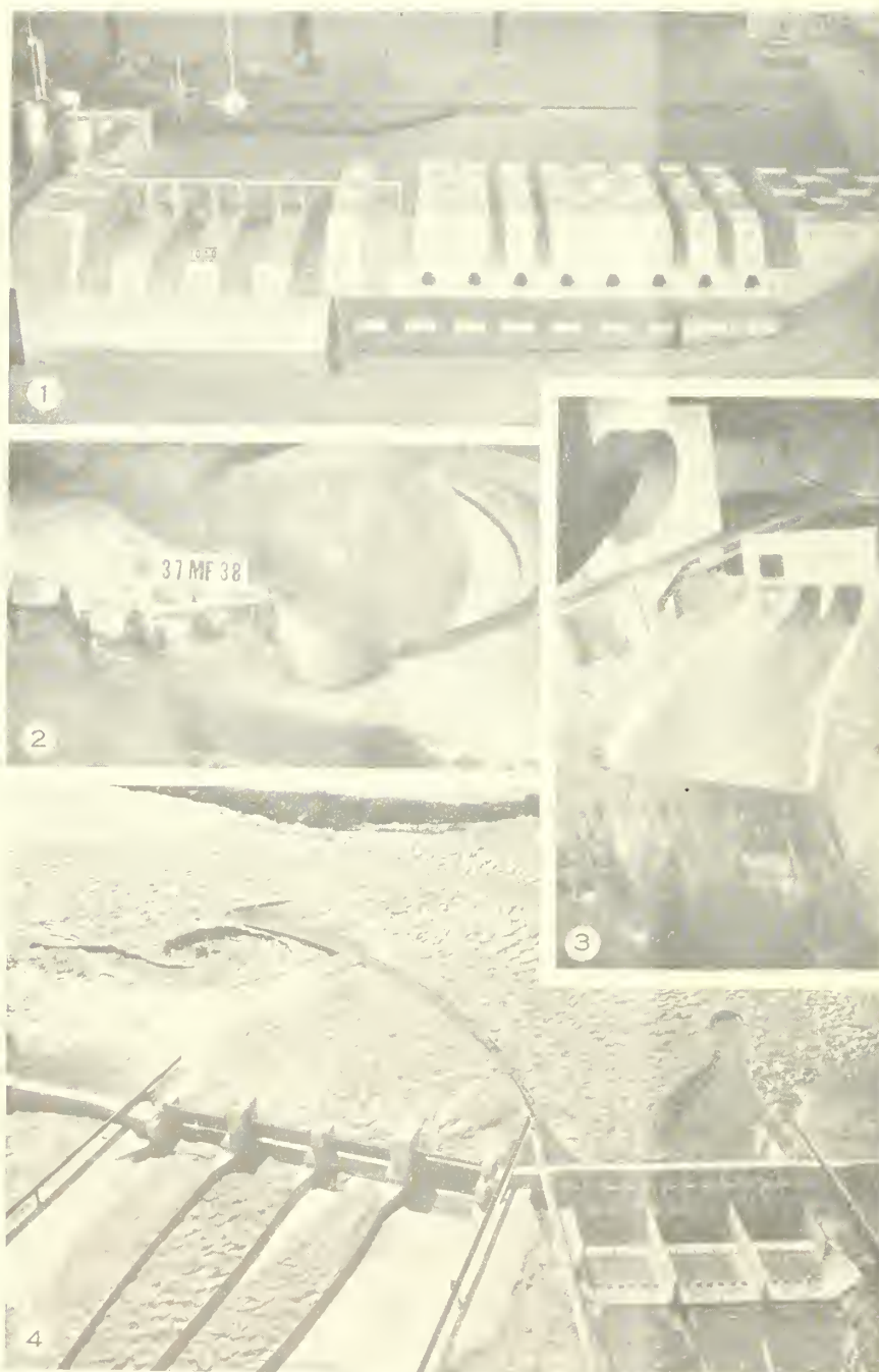
1, GRAND COULEE CONSTRUCTION MODEL; 2, AN ABANDONED DESIGN FOR THE MORMON FLAT SPILLWAY; 3, THE CURVED AND SUPERELEVATED BARTLETT SPILLWAY; 4, MODEL OF ALL-AMERICAN CANAL HEADWORKS.
