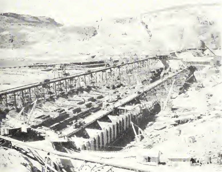
View over the east power-house and spillway sections showing construction work inside the cross-river cofferdams.
