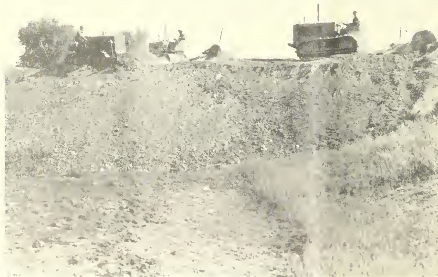
C. C. C. ENROLLEES OPERATING TRACTORS AND TUMBLEBUGS CONSTRUCTING SMALL EARTHFILL DAM TO STORE DRAINAGE WATER CAMP BR-2, BELLE FOURCHE PROJECT, SOUTH DAKOTA
