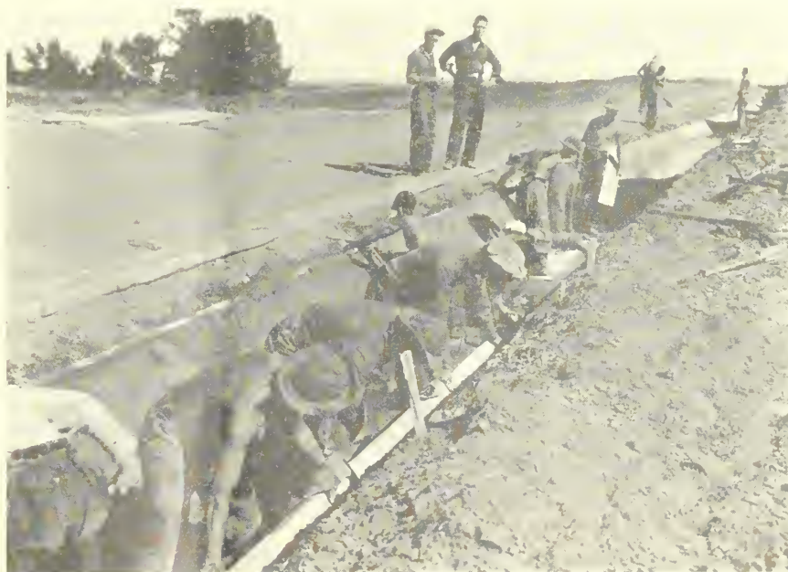
C. C. C. ENROLLEES LEARNING CONCRETE WORK ON LATERAL LINING—CAMP BR-53, NORTH PLATTE PROJECT, NEBRASKA
