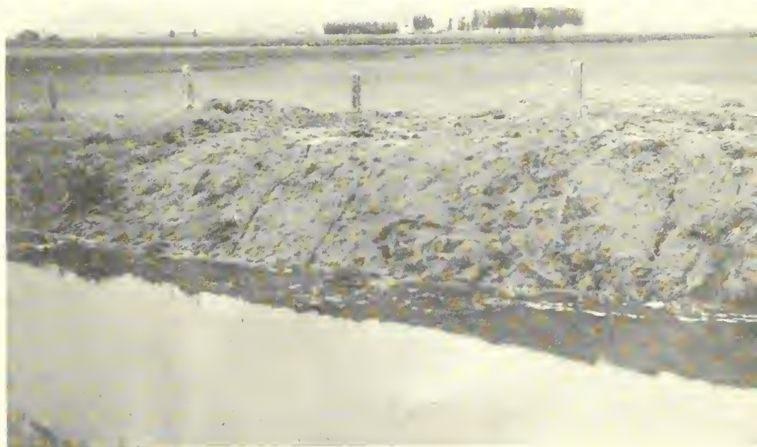
UPPER: BREAK IN CANAL BANK SHOWING FLOODED FARM LANDS, KLAMATH PROJECT, OREGON-CALIFORNIA.
