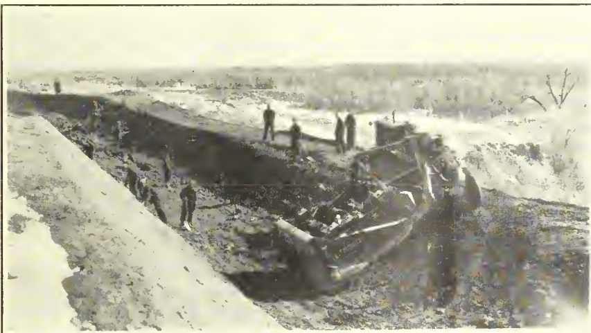
EXCAVATION OF DUCHESNE FEEDER CANAL WITH PNEUMATIC-TIRED SCRAPER. CCC ENROLLEES REMOVING ROCK AND TRIMMING SLOPES.
