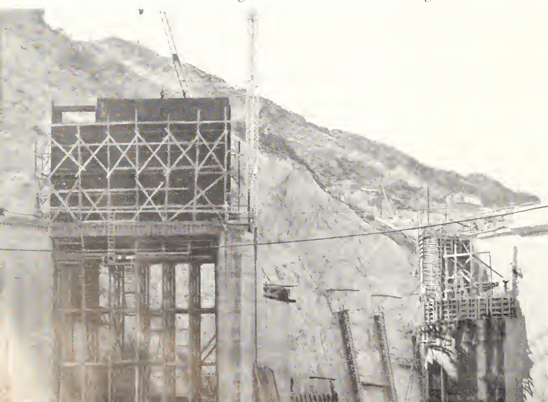
Mormon Flat spillway, Salt River Project, Arizona, showing erection of left gate. Method of trimming channel walls shown in background.
