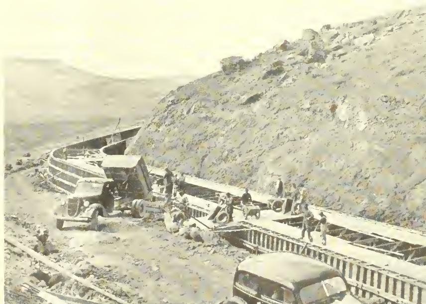
BOISE-PAYETTE DIVISION, BOISE PROJECT, IDAHO. WORKMEN PLACING CONCRETE WALLS OF BENCH FLUME.
