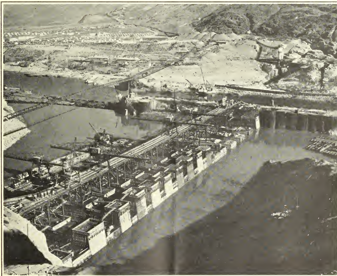
THE COLUMBIA RIVER BEING SLOWLY FORCED FROM ITS ANCIENT COURSE AS CONSTRUCTION OF GRAND COULEE DAM PROCEEDS. A COFFERDAM IS BEING CONSTRUCTED ACROSS THE RIVER
