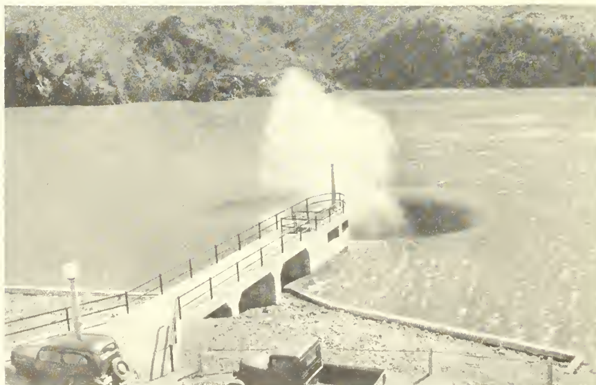
OWYHEE DAM SPILLWAY, OWYHEE PROJECT, OREGON-IDAHO. SPRAY RISING WITH UPDRAFT OF AIR.
