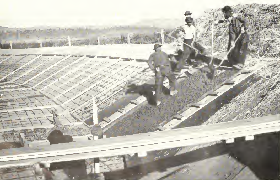
CCC ENROLLEES LINING A CANAL ON THE KLAMATH PROJECT, OREGON-CALIFORNIA.
