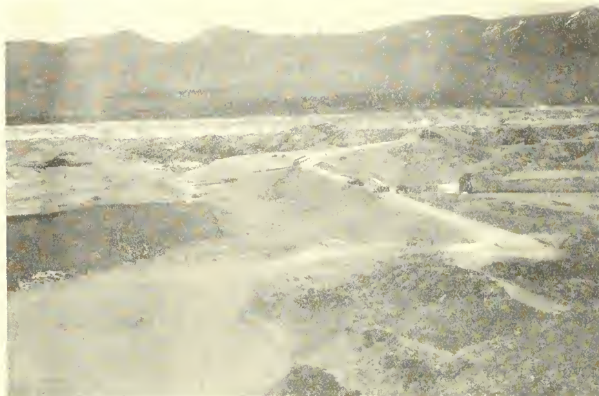
RYE PATCH DAM, HUMBOLDT PROJECT, NEVADA, COMPLETED IN THE SPRING OF 1936. OF EARTHFILL CONSTRUCTION, IT IS 75 FEET HIGH. THE RESERVOIR CAPACITY IS 80,000 AC. FT.
