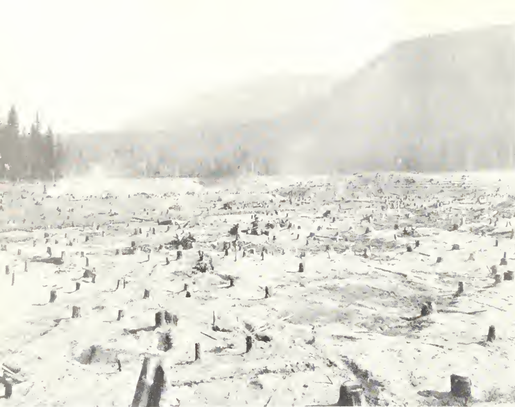
Clear Creek Reservoir area thoroughly cleared of dead timber by C. C. C., Yakima Project, Washington.
