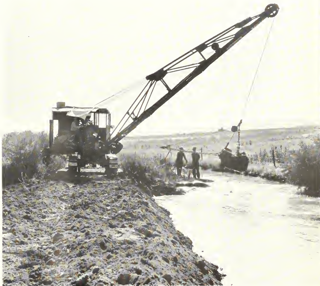
CCC FORCES REMOVING SILT FROM A HALF-FILLED CANAL ON THE SHOSHONE PROJECT, WYOMING.
