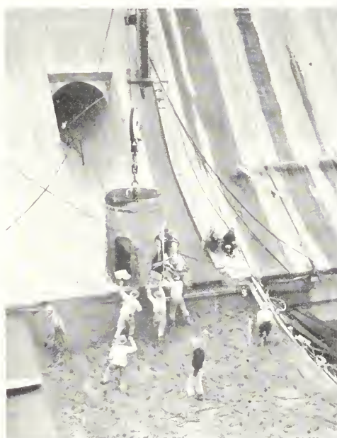
Concrete placing—final lift in block 57-1.
