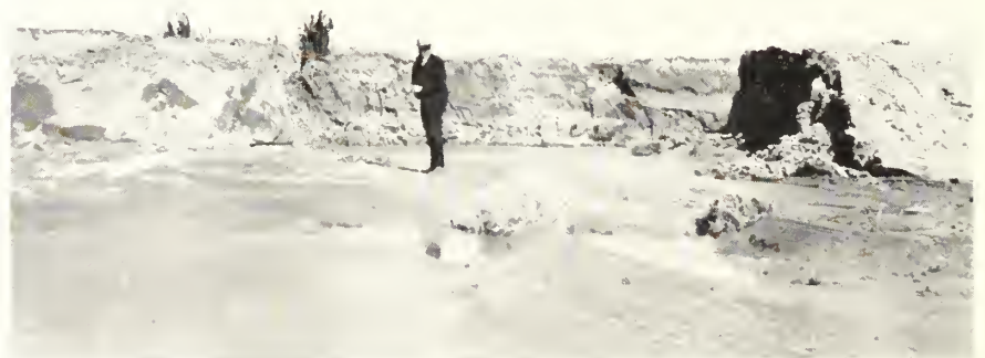
EXPENSIVE CANAL BREAKS ARE FREQUENTLY CAUSED BY BURROWINGS OF GOPHERS.
