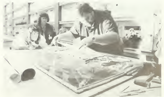
Figure 14. The instructor removes one of six etched plates from a ca. 1905 Tiffany window in order to clean the interspaces and provide a rare educational opportunity at a restoration workshop. Cypress Lawn Memorial Park, Colma, California. Photo: Neal A. Vogel.
