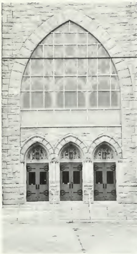
Figure 20. (a) The aluminum frame grid used for protective glazing totally disregards the original tracery of this Neo-Gothic church. The grid mars the appearance of the window inside and out. It also impairs the overall historic character of the building. (b) Protective glazing in this instance preserves both the appearance of the window and its contribution to the building. The latter building is the Cathedral Basilica of the Assumption (St. Mary's Cathedral), Covington, Kentucky (1895-1910). The window, 67' x 24' (20.4m x 7.3m), is among the largest stained glass windows in the United States. Photos: Neal A. Vogel.
