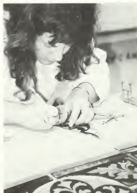
Figure 15. New stencils are used to produce matching replacement glass for repetitive stenciled patterns in a ca. 1870 window. Photo: Neal A. Vogel.
