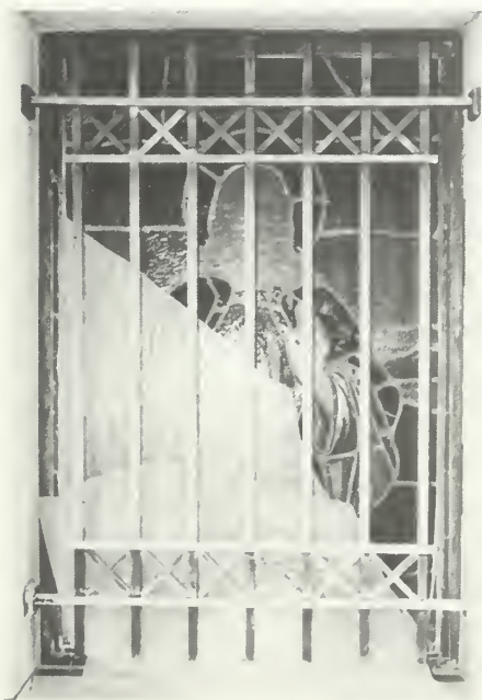
Figure 19. Stained glass in mausoleums requires protective glazing since vandalism is frequent in cemeteries. This plate glass intentionally softened the light transmitted through the window. This feature should be reproduced in the replacement glazing. It may be possible to repair the plate glass and install another, stronger (clear) layer on the outside. Photo: Neal A. Vogel.
