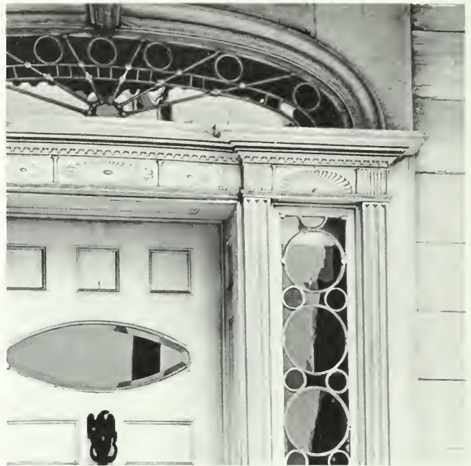
Figure 3. The entrance to the Morris-Jumel Mansion, New York City, is one of the earliest surviving installations of leaded glass in the country. It features a leaded fanlight and sidelights of large clear roundels and small bulls-eyes of red and orange flashed glass from ca. 1810. Photo: The American Institute of Architects Library and Archives, Washington, D.C.
