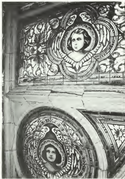
Figure 12. These stained glass angels appear concerned over the cracked terra cotta frames of the rose window they grace. Photo: Neal A. Vogel.
