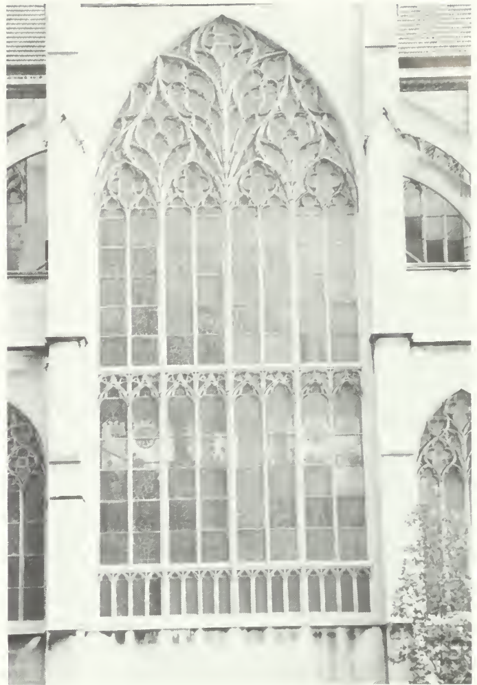
Figure 20. (a) The aluminum frame grid used for protective glazing totally disregards the original tracery of this Neo-Gothic church. The grid mars the appearance of the window inside and out. It also impairs the overall historic character of the building. (b) Protective glazing in this instance preserves both the appearance of the window and its contribution to the building. The latter building is the Cathedral Basilica of the Assumption (St. Mary's Cathedral), Covington, Kentucky (1895-1910). The window, 67' x 24' (20.4m x 7.3m), is among the largest stained glass windows in the United States. Photos: Neal A. Vogel.
