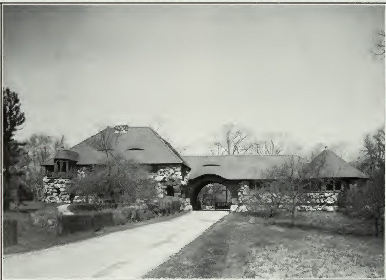
The Ames Gate Lodge, located in North Easton, Massachusetts, was designed in 1880-81 by architect H.H. Richardson during his period of collaboration with landscape architect Frederick Law Olmsted. Constructed of massive, weathered boulders, the lodge contains a gently sloped and curving roof and is bisected by a rusticated arched entrance to the Ames Family estate. Richardson's use of natural materials, the bold arch, and forms to harmonize with the surrounding landscape made the Ames Gate Lodge a model of rustic, Shingle-style architecture that would be adopted by park designers for several generations. (William Pierson)
