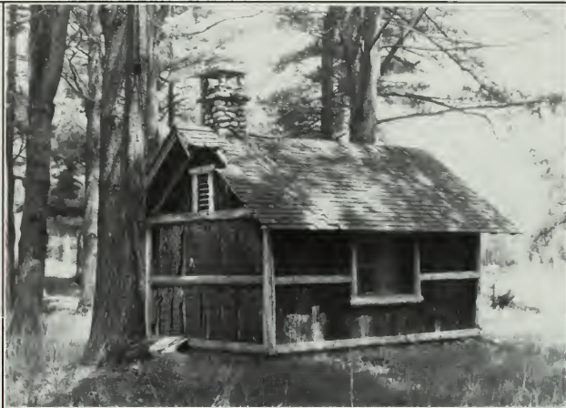
The concern for harmonizing with nature extended to the design of the many small structures associated with the Adirondack camps. The pump house at Camp Uncas was constructed of exterior pole framing made of native cedar logs and sheathing of spruce bark. A cobblestone chimney projects through the shingled gable roof. (New York State Office of Parks, Recreation, and Historic Preservation)
