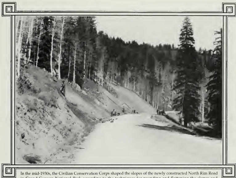
In the mid-1930s, the Civilian Conservation Corps shaped the slopes of the newly constructed North Rim Road in Grand Canyon National Park according to the techniques for rounding and flattening the slopes and blending the banks into the surrounding forest. This work greatly reduced soil erosion along new roads and created the illusion that nature had never been disturbed. (National Archives, Record Group 79)
