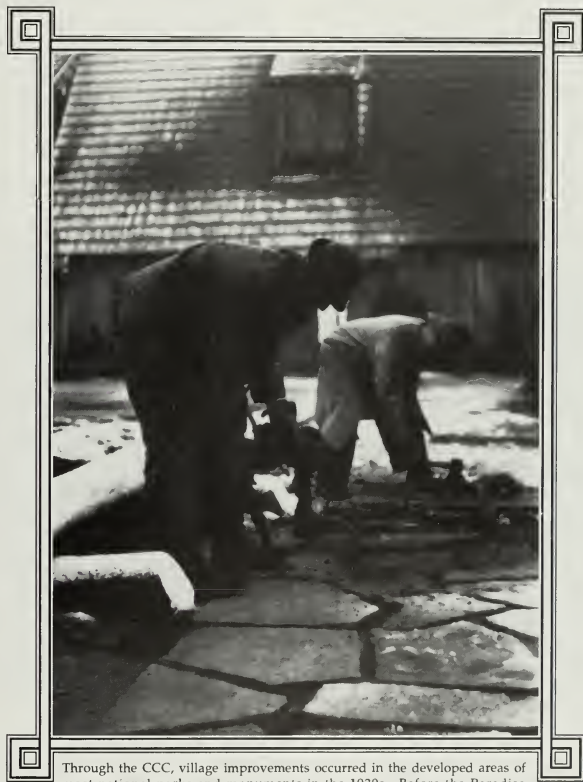
Through the CCC, village improvements occurred in the developed areas of most national parks and monuments in the 1930s. Before the Paradise Community Building in Mount Rainier National Park, CCC enrollees laid a naturalistic, flagstone walk with sod joints. (National Park Service Historic Photography Collection)
