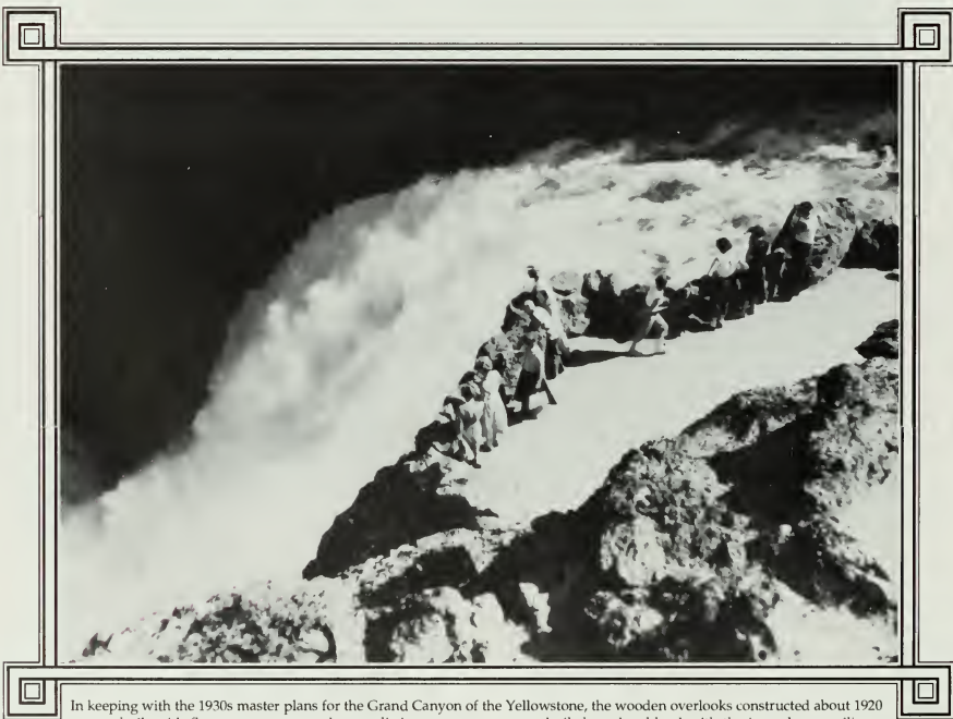
In keeping with the 1930s master plans for the Grand Canyon of the Yellowstone, the wooden overlooks constructed about 1920 were rebuilt with flagstone terraces and naturalistic stonemasonry guardrail shaped to blend with the irregular, curvilinear contours of the natural cliffs. Viewed from a distance the manmade walls were indistinguishable from the walls of the natural gorge. (National Park Service Historic Photography Collection)
