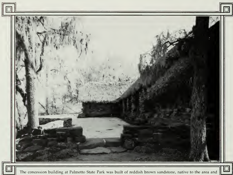
The concession building at Palmetto State Park was built of reddish brown sandstone, native to the area and reflected Herb Maier's principles of rockwork. Among the special features were the raised terrace with its stonemasonry parapet, the battered stone walls that flared as much as ten feet at the corners of the building, and the massive boulder chimney of stones carefully removed from nature and reassembled at the construction site to appear naturalistic. The camp superintendent wrote, "We are matching rocks in such a manner that they appear to grow out of the ground rather than producing a step effect. To protect the growth of lichen found on the rocks in the flare we are leaving the flare above the ground to be built last. . . . I think it worthwhile to protect the beautiful growth which would otherwise be destroyed." (National Archives, Record Group 79)
