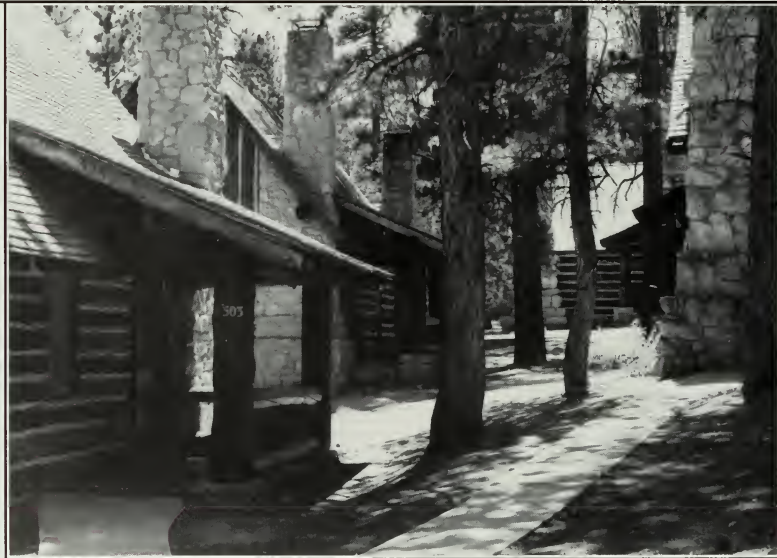
Following the concept he developed at Zion National Park, architect Gilbert Stanley Underwood designed 15 deluxe cabins and a small centrally located pavilion for the concessionaire at Bryce Canyon National Park. Located in a pine grove and reached by meandering paths, the cabins were built to harmonize with the natural setting. They had log slab siding, rubble masonry foundations and chimneys of locally quarried stone, and porches of peeled log railings and posts. (Laura Soulliere Harrison)
