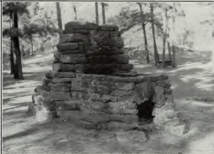
Naturalistic stonemasonry fireplaces were built at Bastrop State Park in Texas. The CCC in state and national parks in the 1930s fashioned utilitarian objects such as fireplaces and water fountains into hand-crafted, naturalistic rockwork that blended with the natural setting. (National Archives, Record Group 79)
