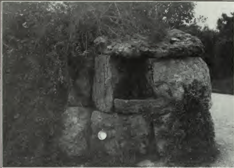
Typical of the sturdy park structures at Franklin Park, this rustic water fountain was made from slabs of local puddingstone laid up in monolithic fashion to imitate the natural rock outcroppings that abounded throughout the park. (National Park Service, Frederick Law Olmsted National Historic Site)
