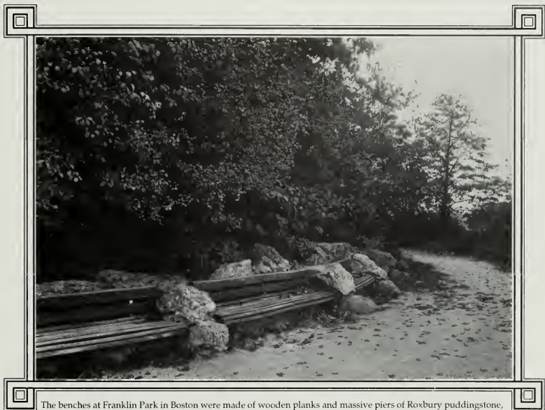
The benches at Franklin Park in Boston were made of wooden planks and massive piers of Roxbury puddingstone, a local conglomerate. They were designed to follow the flowing curves of the drive and to blend the manmade construction with the surrounding woodlands and rock outcrops. (National Park Service, Frederick Law Olmsted National Historic Site).
