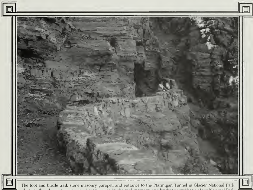
The foot and bridle trail, stone masonry parapet, and entrance to the Ptarmigan Tunnel in Glacier National Park illustrate the advances made in trail construction by the civil engineers and landscape architects of the National Park Service in the late 1920s. The tunnel was blasted through 180 feet of solid limestone and had enough clearance to carry a person on horseback. (National Park Service Historic Photography Collection)
