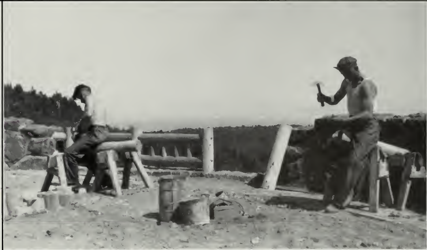
CCC enrollees at Gooseberry State Park, Minnesota, in June 1936 used hand-tools to peel and assemble native logs into naturalistic guardrail for the parking concourse and overlook constructed near the Gooseberry River on U.S. Highway 61, which passed through the park. The retaining wall for the concourse alone required about 646 cubic yards of native granite and contained stones weighing as much as three tons. (National Archives, Record Group 79)
