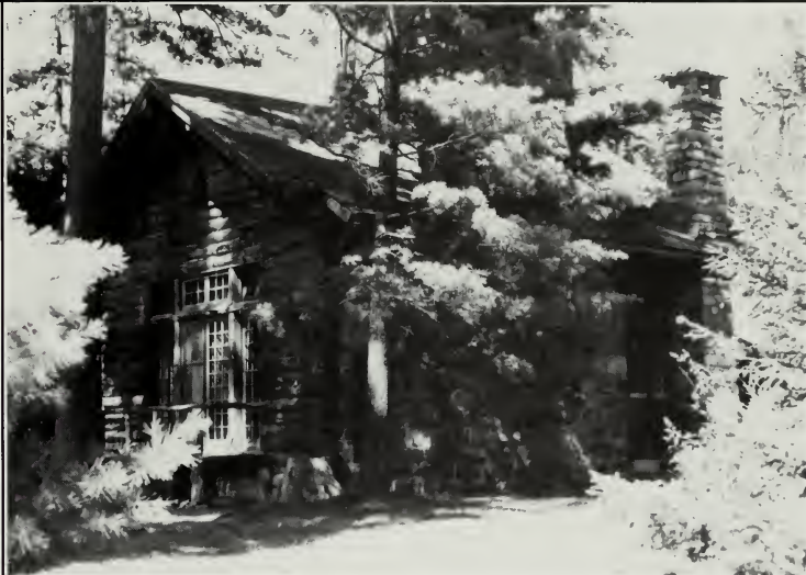
The Dining Hall at Camp Uncas, the Adirondack camp built for financier J. P. Morgan between 1893 and 1895, illustrates characteristics typical of the Adirondack style. The hall was carefully sited above Mohegan Lake to afford views, to disturb as few trees as possible, and to blend with the natural setting. It features a stone rubble foundation, spruce log walls, and a gable roof with overhangs and exposed purlins. A massive native stone chimney projects through the roof. (New York State Office of Parks, Recreation, and Historic Preservation)
