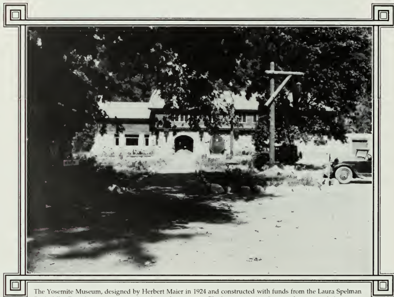
The Yosemite Museum, designed by Herbert Maier in 1924 and constructed with funds from the Laura Spelman Rockefeller Foundation, set a precedent for park museums. The lower story is a fire-proof masonry-clad concrete vault while the upper story reflects the redwood shingle siding and exposed log framing that Myron Hunt had used in his design for the nearby administration building. Photographed about 1928, this view of the entrance shows the boulder-lined paths, log lampposts, and boulder curbs that characterized the village plaza in the late 1920s. ((National Archives, Record Group 79))
