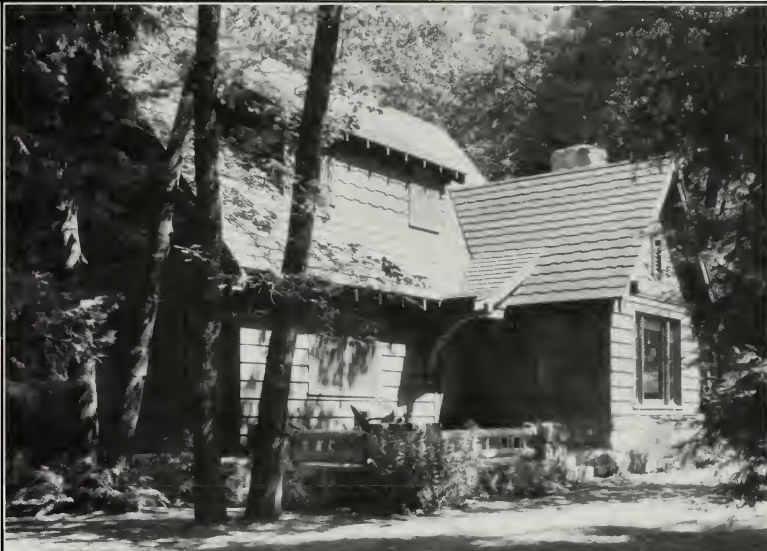
During the 1930s, funding from the Public Works Administration made possible the construction of much-needed housing for park employees in Yosemite National Park. Single-family residences took the form of Craftsman-style bungalows and had redwood siding, wooden shingles, stone foundations, an entrance porch with peeled log railings, and a stone chimney. Each house had a living room, dining room, kitchen, 3 bedrooms, and 2 baths. The CCC removed dangerous limbs from the surrounding oaks and planted ferns, azaleas, and other native plants as part of a program to beautify and naturalize Yosemite Village. (Report on the Building Program from Allotments of the Public Works Administration, 1933-1937)
