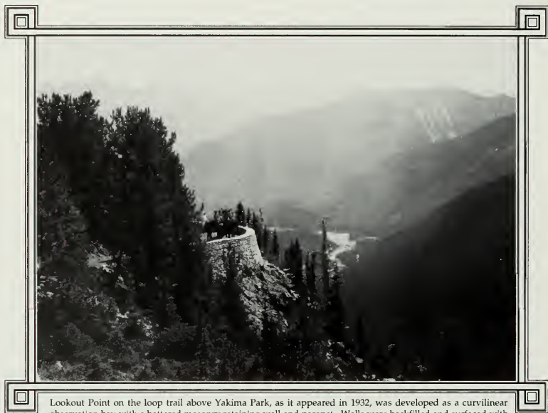
Lookout Point on the loop trail above Yakima Park, as it appeared in 1932, was developed as a curvilinear observation bay with a battered masonry retaining wall and parapet. Walls were backfilled and surfaced with gravel from local rockwork to provide a safe, flat terrace that could accommodate large groups of visitors on foot or horseback. (National Park Service Historic Photography Collection).
