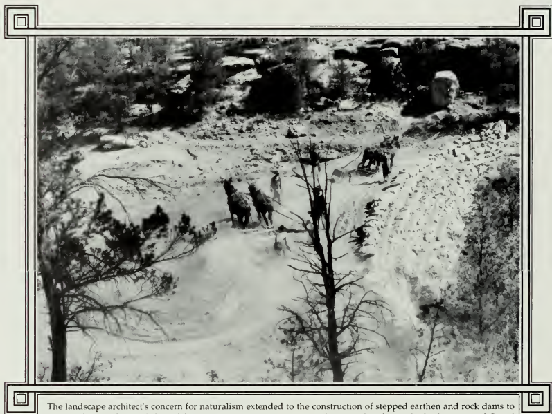
The landscape architect's concern for naturalism extended to the construction of stepped earthen and rock dams to impound water for wildlife and fire suppression. With the help of teams of mules in the backcountry of Grand Canyon National Park, CCC enrollees from the Powell Camp built several dams of dry-laid native rock masonry that were backfilled with earth and blended with the natural surroundings. (National Archives, Record Group 79)
