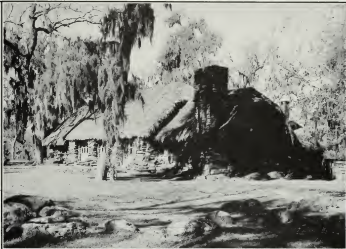
In keeping with the romantic rustic tradition that A. J. Downing had popularized in the nineteenth century and the American Arts and Crafts movement had applauded in the early twentieth century, the roof of the concession building at Palmetto State Park in Texas was thatched with fronds of native palmetto ( Sabal minor ) to contrast with the hanging Spanish moss that hung from the surrounding elm, pecan, and cottonwoods trees. The roof required 32,000 leaves, many of which were gathered outside the park. Since nine leaves alone weighed ten pounds, the roofing turned out to be quite an undertaking. (National Archives, Record Group 79)
