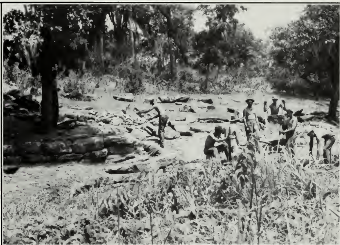
Through a great deal of rockwork and planting of native materials, the CCC at Palmetto State Park in Texas turned this spring into an attractive water garden that blended with the surrounding parkland. Other "landscape naturalization" work in one of the park's swamps included the construction of a new creek channel by forming a series of rock falls and lining the bank with weathered stone "in such a manner as to give the appearance of having been there for years." (National Archives, Record Group 79)
