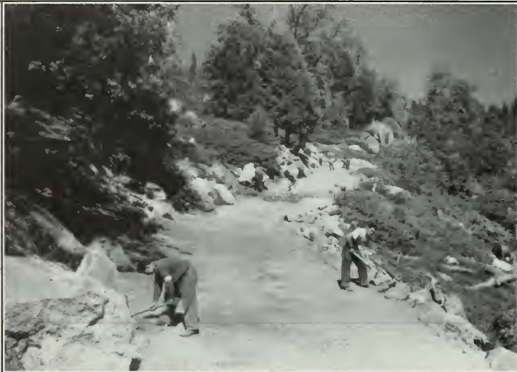
One important activity of the CCC in Yosemite National Park and elsewhere was the construction of truck roads. These were roads built through the national parks for a variety of administrative and fire control purposes. Although visitors seldom used these roads, care was taken in construction to make them inconspicuous, to protect natural features, to avoid erosion, and to blend them into the natural setting using native vegetation and boulders. (National Archives, Record Group 79)
