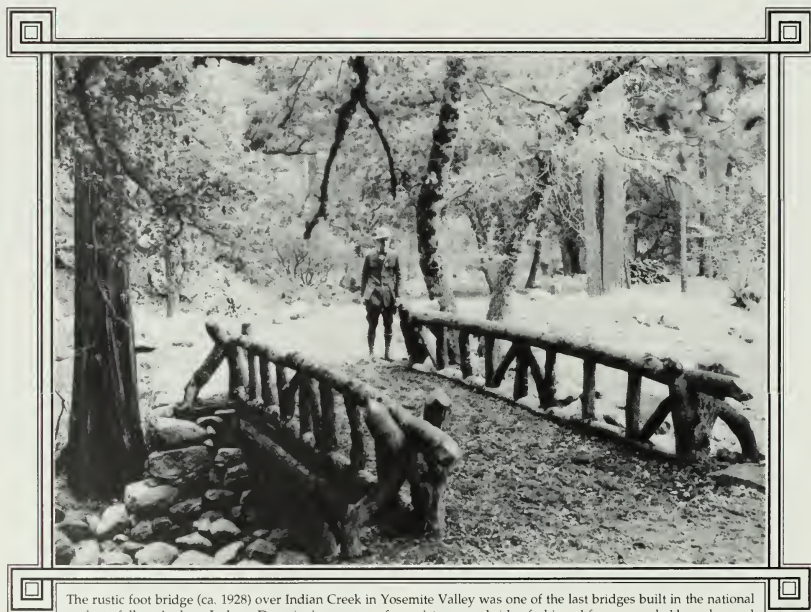
The rustic foot bridge (ca. 1928) over Indian Creek in Yosemite Valley was one of the last bridges built in the national parks to follow Andrew Jackson Downing's prototype for a picturesque bridge fashioned from unpeeled branches and tree trunks. (National Archives, Record Group 79)
