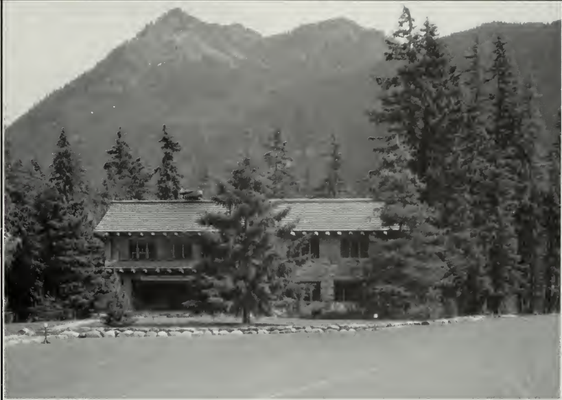
Photographed in 1932, the "naturalized" plaza at Longmire in Mount Rainier National Park reflected the manifold achievements of the National Park Service's Landscape Division on the eve of the New Deal. Completed in 1928 and constructed of massive native boulders and stout logs, the administration building was the focal point of the village. It resulted from a synthesis of rustic design principles, including the use of native materials, pioneer building methods, and elements that stressed irregular lines and horizontality. Native firs, hemlocks, and cedars were left in place or planted around three sides and at the corners of the building. Ferns and other low-growing native plants were planted in the rock-garden by the entry porch and along the foundation. A flagstone walkway and curbing comprised of horizontally-laid, lichen- and moss-covered stream boulders further unified the village setting. The plantings and rockwork represented the beginnings of a program of landscape naturalization intended to erase the scars of construction, to provide village improvements, and to blend manmade structures with a park's natural setting. (National Park Service Historic Photography Collection)
