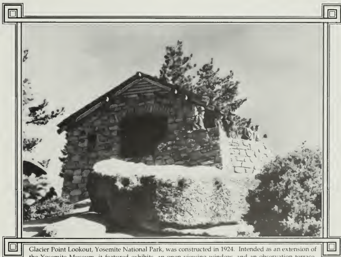
Glacier Point Lookout, Yosemite National Park, was constructed in 1924. Intended as an extension of the Yosemite Museum, it featured exhibits, an open viewing window, and an observation terrace. Made of randomly-laid native stonemasonry, it was one of the first interpretive shelters designed by the National Park Service and established a model for lookouts, nature shrines, and other kinds of interpretive shelters that appeared later in other national parks and in state parks. (National Park Service Historic Photography Collection)
