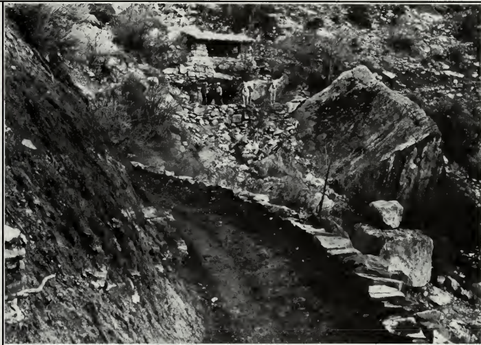
While the Bright Angel Trail in Grand Canyon was rebuilt in the late 1920s to the advanced standards of the National Park Service's Engineering Division, shelters along the trail were constructed by the CCC in the 1930s. Perched above the trail and fashioned from native stone and juniper thatching to blend with the natural setting, the first shelter was located two miles below the canyon rim. It offered visitors traveling on foot or muleback a shady spot to rest, a cool drink of water, and a scenic view. (National Park Service Historic Photography Collection)
