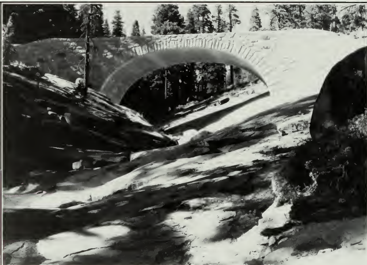
Clover Creek Bridge on the General's Highway, Sequoia National Park, shortly after construction (September 1933) illustrates the simple arch and irregular stone-faced masonry prototype derived from the Scarborough bridges at Franklin Park. The wall and arch rings of native rock were perfectly designed to increase the irregularity and random character of the surface so that the bridge blended into and harmonized with the natural setting, a deeply cut rock creek amidst a towering forest. (National Park Service Historic Photography Collection)
