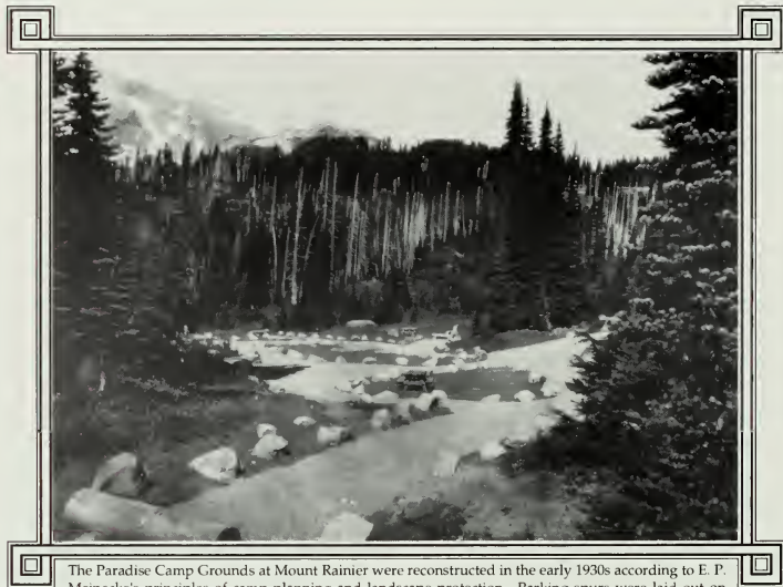
The Paradise Camp Grounds at Mount Rainier were reconstructed in the early 1930s according to E. P. Meinecke's principles of camp planning and landscape protection. Parking spurs were laid out on one-way roads and marked with boulders and log barriers. Each campsite was equipped with a table, fireplace, and tent clearing. (National Archives, Record Group 79)
