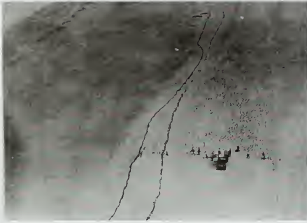
FIGURE 25. A view of workers planting grass to help stabilize dunes created behind sand fences around the Cape Hatteras Lighthouse, from which this photograph was taken. (NPS photograph, late 1930s. CAHA archives)
