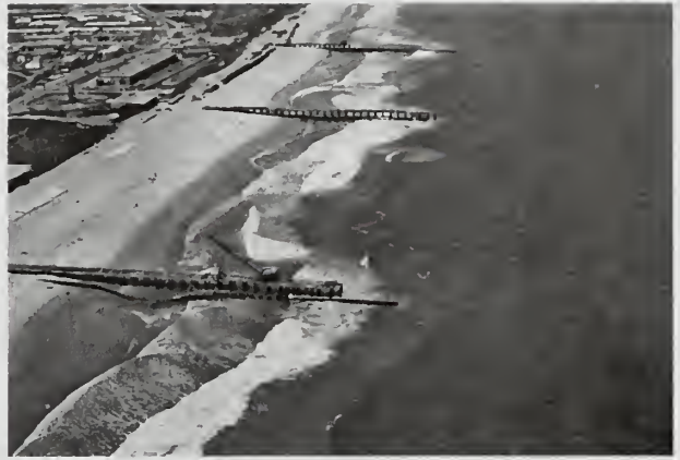
FIGURE 76. In 1968, an effort to check beach erosion near Cape Hatteras, three groins were installed. During construction, the groins began to fail, as is evident in the photograph. (NPS photograph, no date [ca. 1968])
