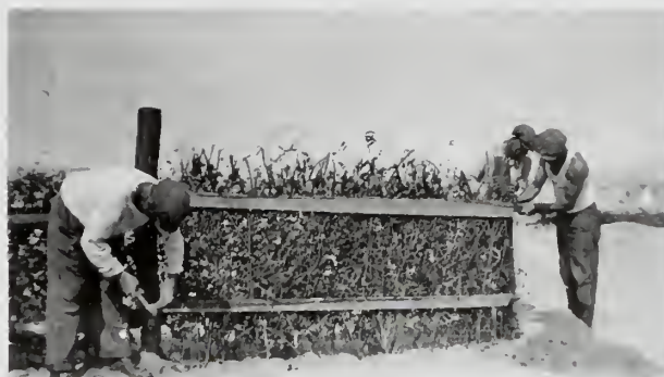
FIGURE 17. Relief workers constructed hundreds of miles of sand fences during the 1930s along the Outer Banks. (NPS photographs from CAHA archives)
