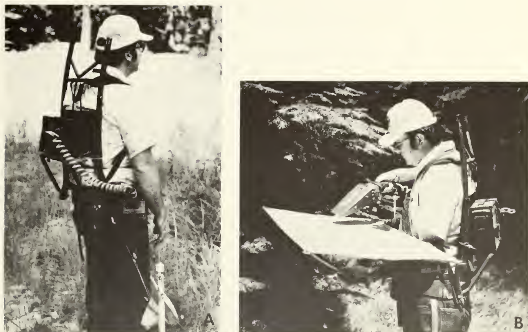
Figure 2.--(A) Pack-frame with mounted battery and side holster for vacuum; (B) collecting arthropods from beating cloth.
