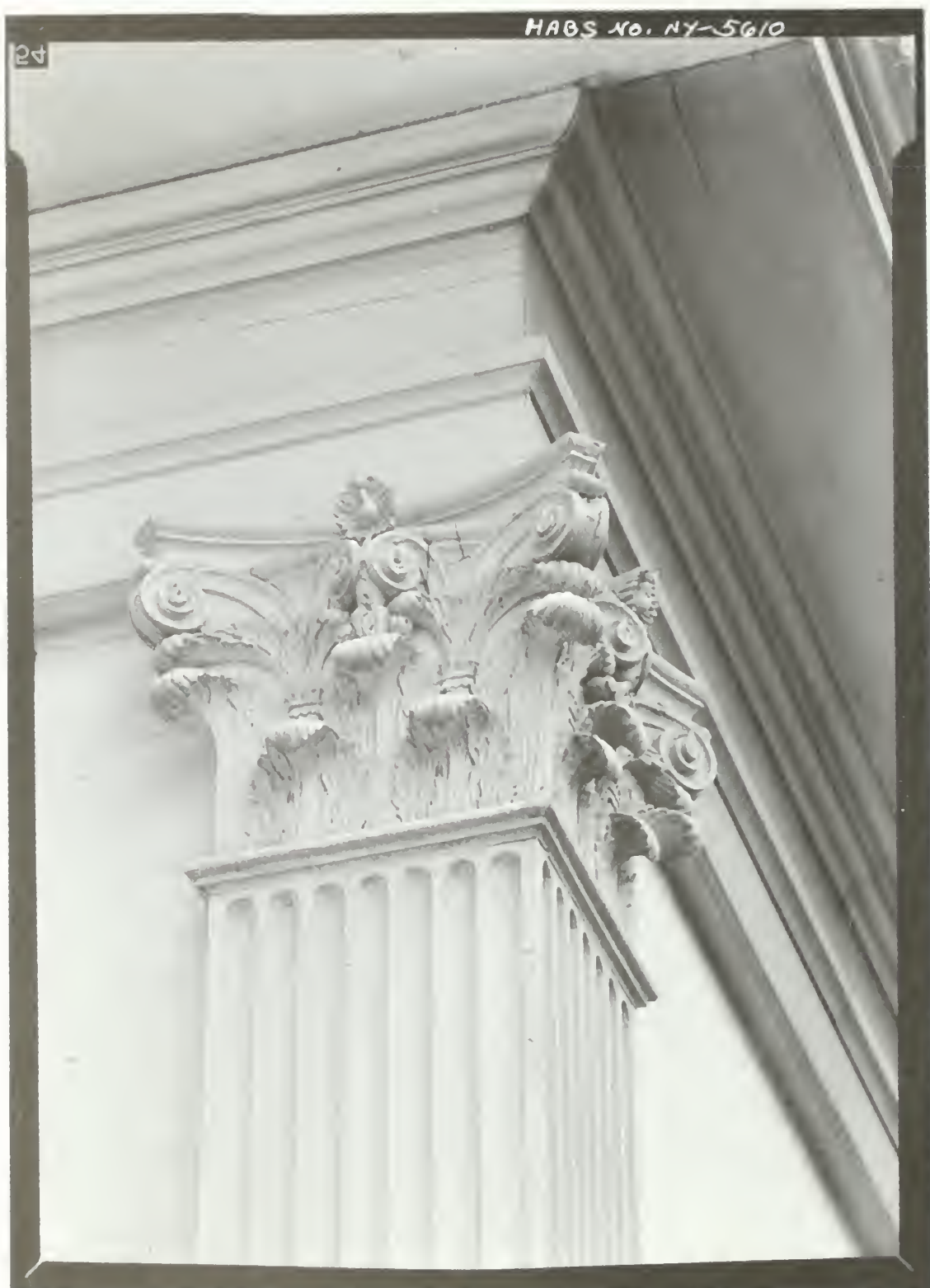
Figure 1.36. Pilaster capital detail, circa 1965.
