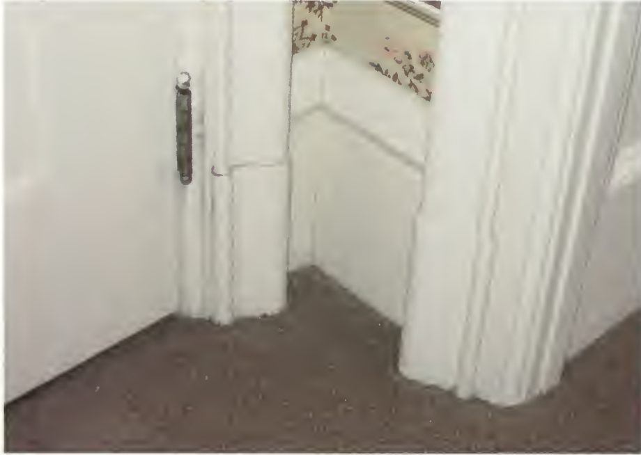
Figure 2.32. Room 102 (Front Hall), ogee casing and plinth blocks.
