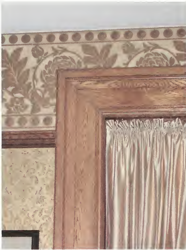
Figure 2.34. Room 104 (Library), molded oak casing.
