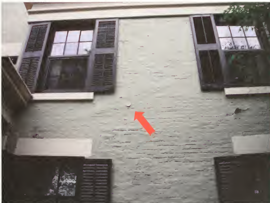
Figure 2.14. North elevation, detail of brickwork scars from formerly attached barracks building.
