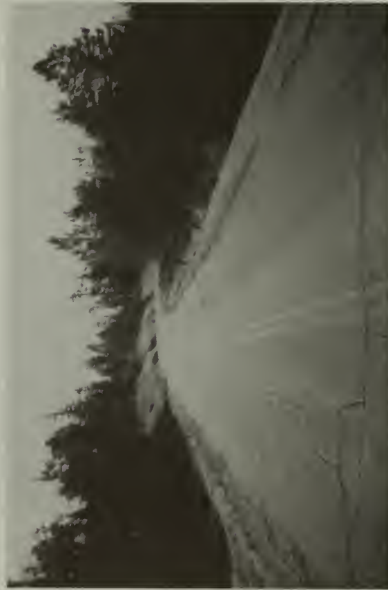
Cracked surface on Rim Road
