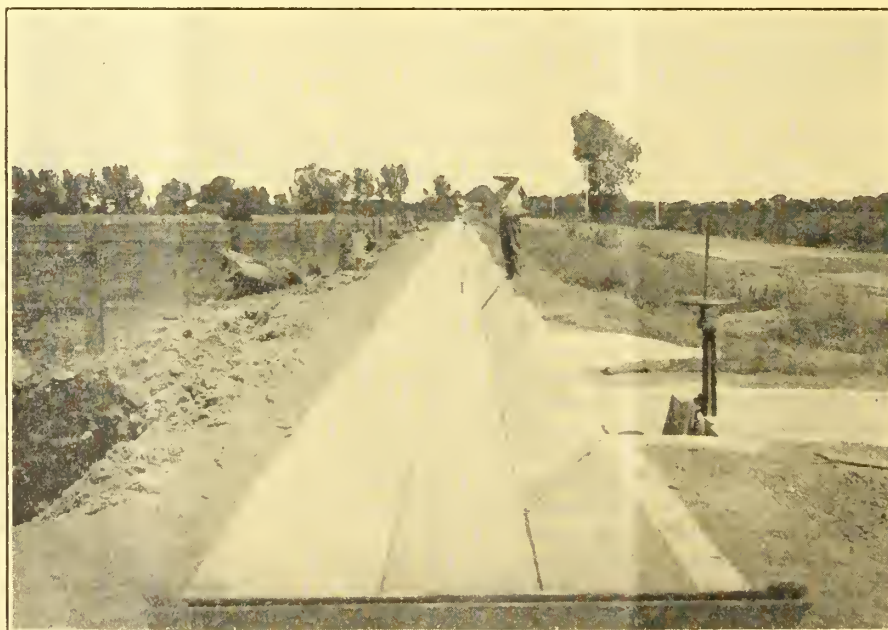
Concrete-lined lateral on the Yuma project, showing a steel water-right gate and safety overflow wasteway
