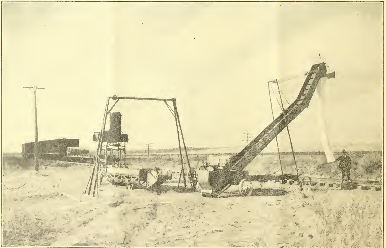
This is one of the portable beet dumps used on the Milk River project, Mont. A small gasoline engine operates the machine
