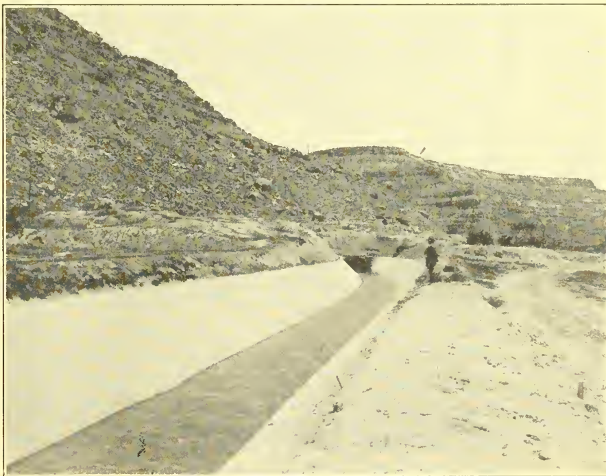
Tunnel and lined section of high line canal, Grand Valley project, Colo.
