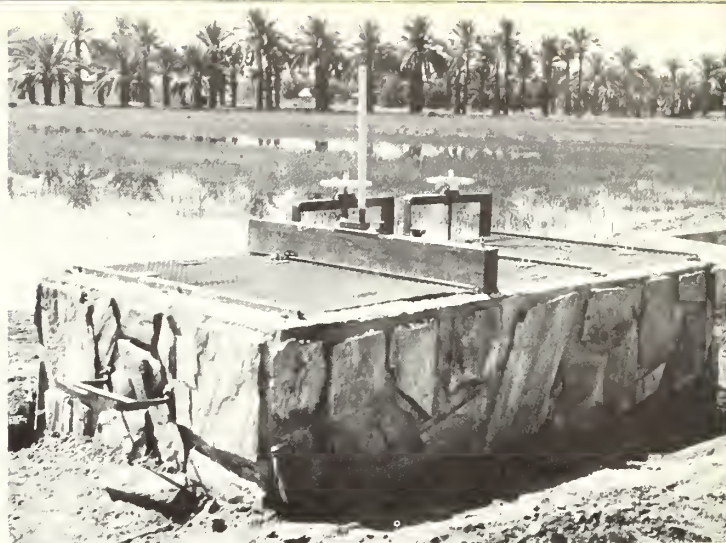
Precast slabs faced with flagstone give beauty to the superstructure of this underground lateral. The creations attract much favorable comment.
