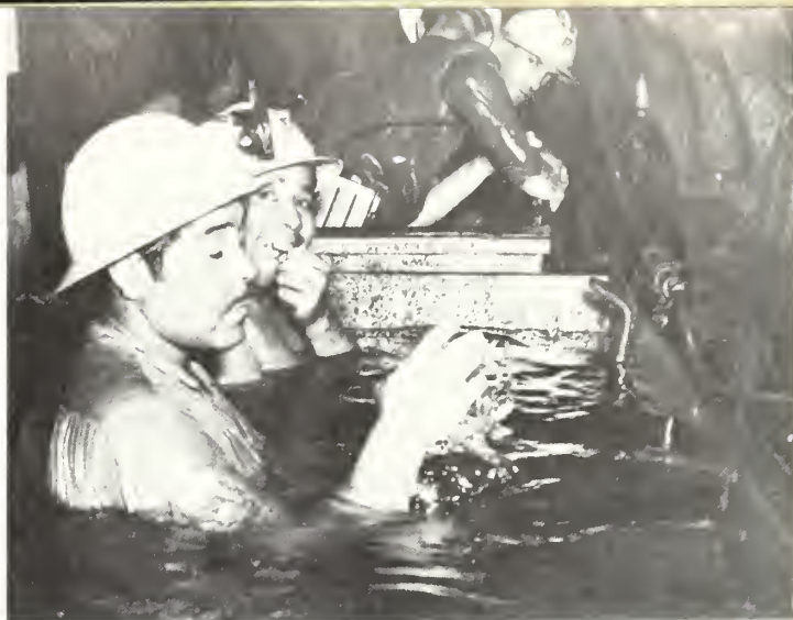
The inflow of hot water at Tecolote Tunnel caused so much difficulty that drillers could only work in very short shifts and were then hauled in and out of the tunnel in mine cars filled with cool water.
