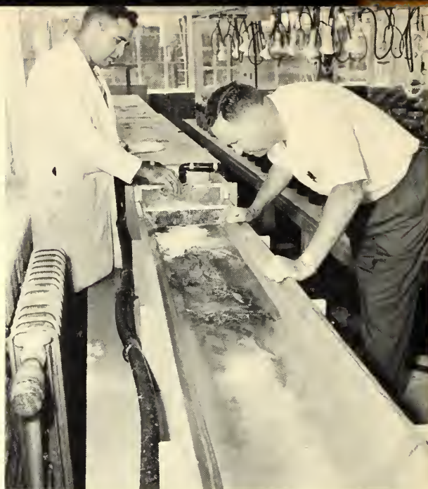
These specialists are making a herbicide test in a model irrigation canal. They are from left, Naman Otto and Thomas Bartley.
