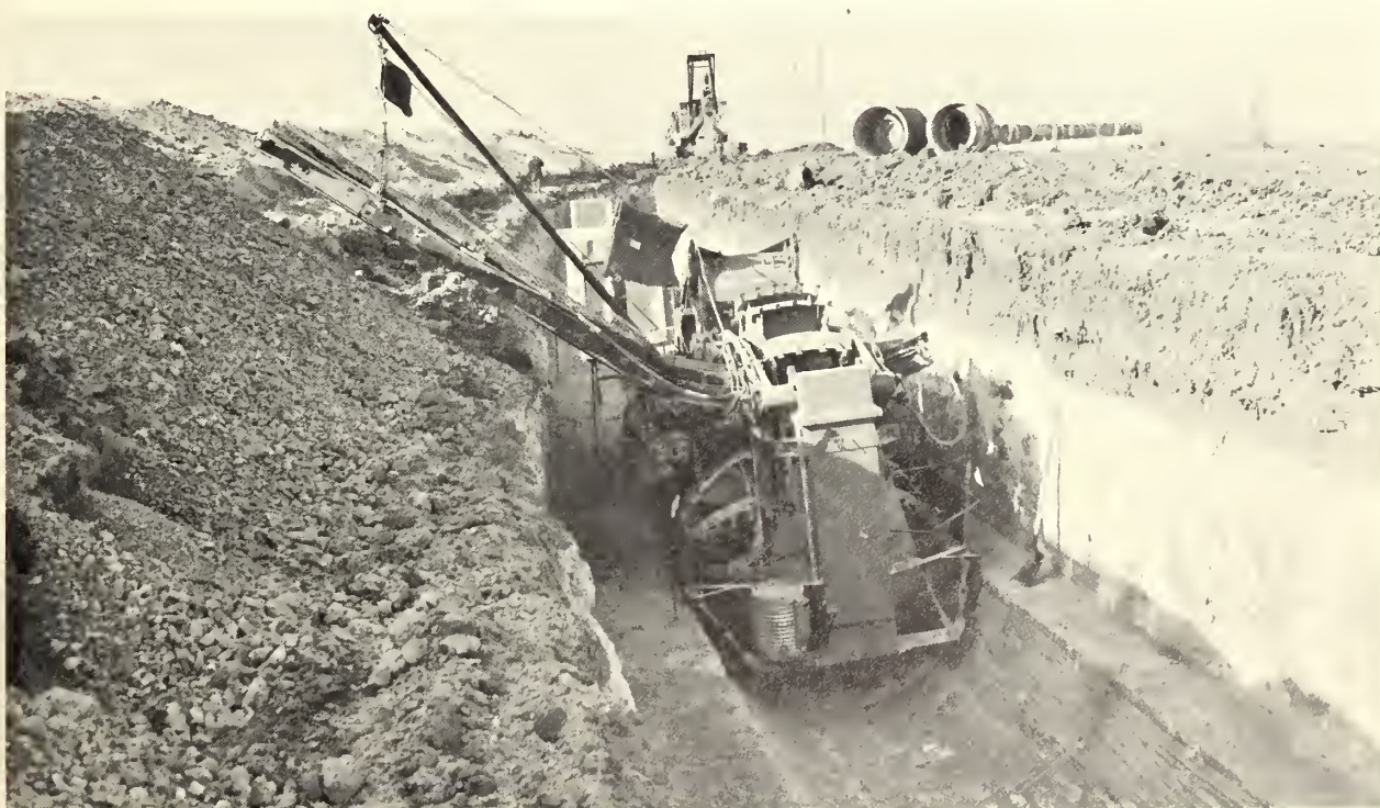
The wheel deepens the center of the trench with a rounded groove.
