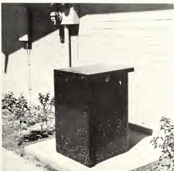
This is a power transformer on a pad sitting neatly by the service entrance of an apartment being served by an underground electric power system. Some transformers are placed underground.
