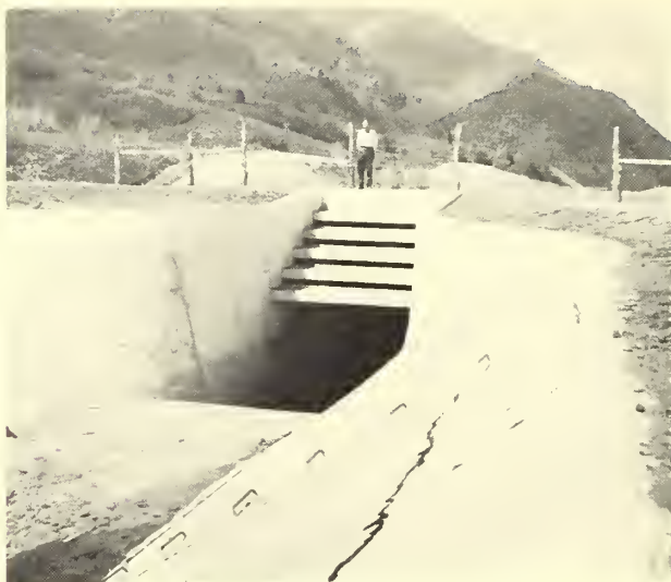
Self-rescue steps constructed into the end of this siphon on the Weber Basin Project, when in full use with water, will be helpful for persons or animals (such as deer) to climb out more easily.
