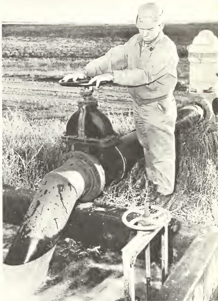
The discharge from this concrete cased well produces 1,700 gallons of water per minute.
