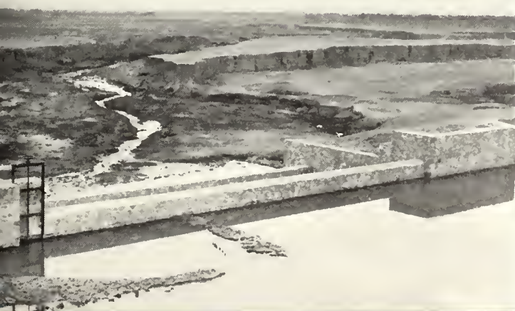
New Wasteway structure provides an escape for high storm waters, completed with help of Reclama- tion specialists.
