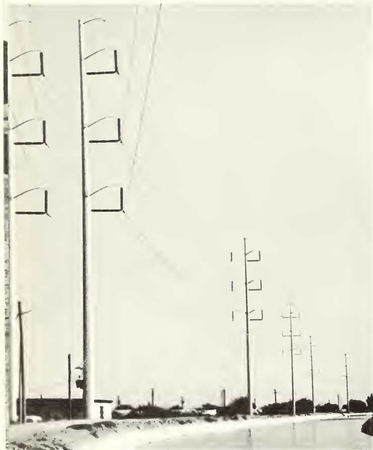
This new type of decorative, attractively painted Meyer pole supports the 230-kilovolt transmission line from Papago Buttes Substation into the Phoenix area.
