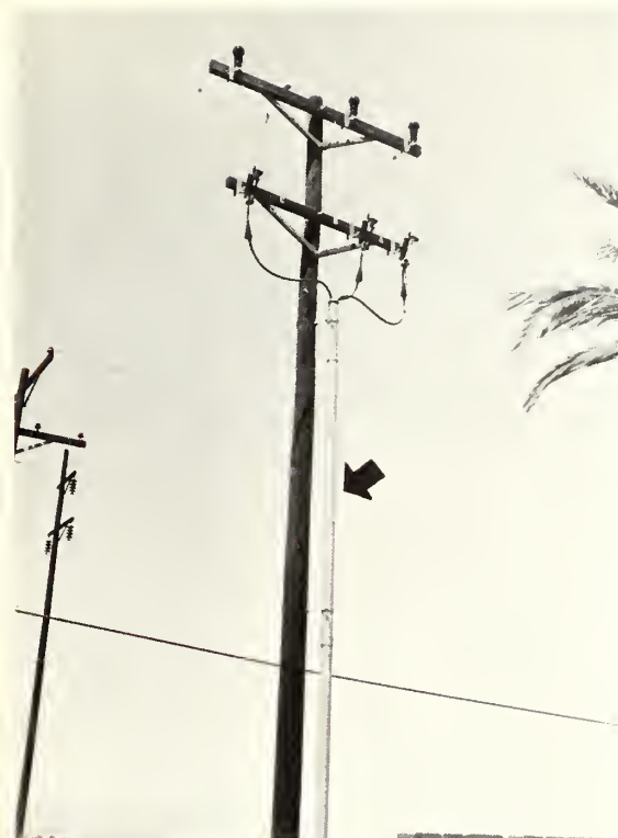
A conduit painted with light-color paint attracts no undue attention to the power going underground at the edge of a subdivision. Arrow points to conduit by pole.
