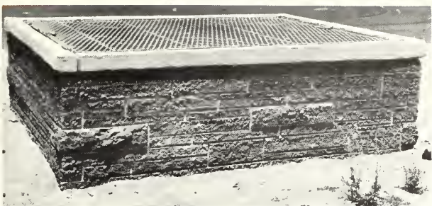
This decorative stone facing makes the irrigation structure functional as well as pleasing to the eye and permanent. (All photos, by courtesy of the Salt River Project.)
