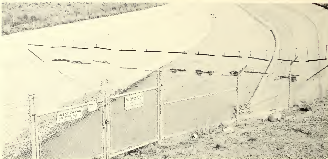
Such a concrete-lined canal as this would be more dangerous to drownings if it were not for the chain-link fence border, the warning sign, safety net hanging across the canal and the iron escape ladder at left. This is at Ephrata, Wash.
