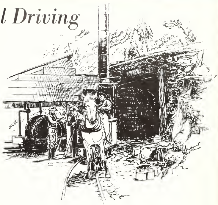
This drawing shows the removal of diggings by a horse-drawn mining car from the East Portal of Gunnison Tunnel in 1905.
