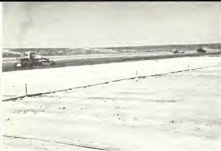
The floor of a 94-acre field, the Northeast Depression, was compacted with large machinery in 1963, and test plots were sprinkler-irrigated to examine the permeability of the soil for holding salt brine.
