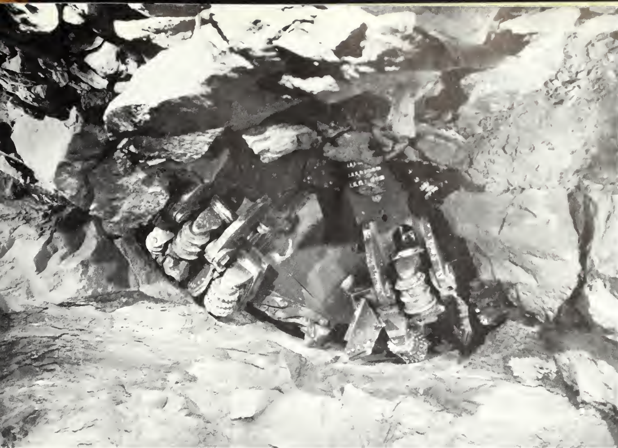
The cutter head of the 20-foot diameter tunnel-boring machine is shown here as it completed "holing-through" Tunnel No. 1 on the Navajo Indian Irrigation project, N. Mex., on March 19, 1966.
