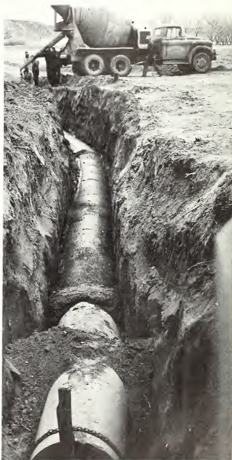
Goshen Irrigation District installing cast-in-place concrete pipe on the North Platte project, Wyo., in 1959—financed by Rehabilitation and Betterment Funds.
