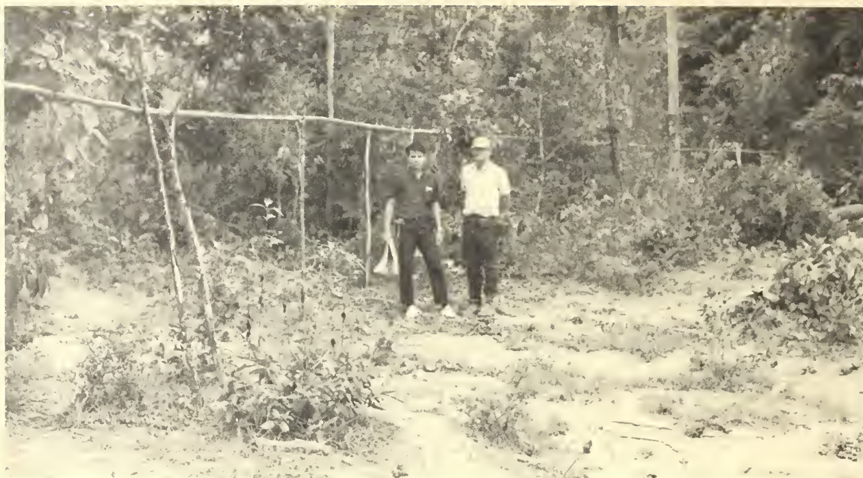
Above. Hollow bamboo pipe carrying water to the temple is shown above the heads of the two men. At right. A fellow can take a refreshing drink at this junction in the pipe.
