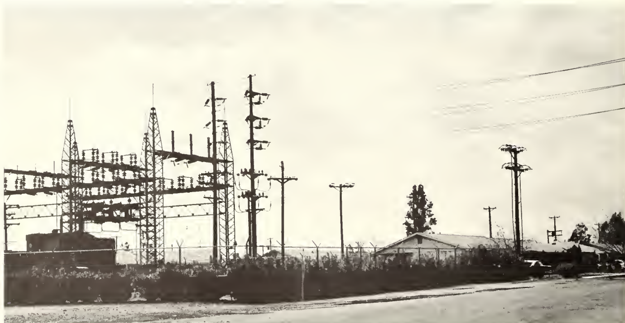
This new type of decorative, attractively painted Meyer pole supports the 230-kilovolt transmission line from Papago Buttes Substation into the Phoenix area.
