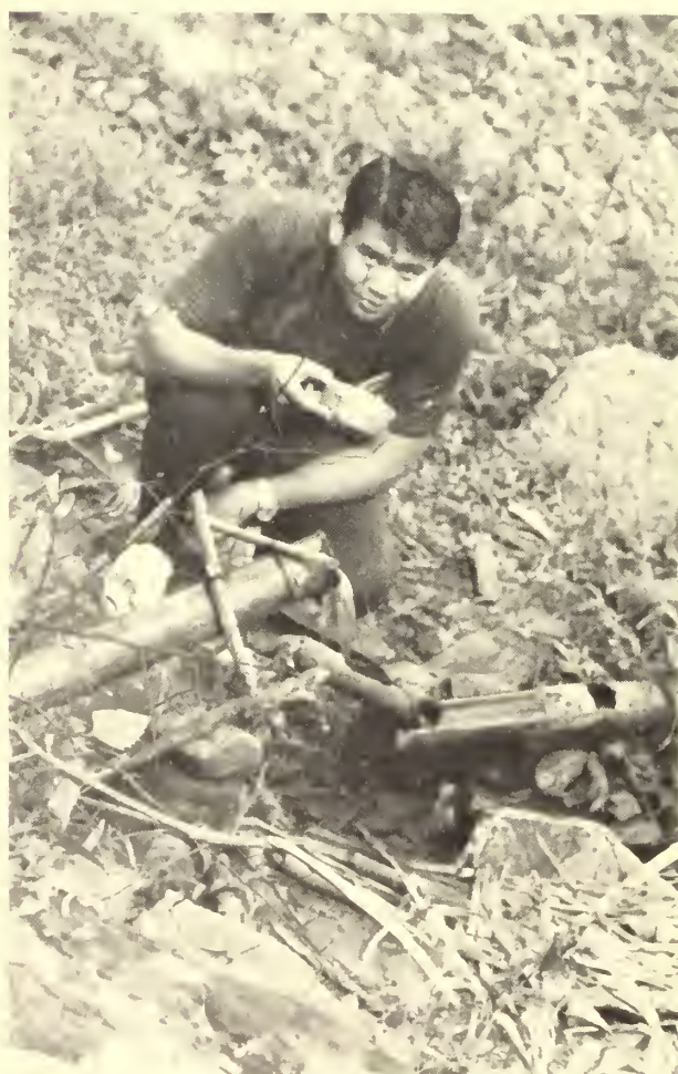
Above. Hollow bamboo pipe carrying water to the temple is shown above the heads of the two men. At right. A fellow can take a refreshing drink at this junction in the pipe.
