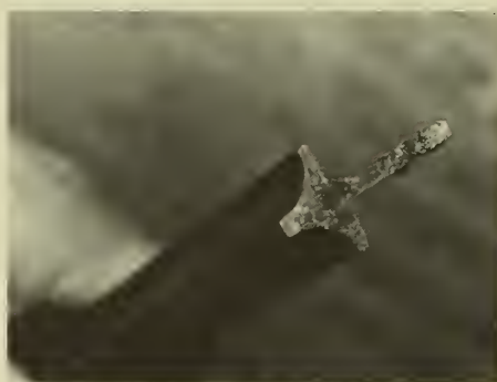
Figure 10. Replacement steel window section used primarily in the sill areas. Photo: Clio Group.
