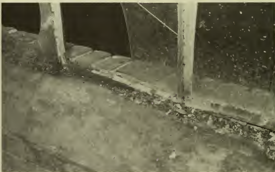
Figure 5. Sill corrosion typically found on 95% of the windows. Photo: Clio Group.
