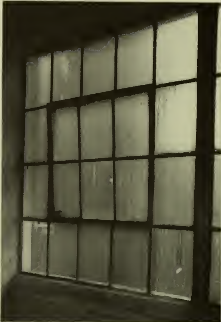
Figure 1. Typical multi-light steel window with ventilator as seen from the interior. This window exhibits typical pre-rehab conditions including sill corrosion, missing hardware and a poorly operating ventilator. Photo: Clio Group.
