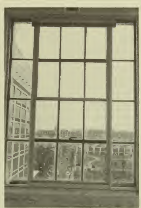
Figure 12. Installed interior triple-track storm window with fixed sidelights. Photo: Clío Group.
