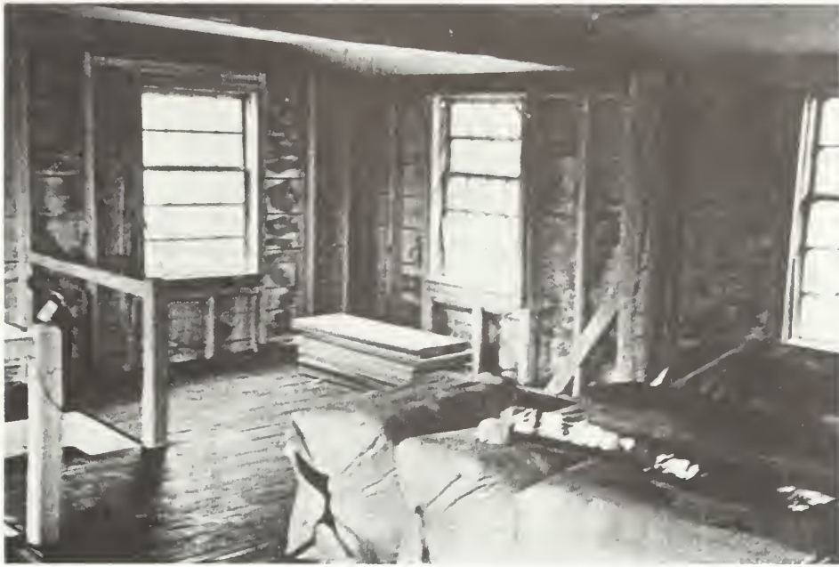
Second floor of WIGS, during rehabilitation work. The exterior wall boards were sprayed with an insecticide "Dursban" then coated over with a white latex paint. View of northeast corner of second floor.
