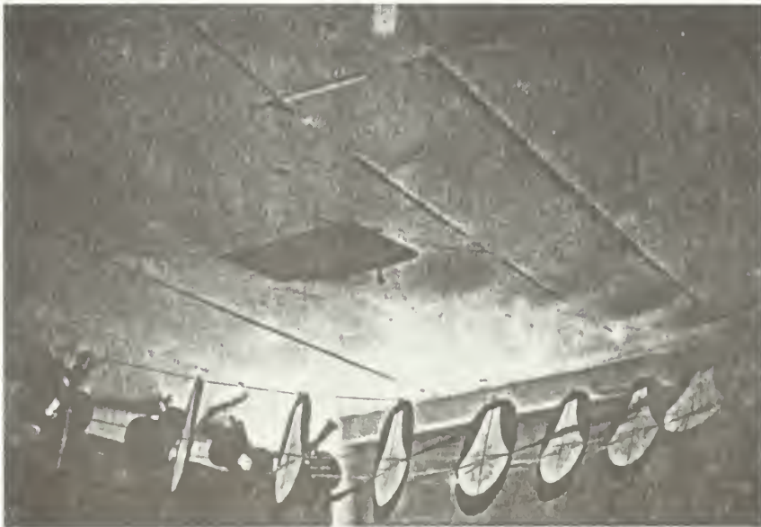
Figure 38. West India Goods Store, interior of first story, bay C, showing hole 12 by 9-1/2 inches cut in wood ceiling.
