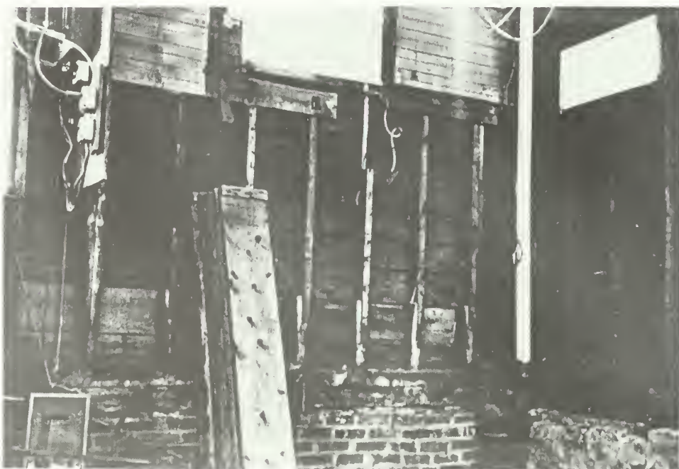
North east corner of WIGS, on the first floor showing reconstruction of end bay of building, probably dating from the restoration of ca. 1920.
