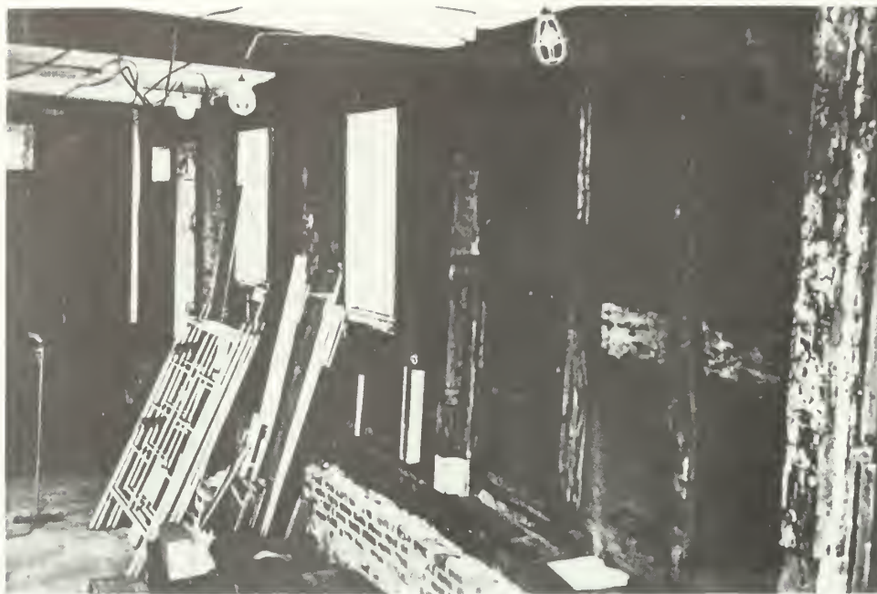
Interior of WIGS after joists and floor boards were removed from the first floor. View of east wall after interior wall boards were removed. Exterior wall sheathing was sprayed with an insecticide, "Dursban" which in turn was coated with an acrylic to prevent sublimation of the insecticide crystals.
