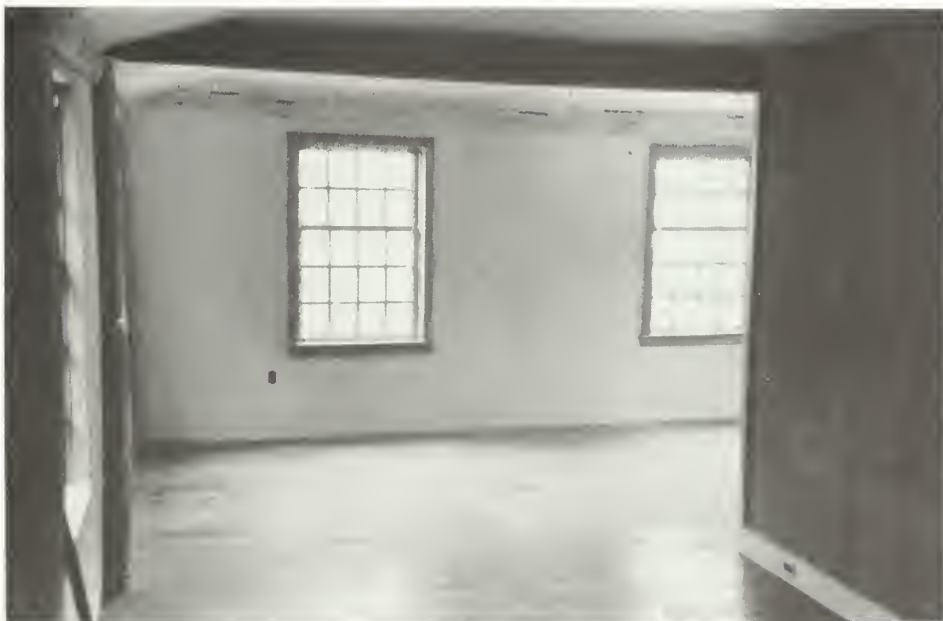
Interior partition, second floor, WIGS, showing rock lath nailed to walls.
