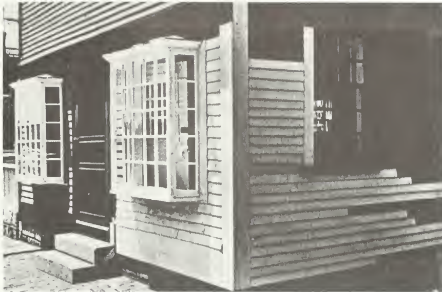
WIGS building after repair work was completed to the southwest corner in 1983. Both storefront windows were replaced at this time. The building was damaged in an automobile accident, November 1983.
