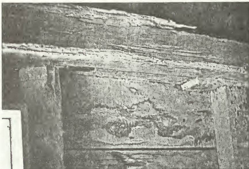
Figure 42. West India Goods Store, interior of second story, south wall, showing girt with vacant stud pocket and two studs in nonhistoric positions. The stud on the right is in the approximate center of the south wall.
