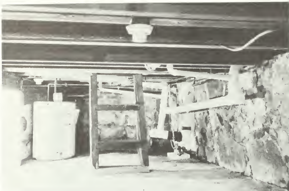
View of crawl space below first floor after the installation of the hot water heater, electrical, plumbing, heating and fire detection systems were completed. View shows east half of crawl space at north end.
