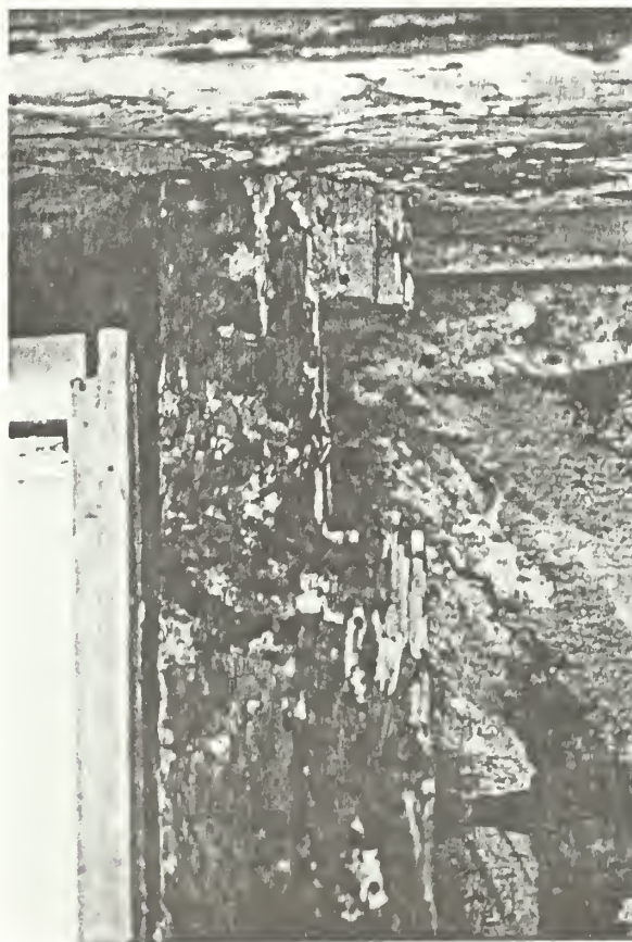
Figure 41. West India Goods Store, interior of second story, south wall, showing stud with cut to receive possible window head.
