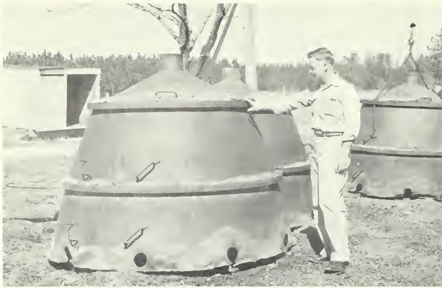
DIG THIS CRAZY BEEHIVE --Talbot County Ranger Harvey Butler looks over one of the portable charcoal "beehive" dry kilns used at Talbrion Farm. Each kiln has a half-cord capacity and produces about 400 pounds of charcoal from a single charge.
