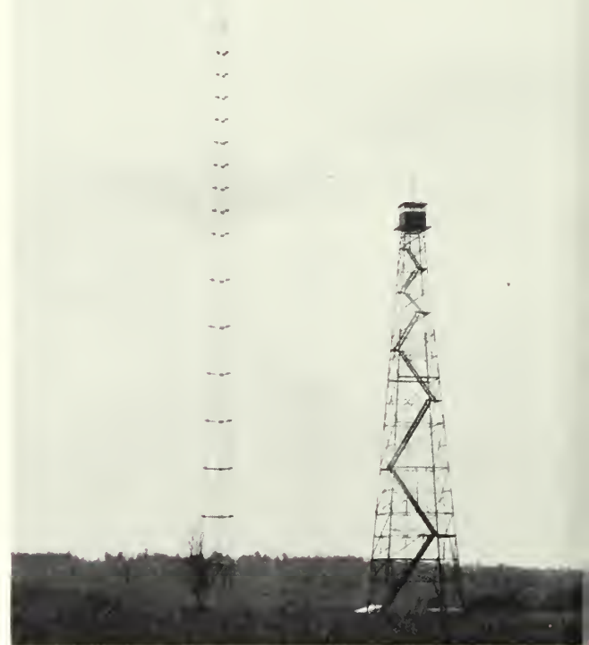
Oh, that towerin' feelin'. The GFC's new 400-foot radio antenna will soon be beaming messages direct to every part of the state. It replaces the old 100-foot antenna which was mounted on the fire tower at right.
