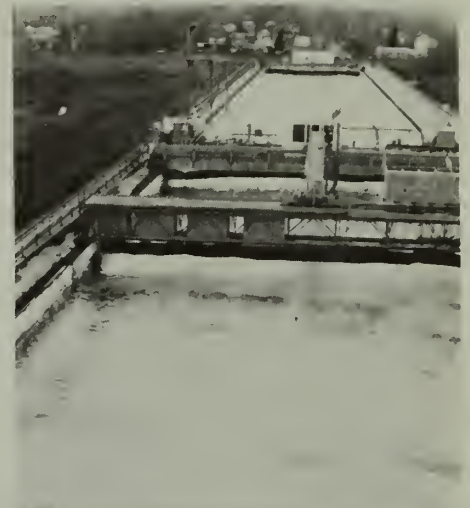
EPA test tank at Leonardo, N.J. serves as demonstration and training facility for exercises in handling oil and hazardous material spills.
