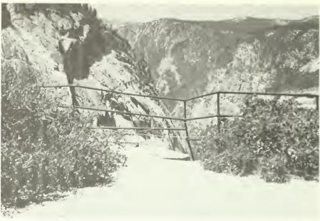
Defective railing at overlook above precipitous cliff. Standards for location and maintenance are poor.
