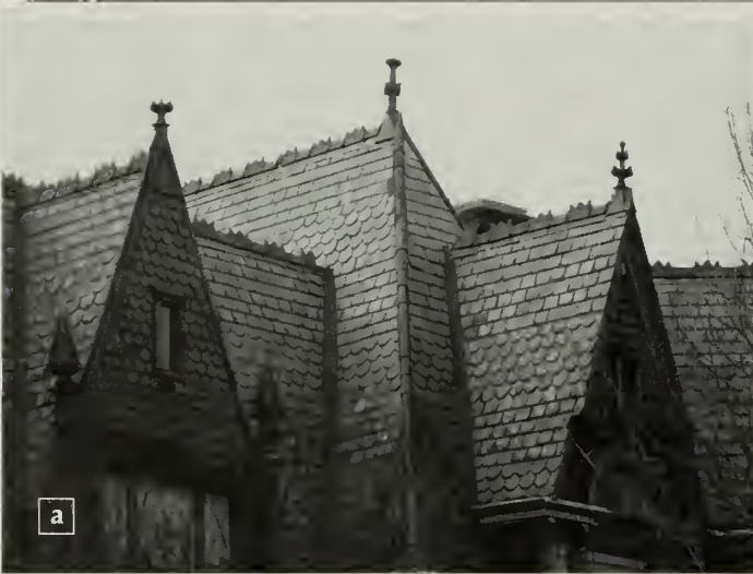
Figure 7. Ridge caps and cresting can be elaborate. Ridges are formed at the long horizontal juncture of two roofing slopes and capping protects this joint from moisture. In (a), a terra cotta capping with a decorative profile complements the finial over the various roof peaks. In (b), the mansard roof has a decorative iron cresting at the break between the lower and the upper roof slopes.
