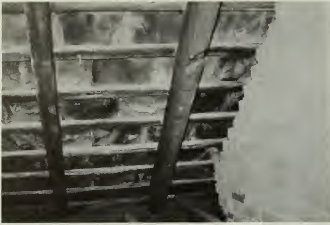
Figure 15. View of the underside of slates laid on open sheathing shows that delamination and flaking is just as bad or worse on the underside of slates as on the exposed surface. This is why most slates cannot be flipped over for reuse.
