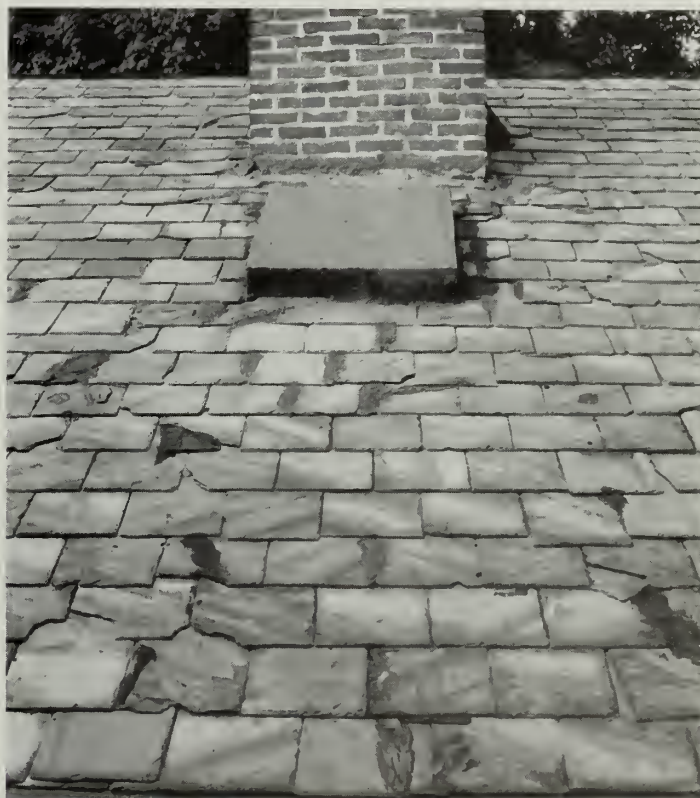
Figure 20. This roof has been poorly repaired numerous times in the past. The installation of mastic to seal out moisture has only exacerbated the problem. A timely repair and good maintenance could have extended the life of this roof.
