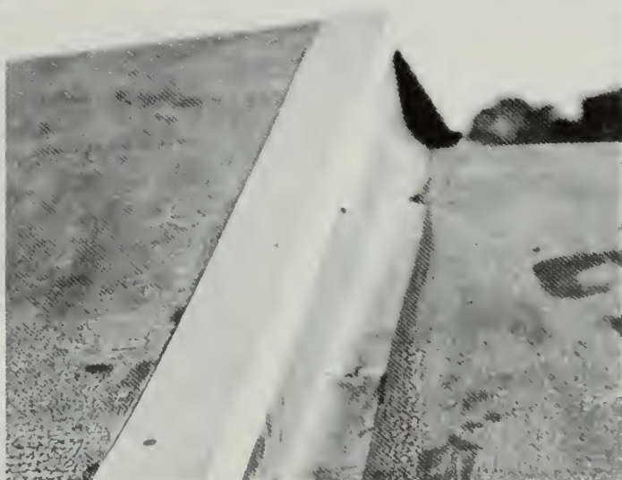
(f) Lead coated copper flashing was installed throughout. Seen is the offset between the portico roof and the main roof in progress.
