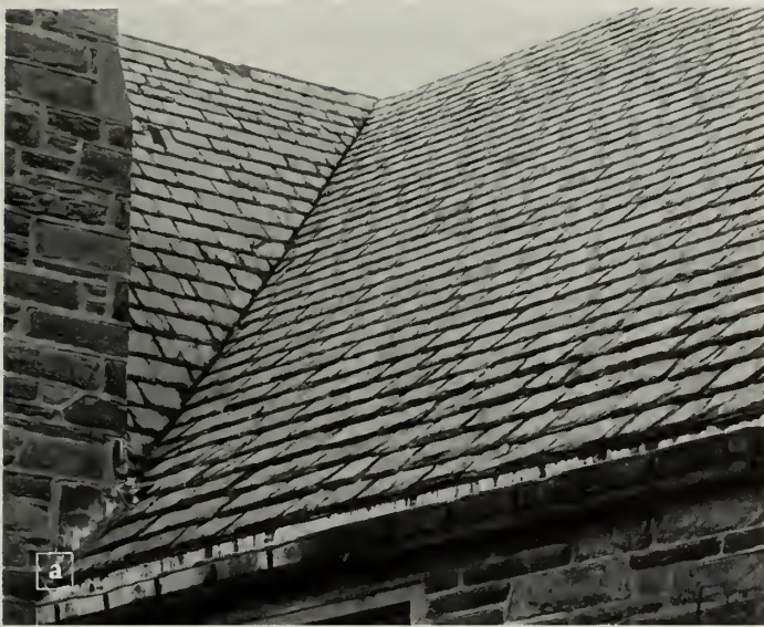
Figure 9. Valleys are formed at the internal angle of two roofing slopes. Flashing is often placed under the slate to increase moisture protect at this vulnerable joint. Show in (a) is a closed valley where the slates are held tight to the valley line. (b) illustrates of a round valley where the transition between the two slopes is a continuous curve. It requires careful workmanship and an experienced roofer.
