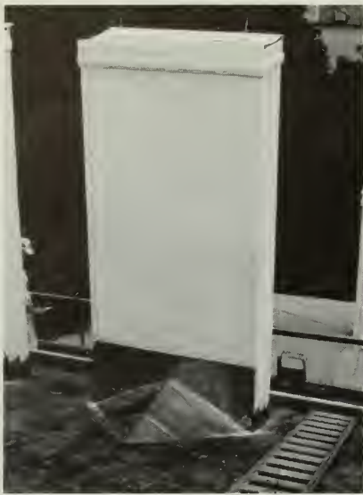
(g) Masonry chimneys were repaired and metal crickets were fabricated at the chimneys.
