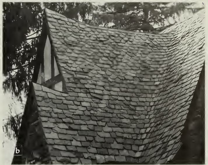
Figure 9. Valleys are formed at the internal angle of two roofing slopes. Flashing is often placed under the slate to increase moisture protect at this vulnerable joint. Show in (a) is a closed valley where the slates are held tight to the valley line. (b) illustrates of a round valley where the transition between the two slopes is a continuous curve. It requires careful workmanship and an experienced roofer.
