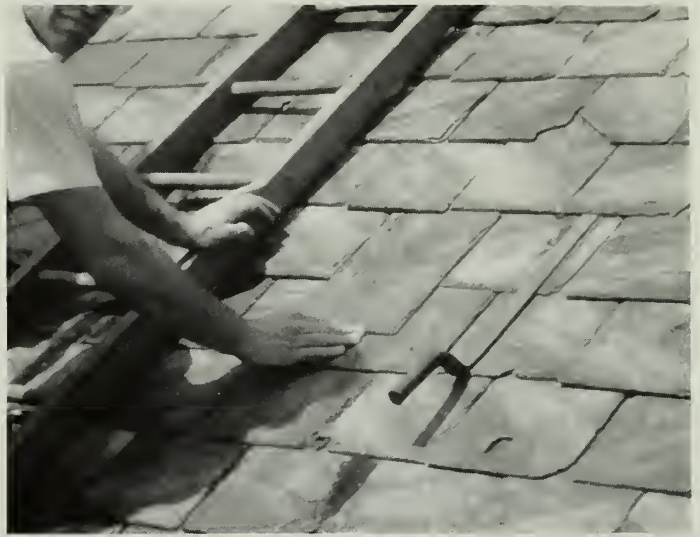
(b) A replacement slate is slid into place.
