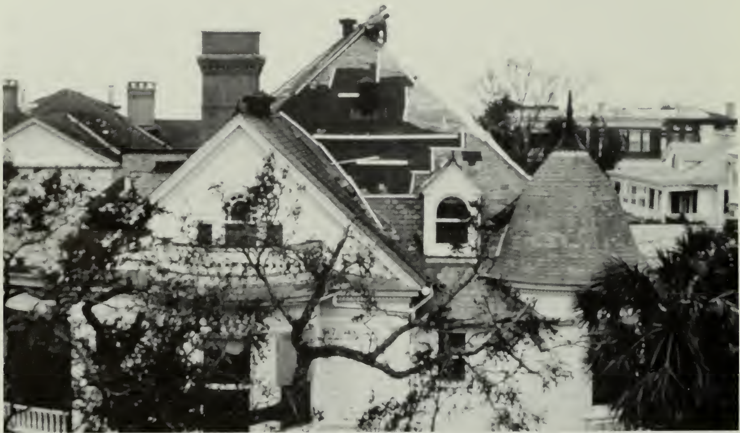
Figure 21. As a result of hurricanes and other disasters, it may be necessary to temporarily stabilize a roof until materials can be obtained and a qualified roofing contractor hired. Heavy roofing felt was stitched into this slate roof to stop moisture penetration until matching slate was obtained for repair. Significant slate roofs should not be stripped off and replaced with asphalt shingles. Photograph courtesy of the National Park Service.
