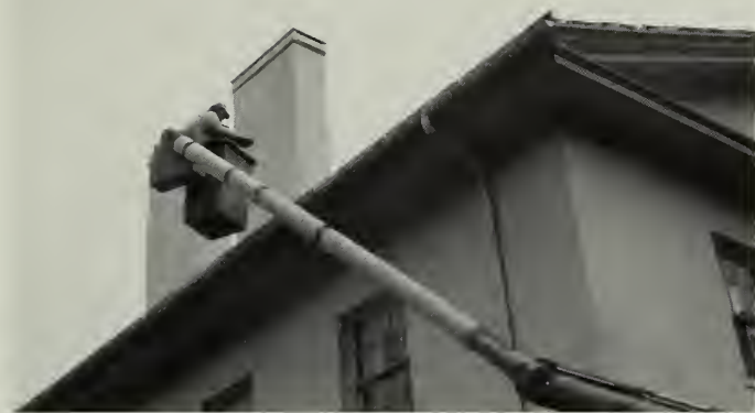
Figure 23. Slate roofs should not be walked on if at all possible. For large projects, lifts can be used to inspect roofs periodically to assess maintenance needs. Photograph courtesy of the National Park Service.
