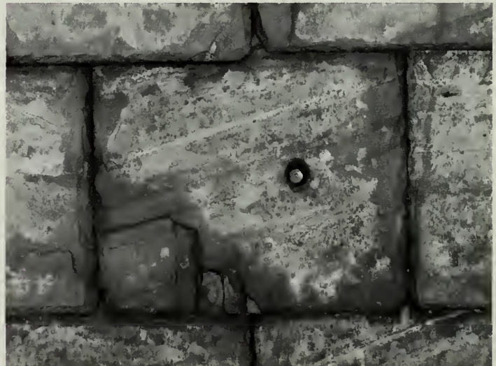
Figure 16. Detail view of a slate which has been punctured by the head of a nail used to secure the slate in the course below. Likely, the nail was not hammered in far enough when originally installed.
