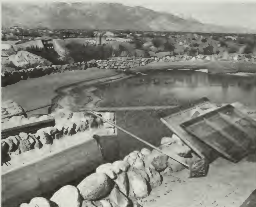
Photo 41: Reservoir Stilling Basin, Manzanar War Relocation Center; Toyo Miyatake Photograph, Toyo Miyatake Studio, San Gabriel, California.
