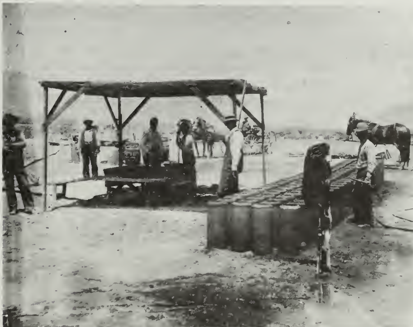
Photo 6: V. C. Lutzow at the construction site of Manzanar making cement pipe for the Manzanar subdivisions.
