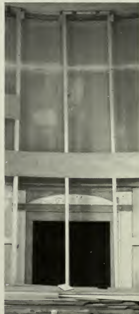
Figure 3. Vibrations generated during construction may necessitate the installation of temporary support for such fragile features as plaster ceiling cornices and soffits. Drawing: Villard Houses — courtesy of Emery Roth & Sons Architects, P.C. Photo: The Octagon, Lonnie Hovey, AIA.
