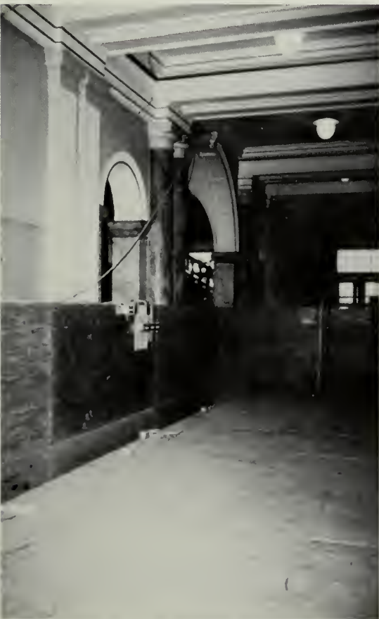
Figure 5. To provide for adequate floor protection in the New Jersey State Capitol, this area was swept clean, then covered with polyethylene sheeting to protect against spills and dirt abrasion. Fiberboard (1/2" thick) was placed over floors and the joints sealed with tape. Finally 1/2" plywood was laid with all joints taped. This floor protection system has been successful over many years of use and is recommended in major construction areas, and where tile, marble, parquetry wood, or other historic flooring is involved. Photo and drawing: Ford Farewell Mills and Gatsch Architects.
