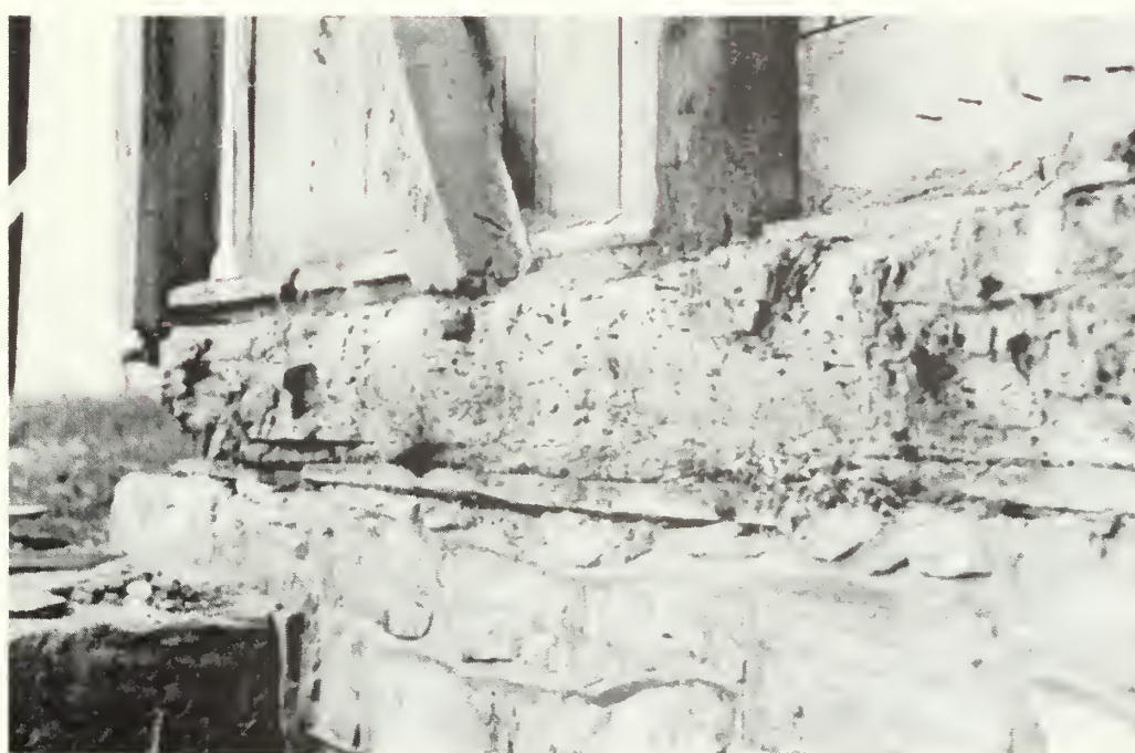
Figure 130: Condition of exterior of northwest granary during 1992 repair work by park maintenance crew. Note deteriorated condition of sill due to insect attack and moisture damage.
