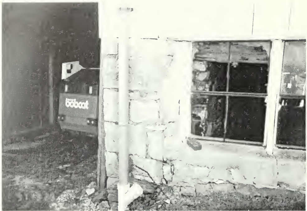
Figure 197: New downspout at the dairy area leading into sub-grade drainage system (north corner of the barn).
