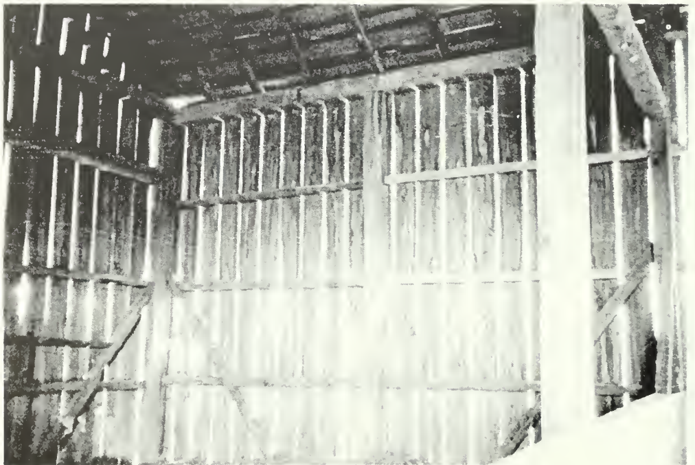
Figure 59: Interior of the barn showing the gaps providing ventilation between boards of wood siding.
