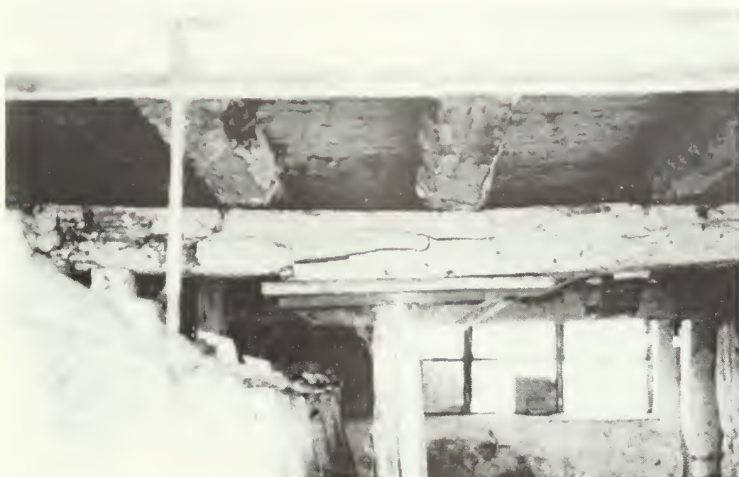
Figure 108: Failed girder on northeast side of barn prior to repair (1985).
