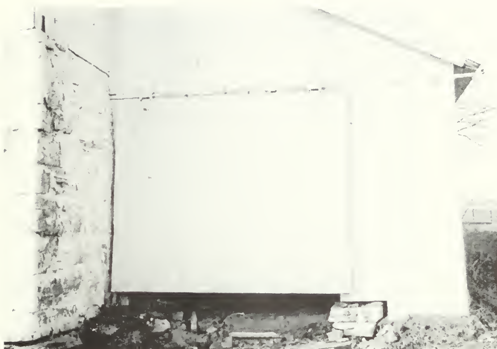
Figure 129: Door at southeast elevation of implement shed. Note erosion at base of door.
