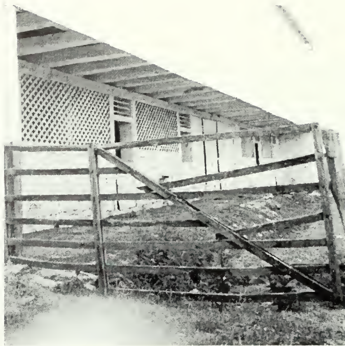
Figure 201: Gate at the south side of the barn is non-original and in a state of disrepair..
