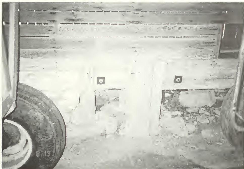
Figure 175: Deteriorated siding and foundation of shared wall between corn crib and wagon shed.
