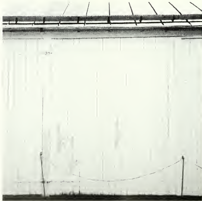
Figure 202: Typical peeling paint on the surface of the barn (northwest elevation).
