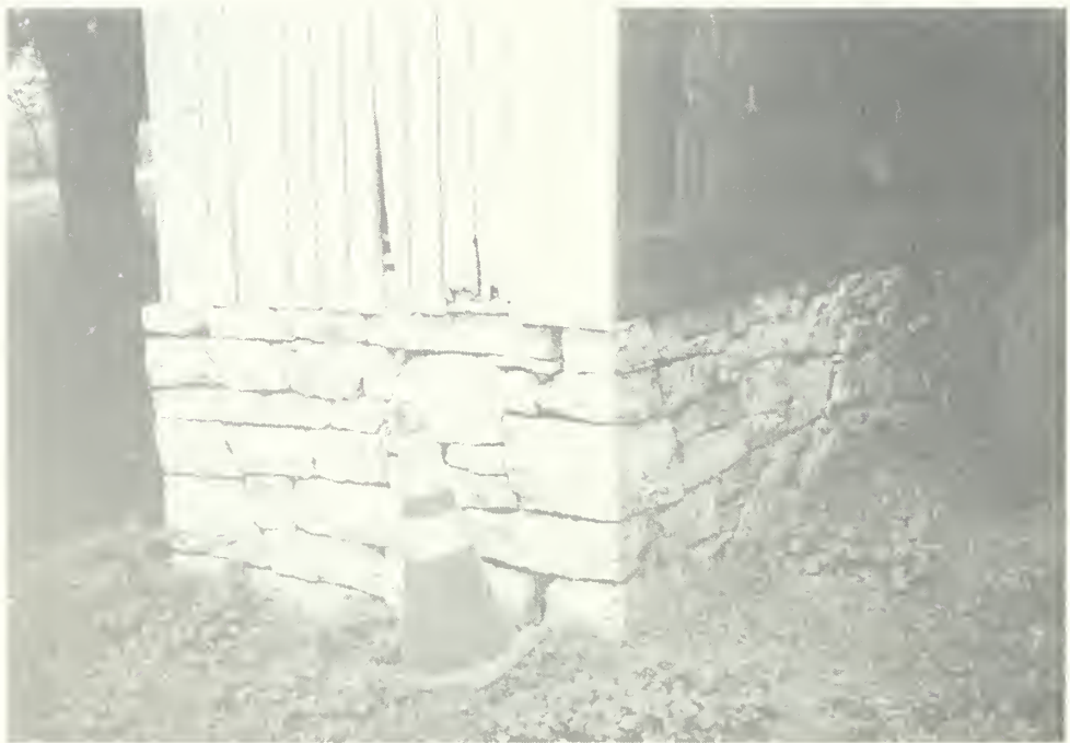
Figure 174: Deteriorated foundation wall of corn crib (southeast elevation).
