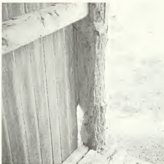
Figure 176: Post at front of corn crib damaged by insect attack.
