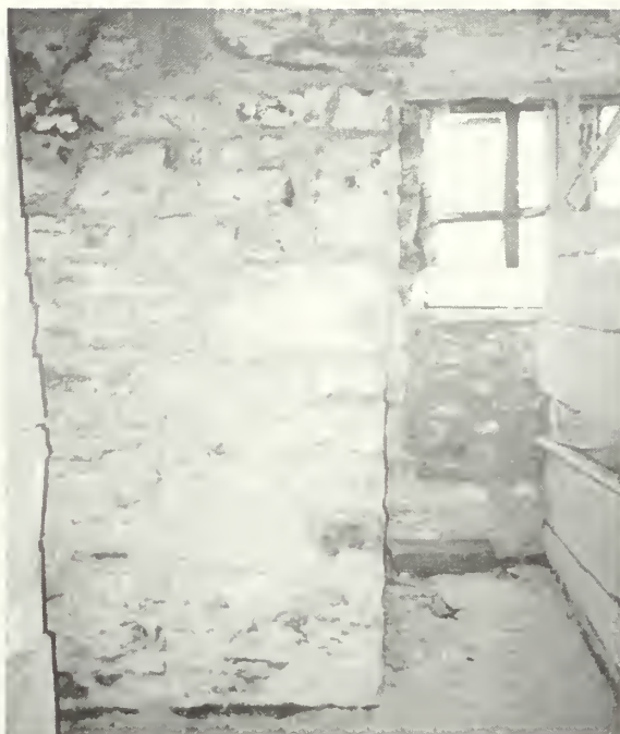
Figure 119: Repointed foundation wall at the west end of the dairy area.
