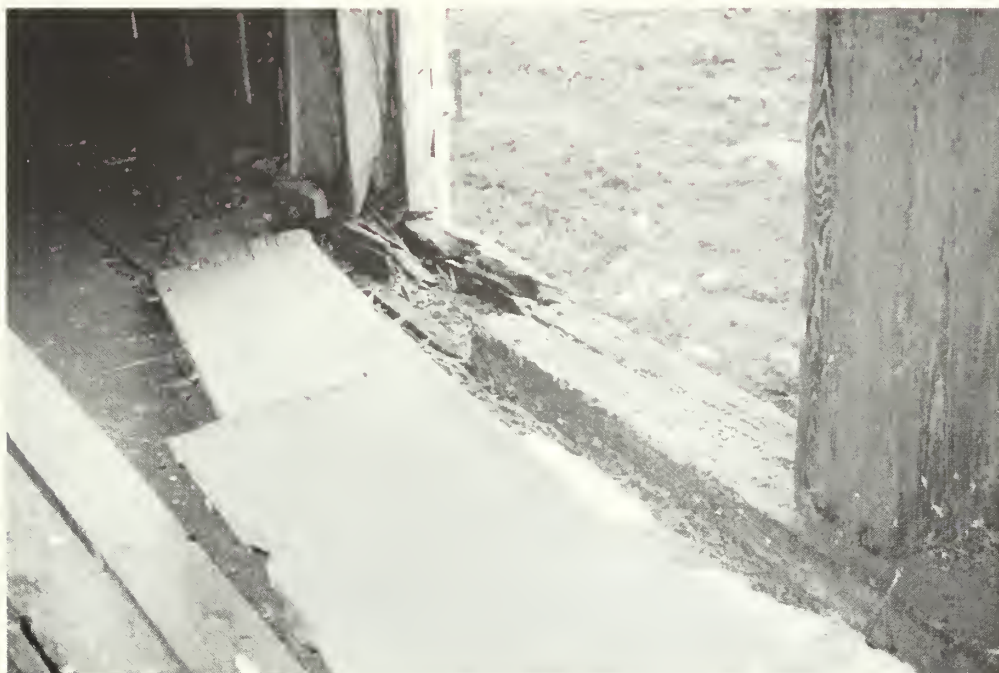
Figure 85: Rotted sill at threshold of winnowing door.
