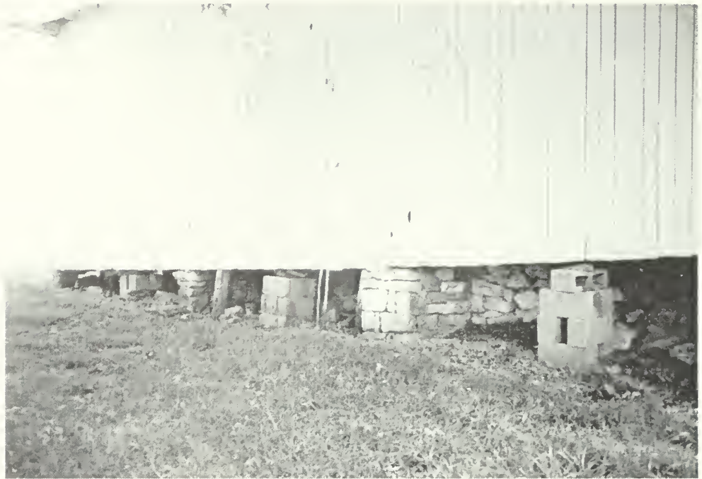
Figure 173: Exterior of corn crib (southwest elevation). Note deteriorated state of foundation.
