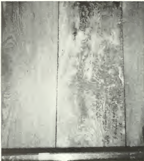
Figure 131: Insect damage at interior siding of north granary.
