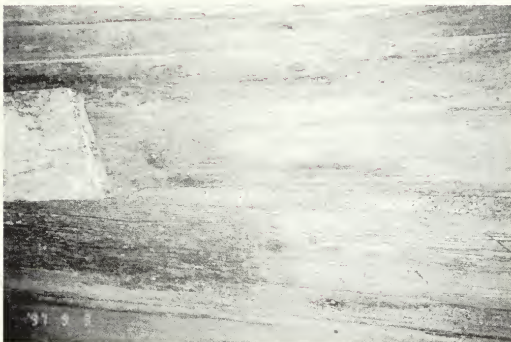
Figure 148: Original, wood threshing floor. Damaged area of the floor was patched with galvanized metal.
