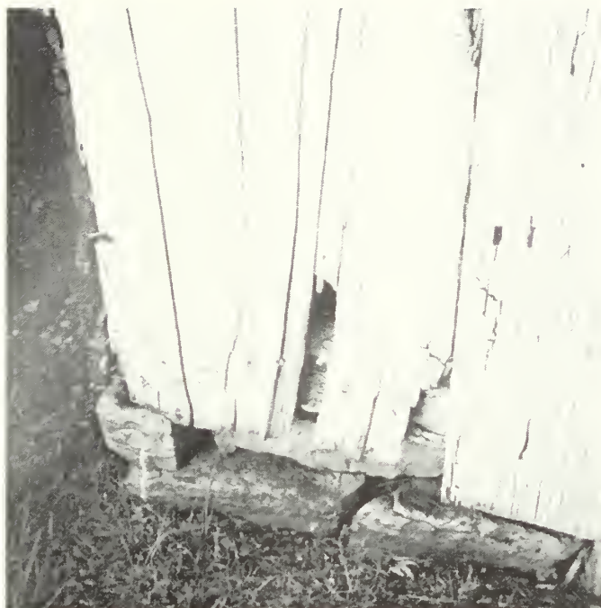
Figure 179: Damaged siding at exterior of corn crib.
