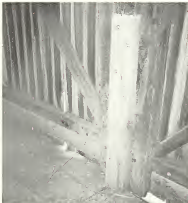
Figure 183: Post repaired by park in 1993 (due to Powder Post Beetle attack).
