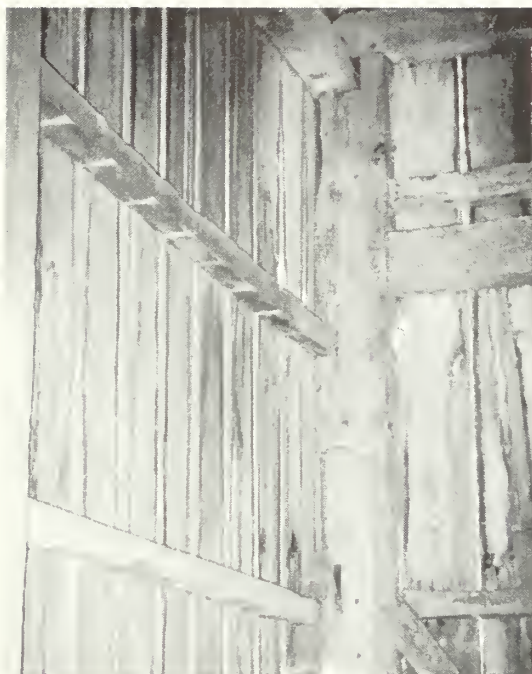
Figure 92: Main vertical member at the southern corner of the barn, which has been severely damaged by insects. Reinforcing was added at some point.
