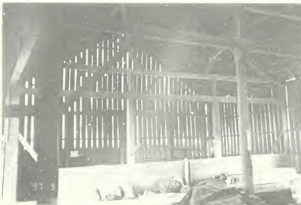
Figure 56: Interior view of the barn showing the structural bents.
