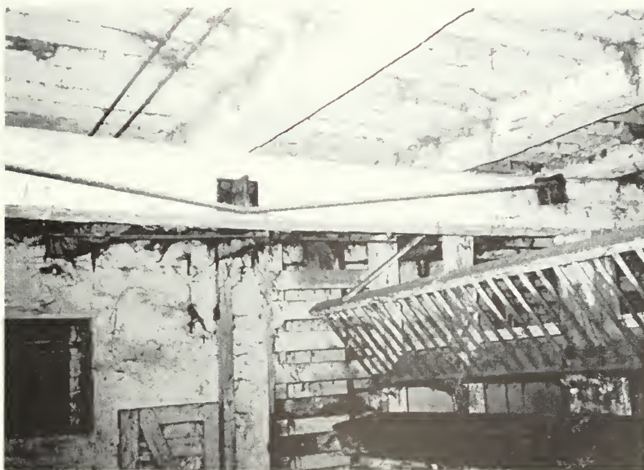
Figure 81: Steel reinforcement at basement beam of Piper Barn.
