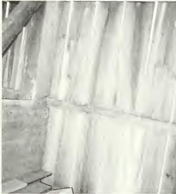
Figure 133: White bloom visible on interior siding. This is likely a fungal growth.
