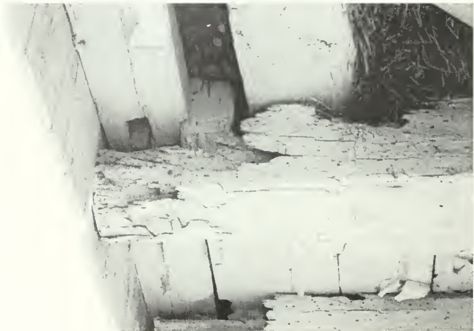
Figure 91: Detail of deteriorated joist ends.
