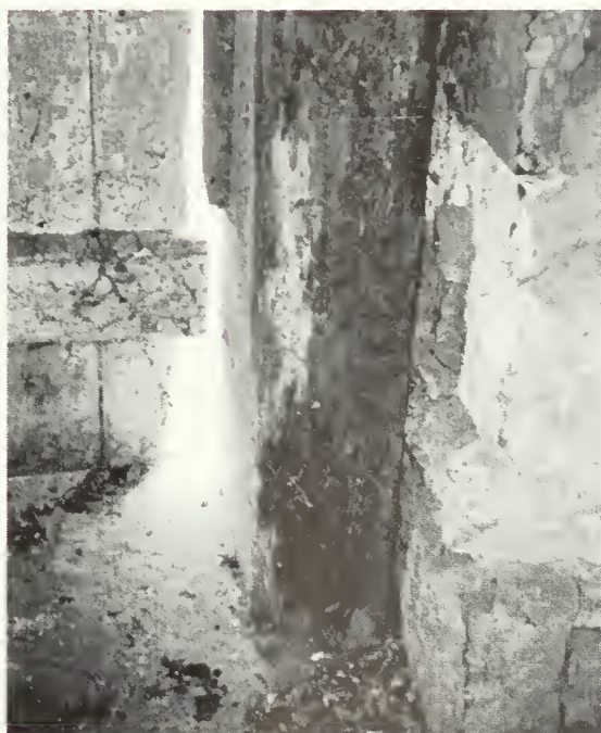
Figure 192: Wood door frame of split door on the southeast elevation. Note insect attack.
