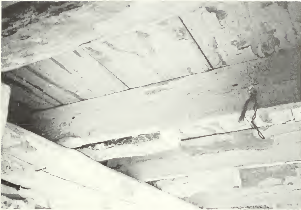
Figure 159: Original log joist cut below outshed/granary. Typical under both outsheds.
