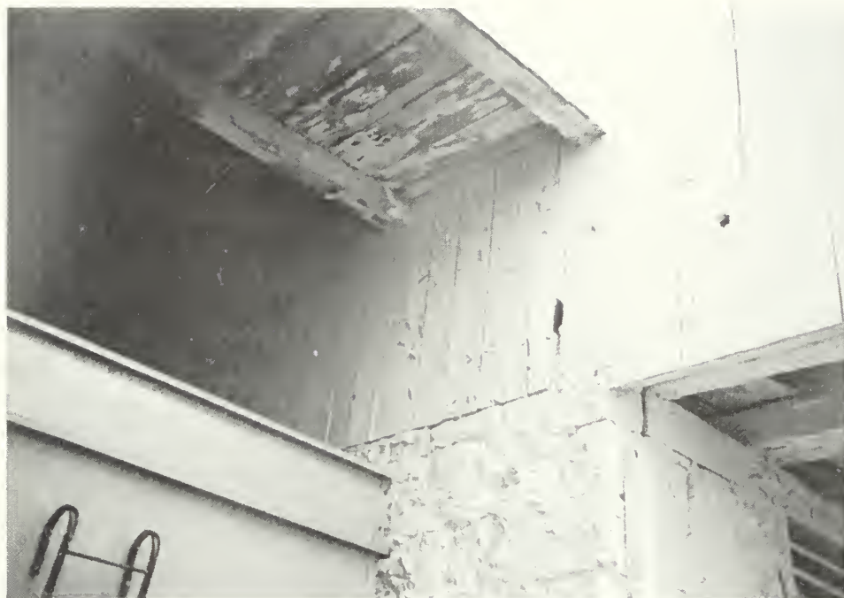
Figure 171: Damaged siding at south end of wagon shed.
