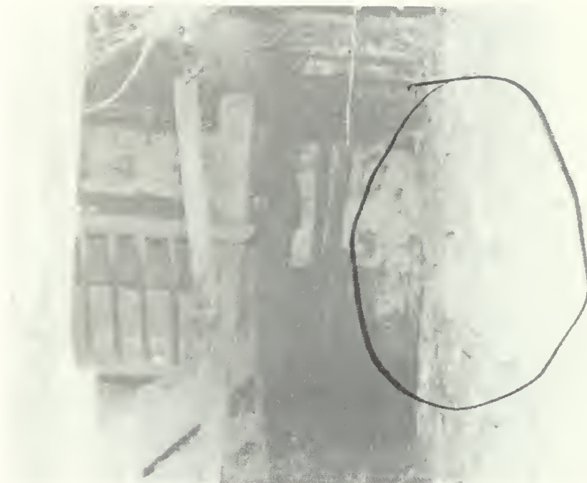
Figure 94: Bowing of the wall was evident as far back as 1985, as is apparent in this photograph.
