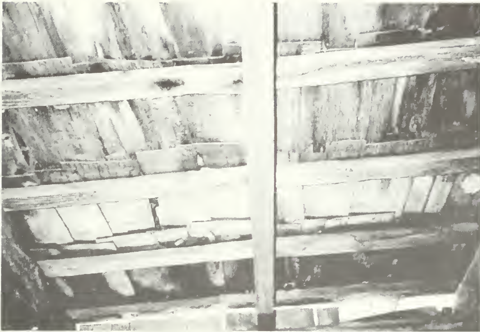
Figure 52: Biaxially tapered shakes at underside of Mumma Farmstead hog pen roof.
