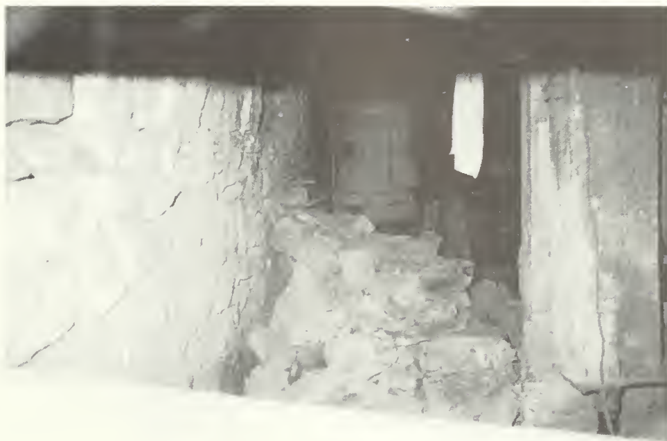
Figure 96: Collapsed northwest foundation wall. The wall came down in September of 1997 and was rebuilt in December of 1997.
