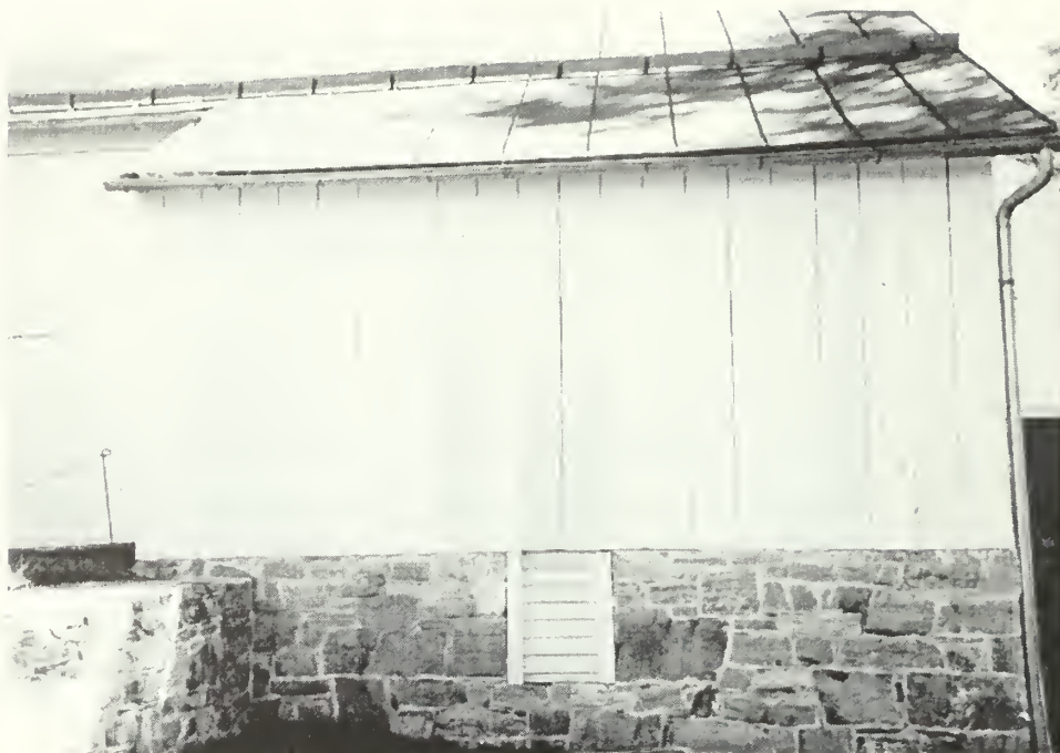
Figure 135: New siding at the west granary.
