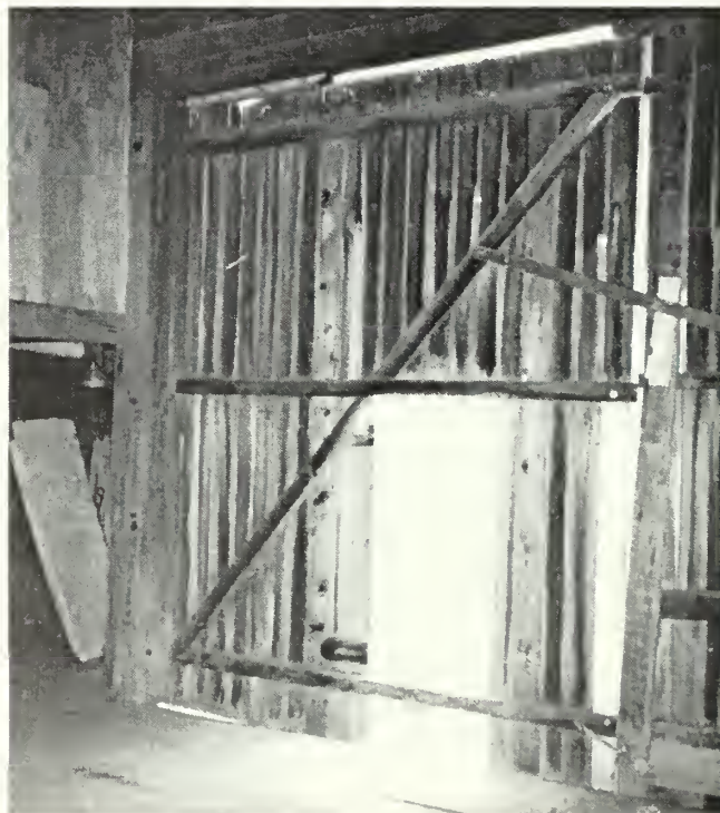
Figure 55: Interior side of the western-most wagon door. The smaller 'door-within-a-door' is open for easier access.
