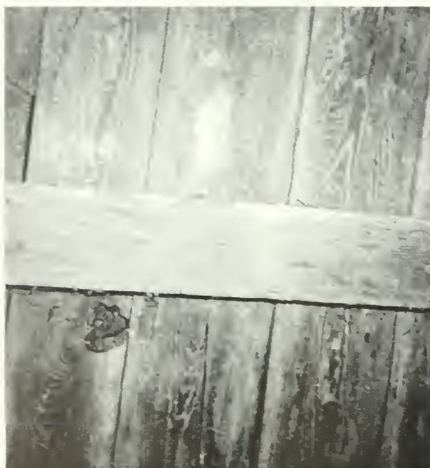
Figure 132: Insect damage at interior siding of west granary.
