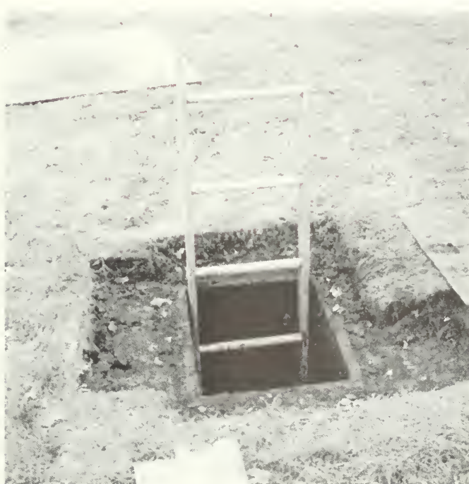
Figure 100: Cistern entry hatch.
