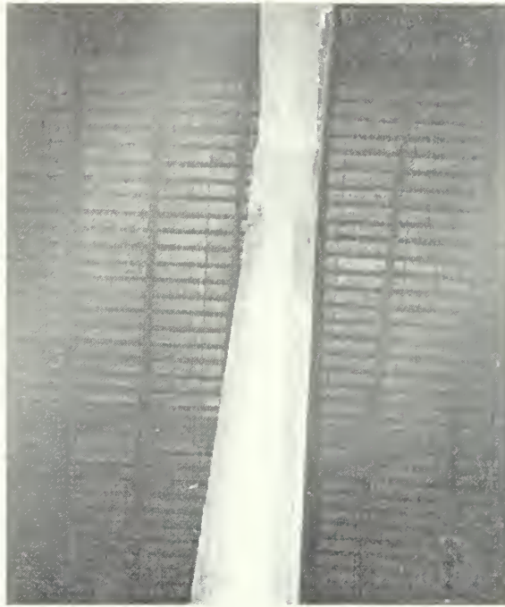
Figure 86: Chamfered post of central bent.
