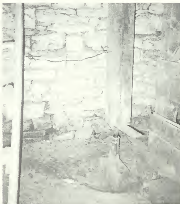
Figure 95: One of two temporary jacks and posts carrying the load of the structure above the northwest foundation wall.
