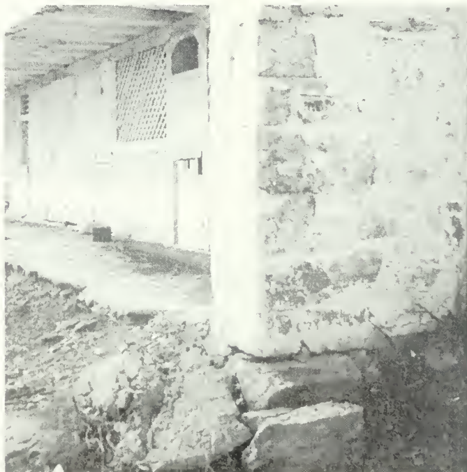
Figure 198: Moisture damage at east corner of barn due to faulty drainage.
