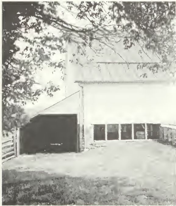
Figure 142: View of the windows added to the north corner of the barn at the time the barn was converted for dairy use.
