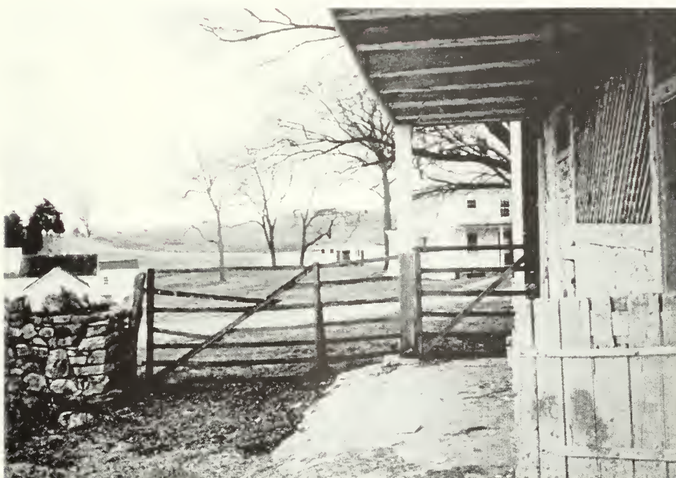
Figure 39: Posted-forebay end at southern corner of barn.
