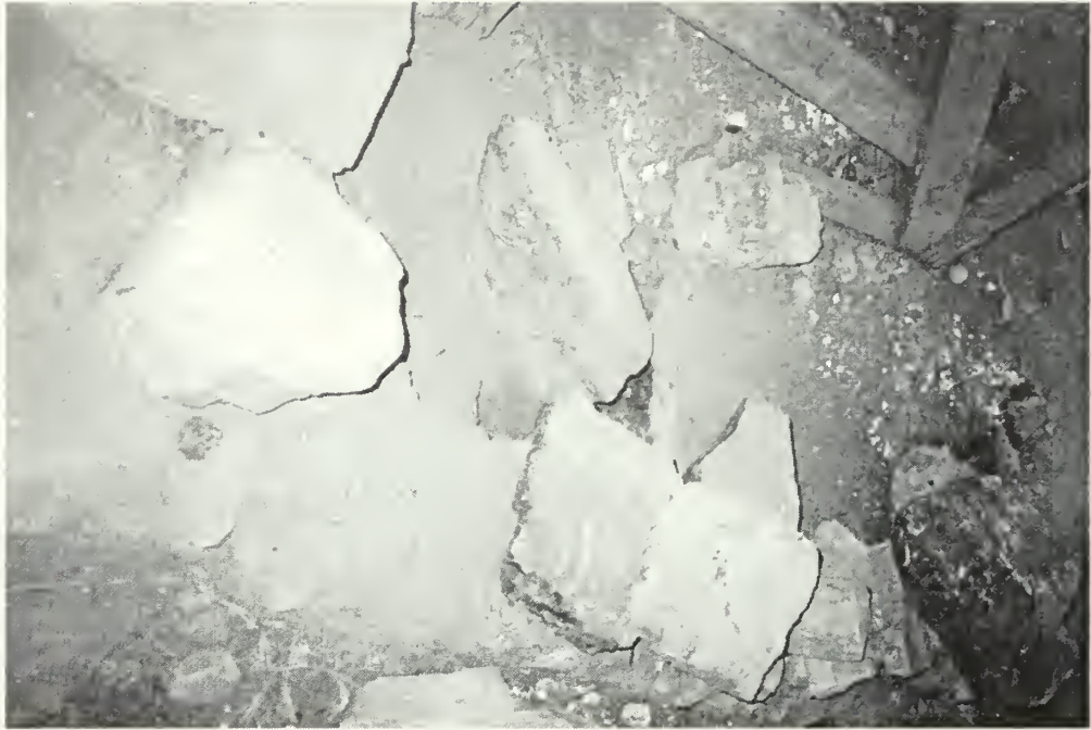
Figure 153: Concrete topping slab in dairy area in a state of disrepair due to rodent infestation.
