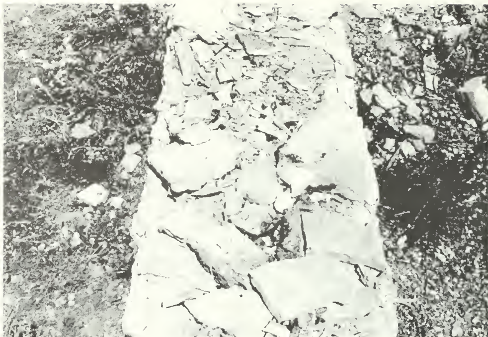
Figure 113: Condition of ruined Sherrick Barn foundation prior to stabilization. Note failure of limestone when exposed to extreme heat.
