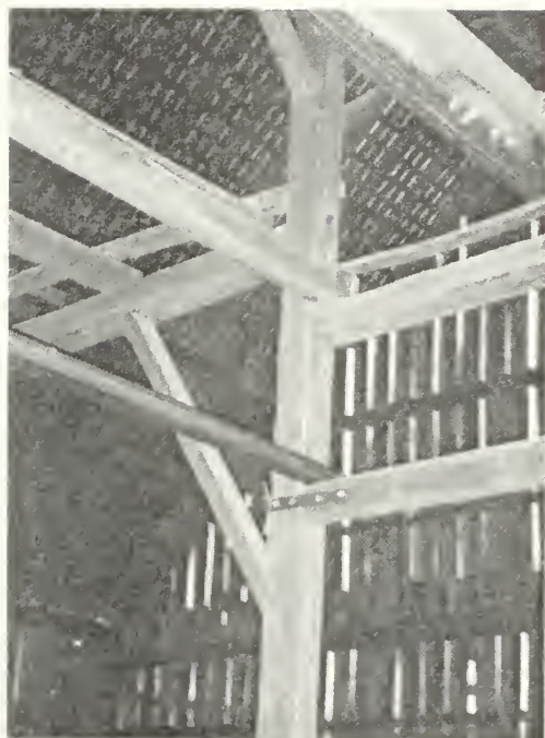
Figure 80: Steel beam in place to stabilize historic bents at the Piper Barn. Also note steel plate at connection of tie beam to post.
