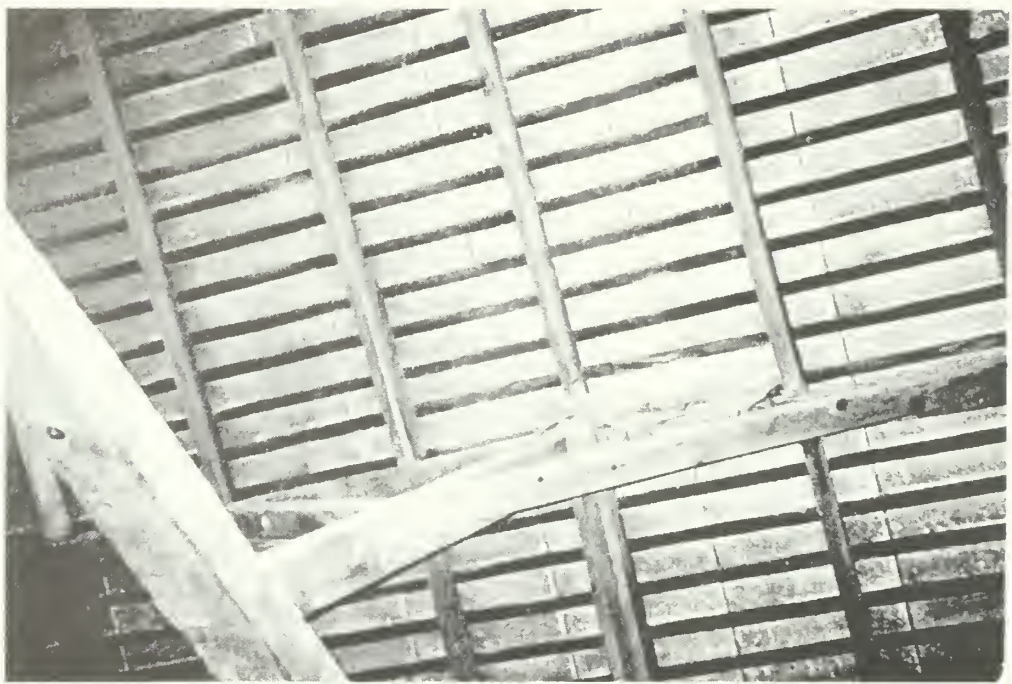
Figure 58: View of underside of galvanized-metal roof, rafters, and roof lath.
