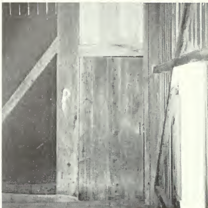
Figure 165: Entrance from the barn into the west granary. Note non-original infill panel above door.
