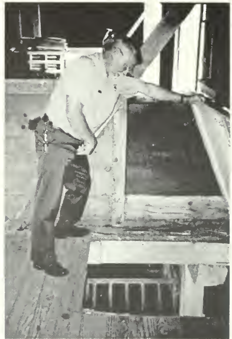
Figure 66: Hatch (hay bay) in the northeast mow used for throwing hay, straw, and grain to the animals stalls below
