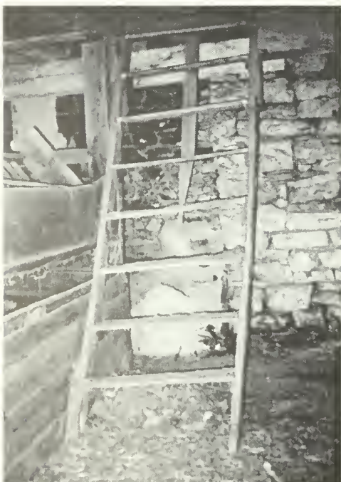
Figure 67: Open stair leading from a hatch in the southwest mow to the lower level.
