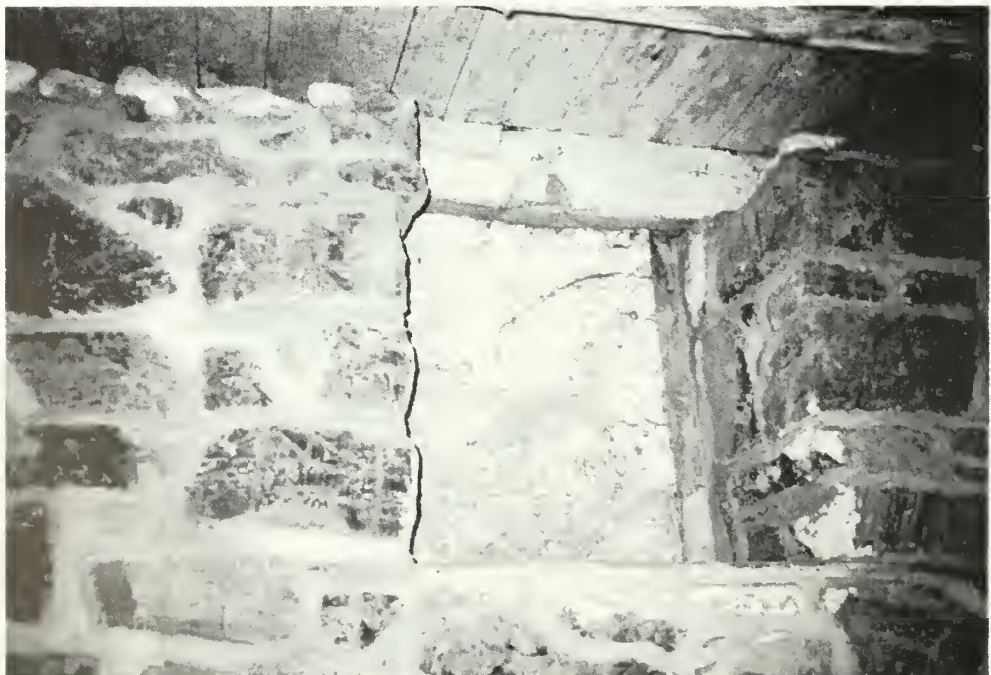
Figure 194: A typical opening (at the northeast elevation) covered over with sheet metal.
