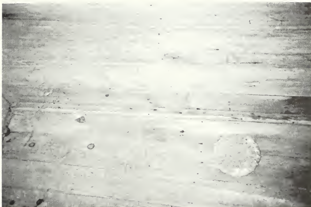
Figure 147: Original, wood threshing floor. Nonoriginal, galvanized patch covers a hole to the grain chute.
