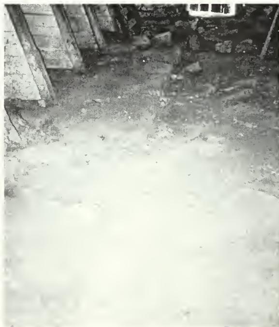
Figure 154: Deteriorated concrete topping slab in dairy area.
