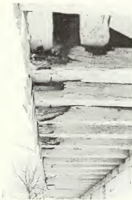
Figure 89: Deteriorated joist ends over forebay in 1985.
