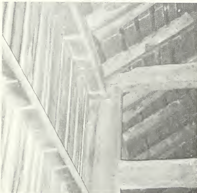
Figure 88: Rotting at tie beam connection to post (forebay side of interior).
