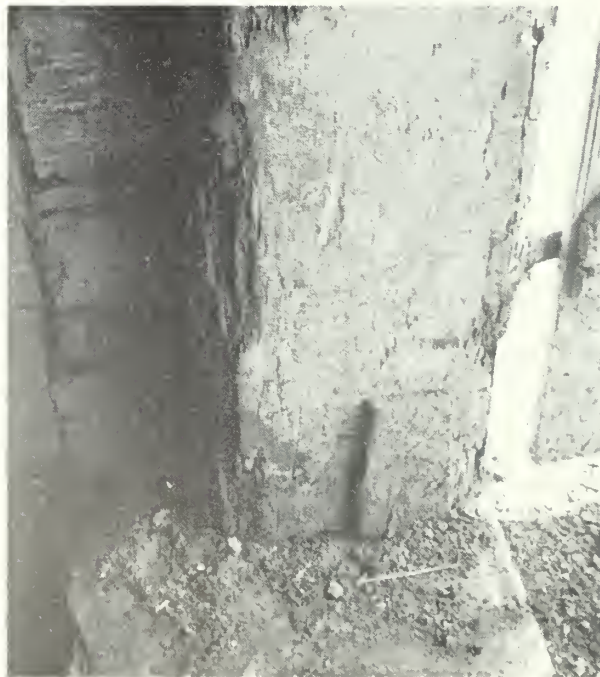
Figure 190: Wood frame of the double doors (southeast elevation). Note insect damage and splintering.
