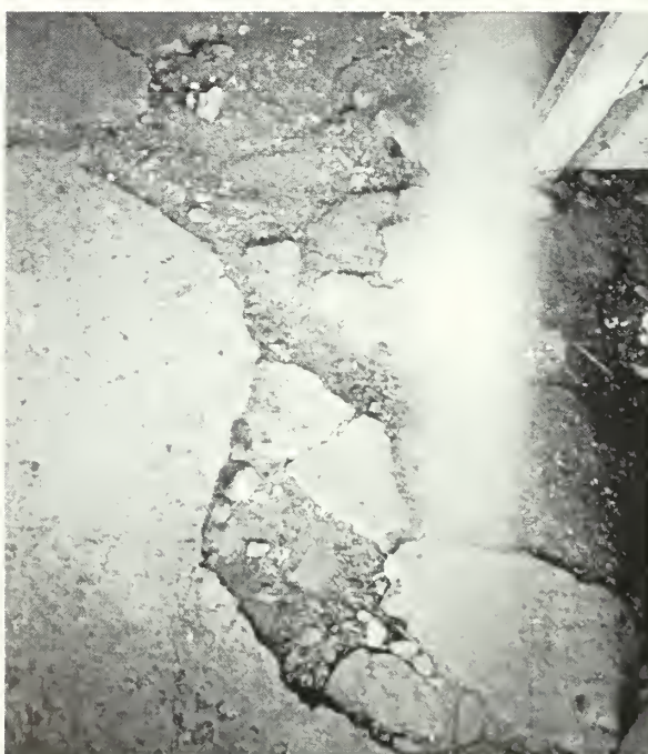
Figure 146: Deteriorated concrete topping slab at dairy area floor. Rodent infestation is the major cause of this damage.
