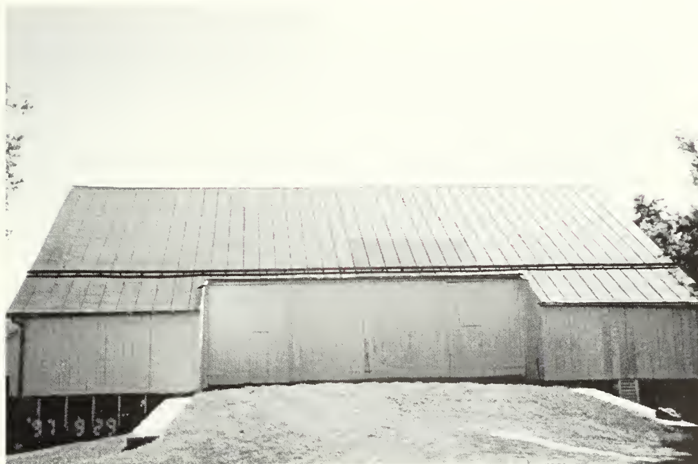
Figure 138: View of the barn's standing metal seam roof. To the knowledge of the park, the roof is still the 1936 version. No records indicate otherwise. Note the color of the roof is matte-brown.
