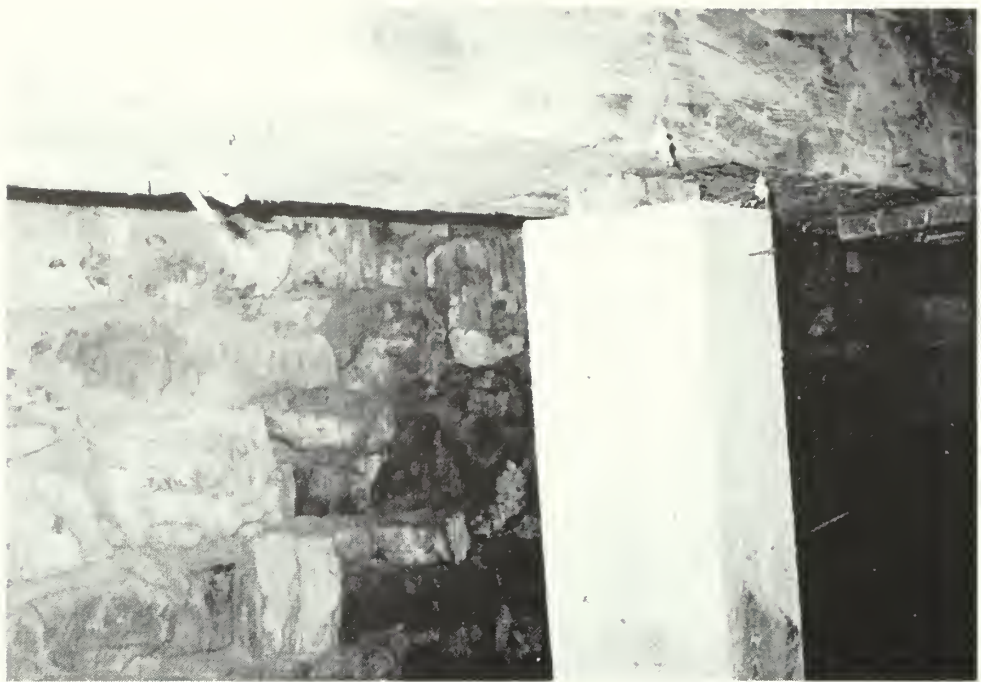
Figure 105: Separation of post from beam above.
