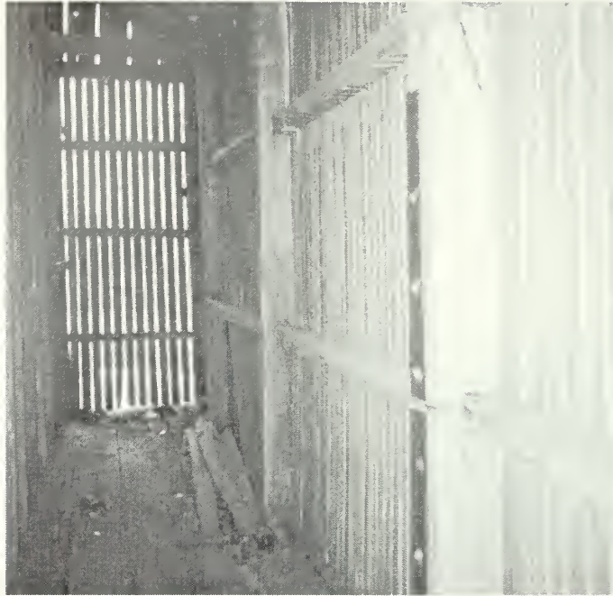
Figure 177: Interior of corn crib. Note vertical metal reinforcing.
