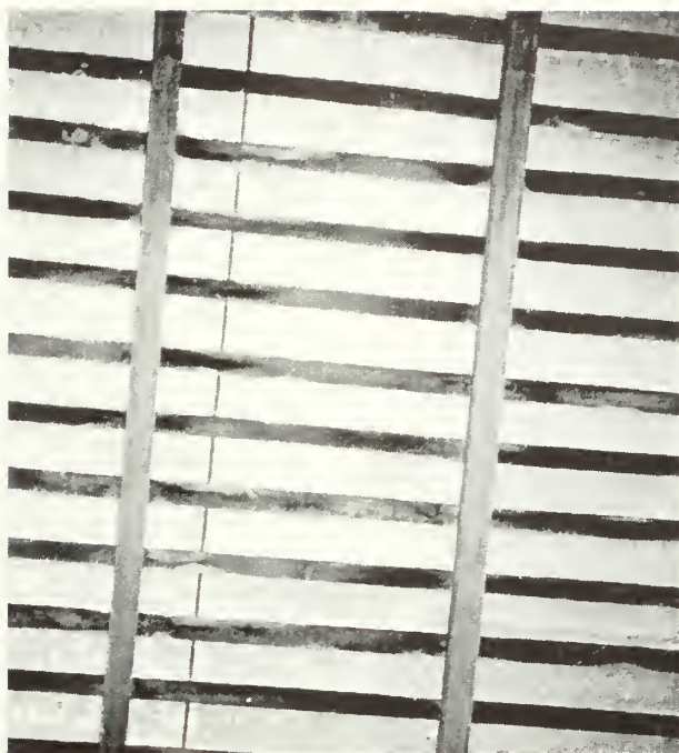
Figure 137: Roofing lath at underside of ceiling.
