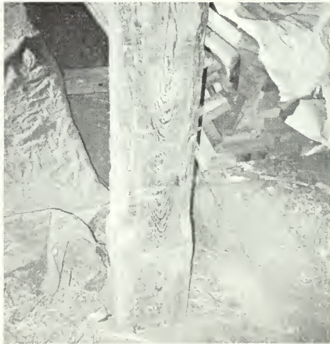
Figure 87: Base of chamfered post at central bent.
