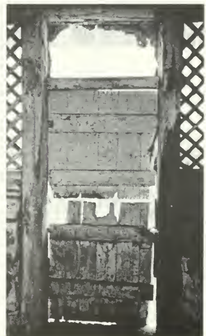
Figure 68: Typical split door leading from the ground level into the barnyard. Note lattice-work for ventilation.
