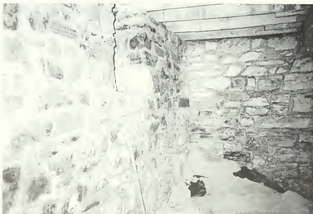
Figure 118: Western corner of foundation after repointing.
