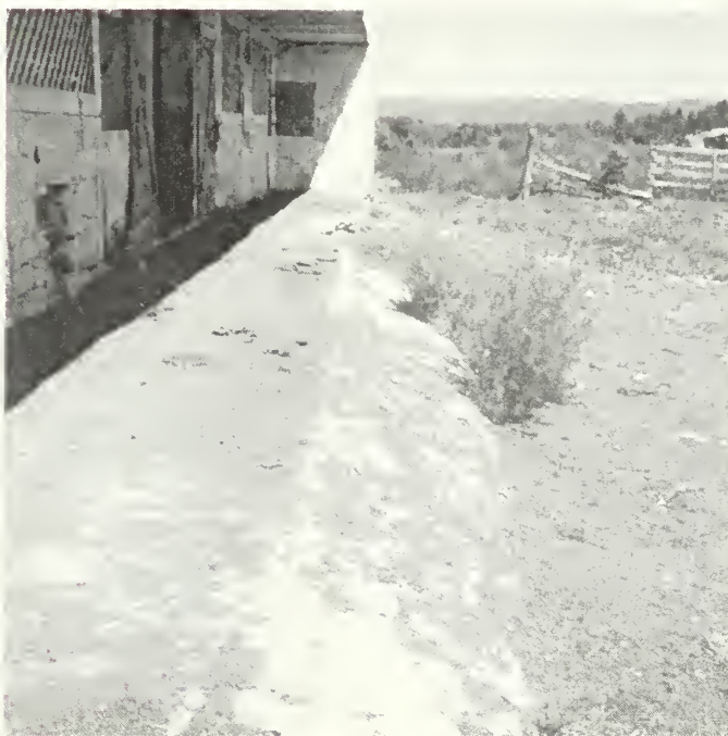
Figure 200: Concrete path that runs the length of the barn (front elevation). Note the significant drop from the path to the barnyard. This is due to animal traffic over the years.
