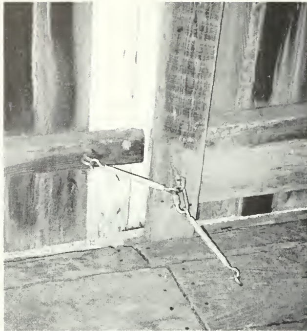
Figure 185: Modern hardware added by park maintenance to secure main wagon doors.
