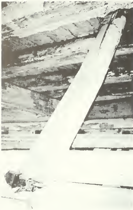
Figure 65: A nonhistoric, galvanized-metal grain pipe that runs from the threshing floor above, to the naimal stalls below.
