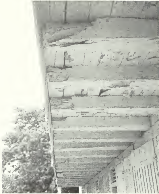
Figure 90: Deteriorated joist ends today. Paint helps to obscure some of the damage, but no repairs have been made.
