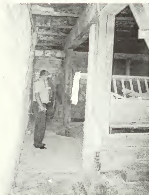
Figure 93: Bowing out of the northwest foundation wall. Note temporary jacks and posts relieving the load on the wall.
