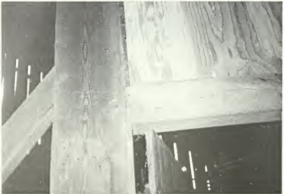
Figure 158: Mortise and tenon framing demonstrates that outsheds/granaries are original.
