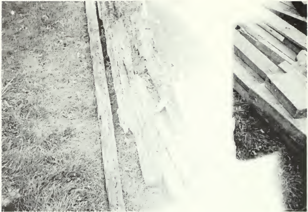
Figure 127: Portions of the rotted sill that was removed and replaced in 1990.
