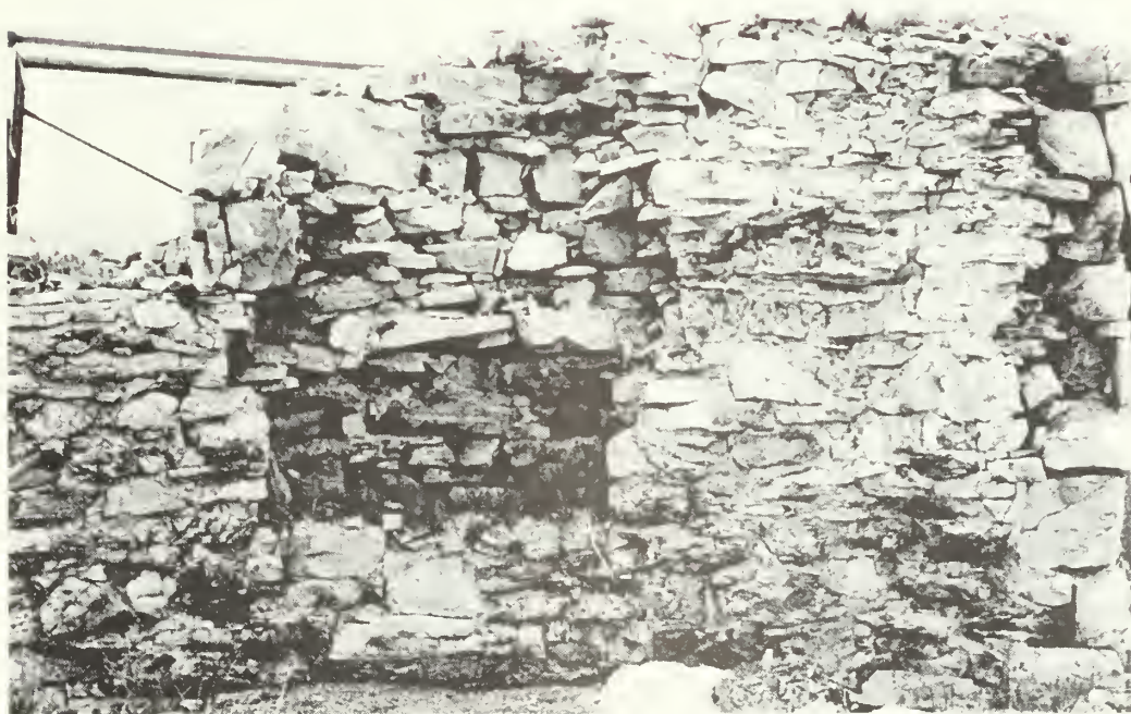
Figure 112: Condition of ruined Sherrick Barn foundation prior to stabilization.
