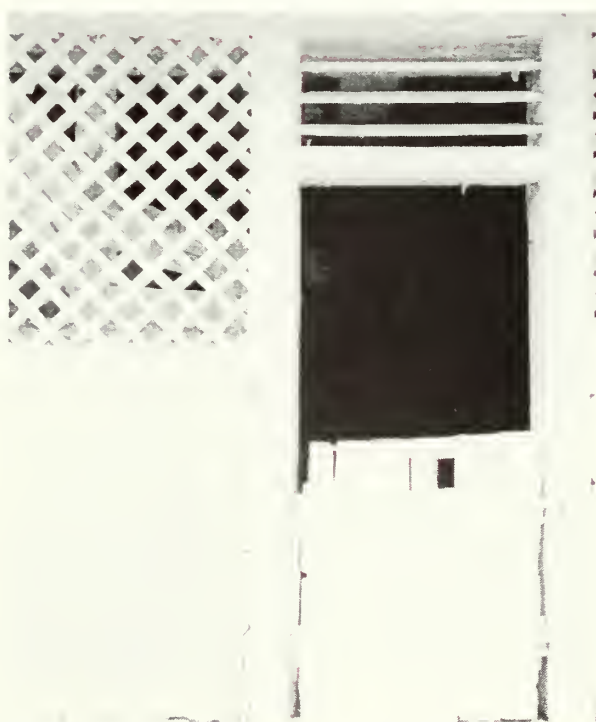
Figure 188: Top half of split door missing (southeast elevation).
