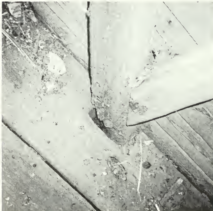
Figure 178: Deterioration where vertical post and diagonal brace meet floor (at interior of corn crib).
