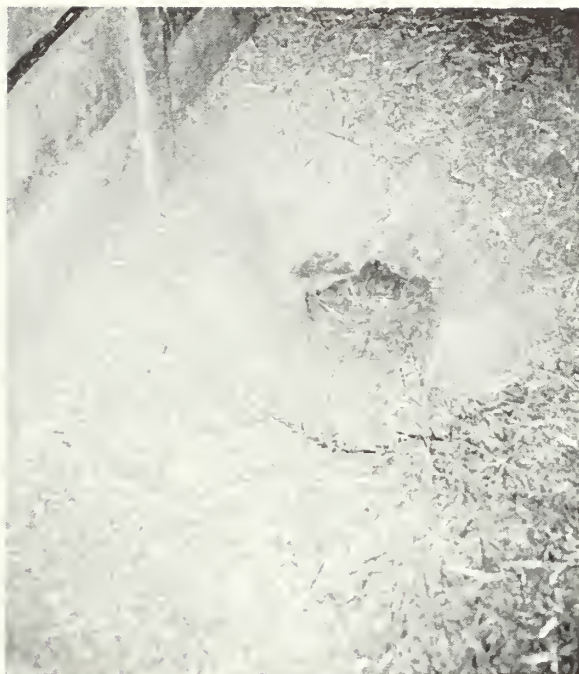
Figure 155: Damage caused by burrowing ground hogs.
