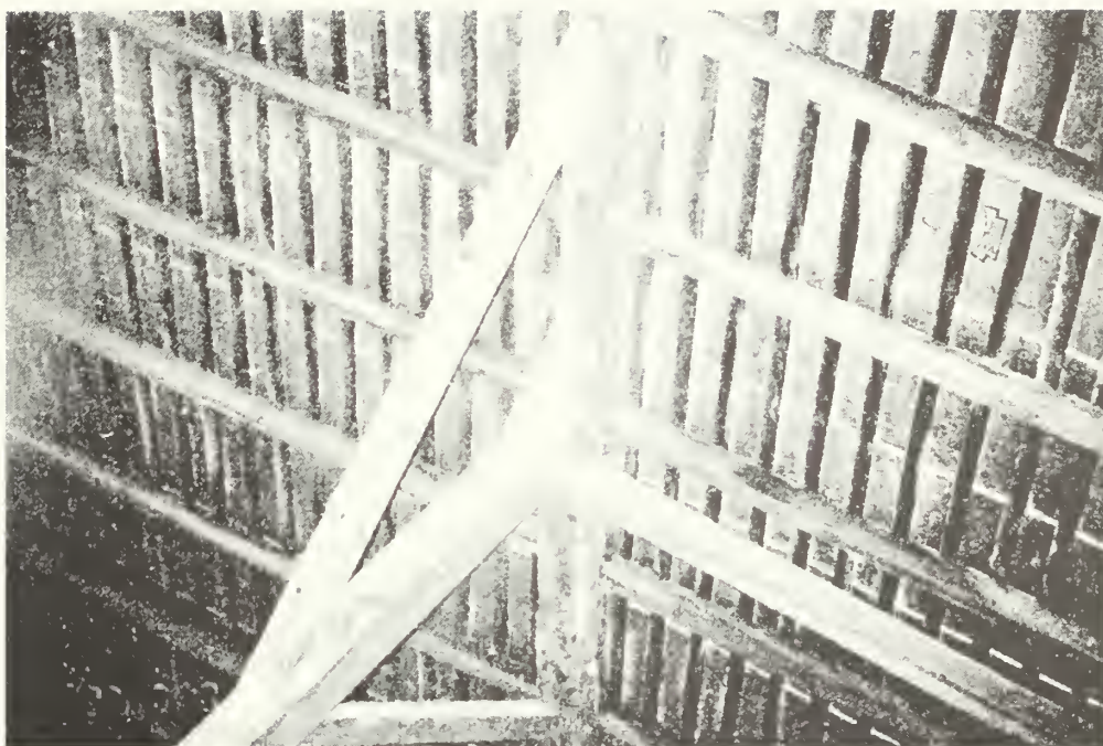
Figure 84: Rotted connection of angled purlin post (diagonal brace) to roof purlin (forebay side of interior).
