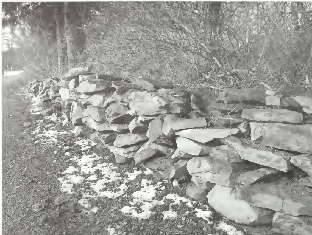
Figure 7.20. Typical stone wall at Val-Kill. This is an informal dry-laid wall created from agricultural activities (OCLP, 2003).
