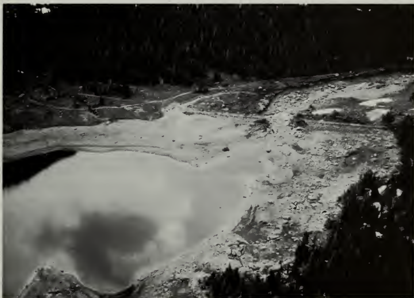
Fig. 3. Aerial view of Lawn Lake about 1 week after the dam failure, showing water still remaining in the natural depression of the original lake (from Jarrett and Costa 1986).
