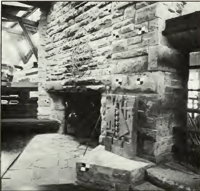
Targets placed on the hearth of Taliesin, Spring Green, Sauk County, Wisconsin, as part of the demonstration of convergent photogrammetry by Dana L. Lockett, HABS Architect, and John A. Burns, AIA, HABS/HAER Deputy Chief. Photo by: Dana L. Lockett, 1993.
