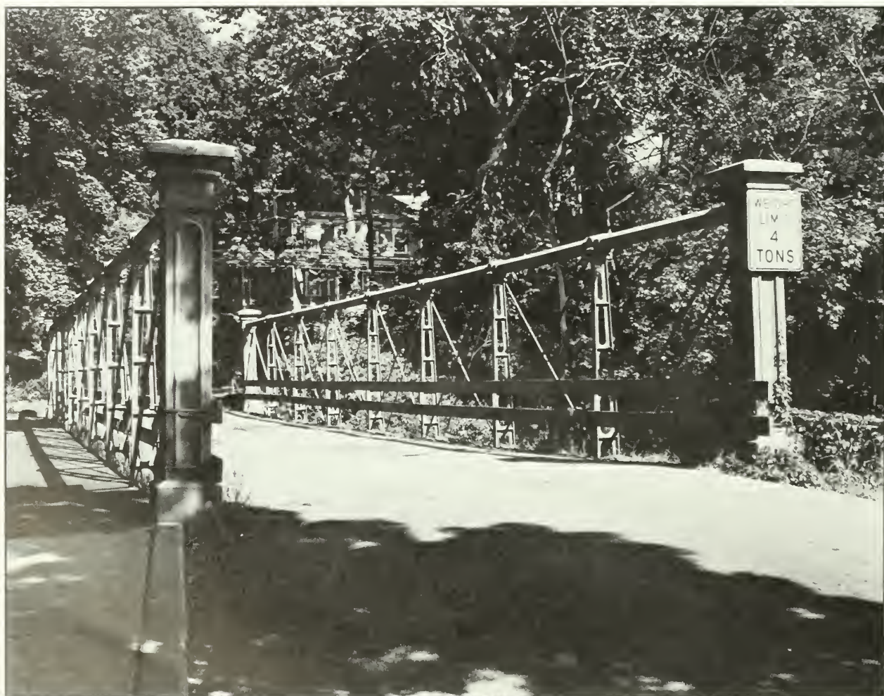
Glen Gardner Bridge, Glen Gardner, Hunterdon County, New Jersey (HAER No. NJ-92), is an example of a prefabricated truss bridge that HAER's Historic Bridge Program has recorded. HAER Photograph by: Joseph Elliott, 1991.
