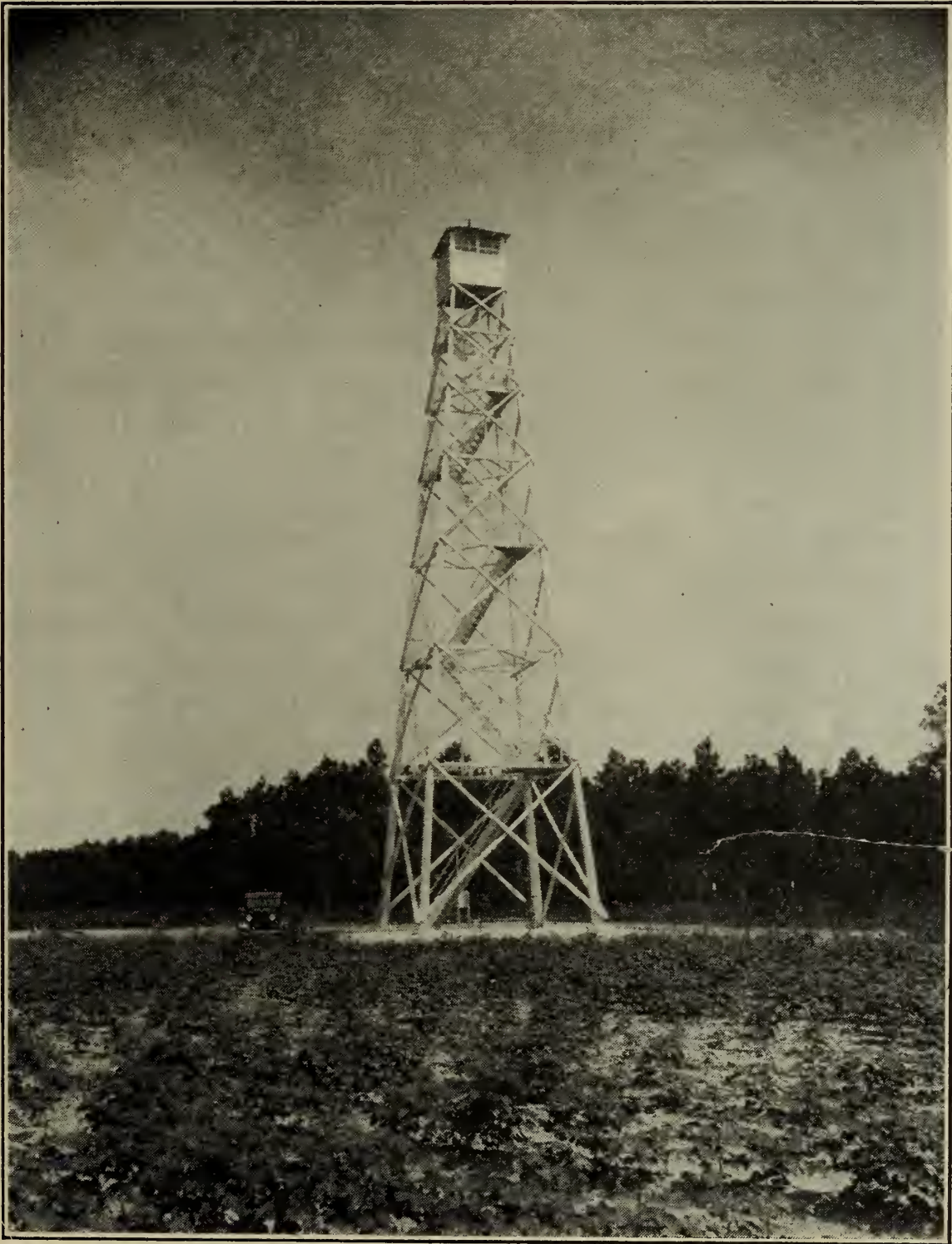
90 Ft. Wood (Cypress Pole) Tower—Sumter County Note: Secondary tower used during periods of low visibility.
