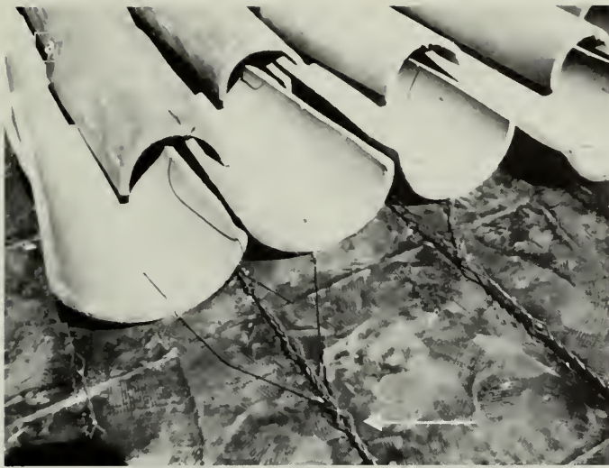
Figure 13 (a-b). These custom-made tapered mission tiles are being attached to the roof using a special system. This consists of twisted 10-gauge brass or copper wires that run up the roof slope through a new treated roof ridge, and down the other side of the roof. These twisted wires are placed about 12" (30.5cm) apart, and diamond shapes are twisted into them every 6" (15cm). The vertical wires are secured with 10-gauge copper or brass anchors approximately every 4' (1.22m) on center depending on the roof slope. Although these tiles would have originally been laid in mud mortar, this method of attachment is particularly successful in seismic areas. The random placement of the tiles accurately replicates the pattern traditionally used on the early missions. Photos: Gil Sánchez, FAIA.
