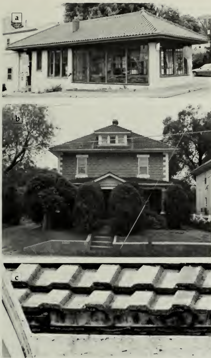
Fig. 7. (a) Metal “tile” roofs of galvanized steel closely resemble the clay tiles they mimic. Often painted to look like terra cotta, their identity can sometimes be revealed by peeling paint or dented “tiles.” (b-c) Concrete roofing tiles are generally thicker than clay tiles, and tend to fade and lose their color. Photos: (a-b) Anne Grimmer, (c) National Park Service Files.
