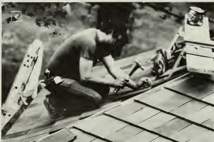
Figure 12. When constructed in Frankfort, Kentucky, in 1900, the Colonial Revival-style Berry Hill Mansion, and its 1912 Music Room addition were both roofed with "Imperial" tiles manufactured by Ludowici-Celadon (a). In 1992 the entire roof was replaced because of deterioration and surface spalling of many of the tiles (b). It was not possible to reproduce the original tiles due to budget limitations, thus Ludowici-Celadon's stock "Classic Interlocking" Shingle tiles were selected as replacements which could provide a close, if not exact, match. After tearing off and removing the old tiles, 30 lb. roofing felt was laid over the existing wood sheathing, new lead gutters and valleys were installed, and 90 lb. roll roofing was laid, on which the new tiles were laid. Although most of the field tiles were simply attached by 2 nails to the substrate (c), many of the tiles that had to be cut to fit hips, valleys and dormers were left with only one hole, and had to be wired and then nailed in place (d-e). The exact color and glaze of the original tiles also could not be duplicated because the coloring material is no longer available; however, the new hipped roof terminus for the Music Room roof was custom-made and the replacement field tiles are very similar to the originals (f). The original ridge tiles were designed to "nest" and fit perfectly over the field tiles beneath them whereas the new ridge tiles simply overlap one another, but this is barely perceptible when viewed from the ground. Photos: Edwin C. Krebs, AIA.
