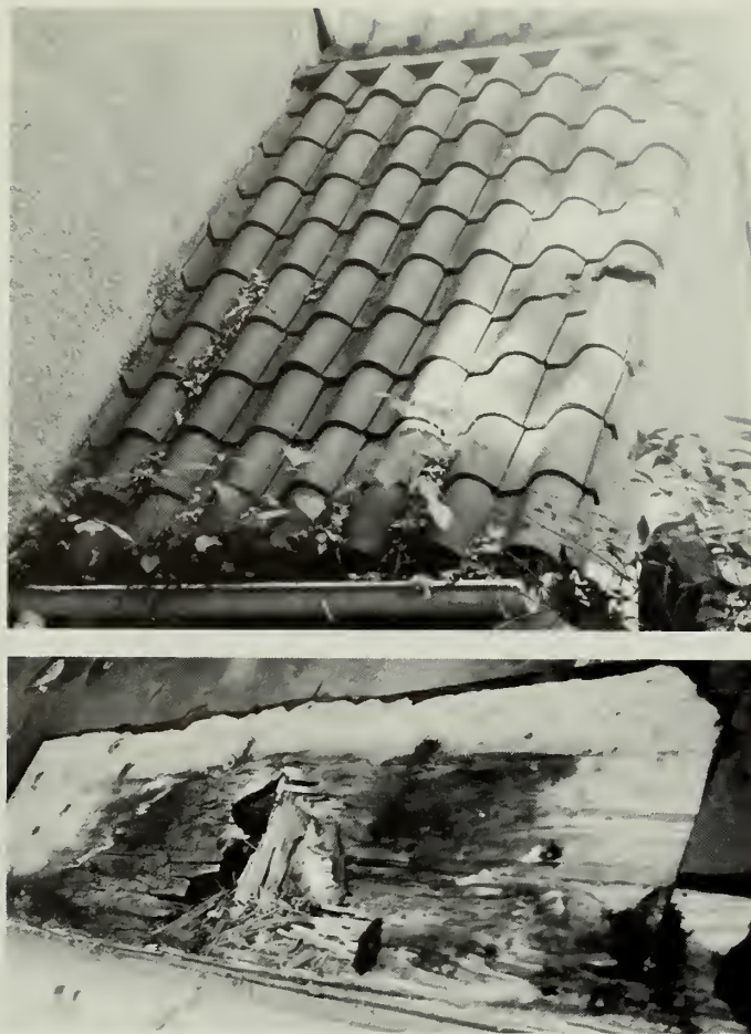
Figure 15. (a) A regular cleaning schedule would have eliminated the plant growth and leaf build-up in this gutter, which, if not removed, will result in serious damage to roof sheathing and structure (b). Photos: (a) Paul K. Williams, and (b) Walter S. Marder. AIA.
