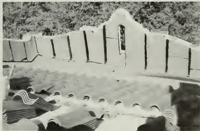
Fig. 14. The Spanish or "S" tiles used to re-roof the Mission Revival style Holy Cross Episcopal Church in Sanford, Florida, have corrugated projections or "teeth" on the underside of the flat portion of each tile which adhere to the cement mortar holding them to the roof sheathing. Photo: Walter S. Marder, AIA.
