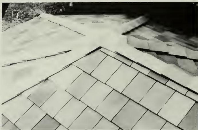
Figure 12. When constructed in Frankfort, Kentucky, in 1900, the Colonial Revival-style Berry Hill Mansion, and its 1912 Music Room addition were both roofed with "Imperial" tiles manufactured by Ludowici-Celadon (a). In 1992 the entire roof was replaced because of deterioration and surface spalling of many of the tiles (b). It was not possible to reproduce the original tiles due to budget limitations, thus Ludowici-Celadon's stock "Classic Interlocking" Shingle tiles were selected as replacements which could provide a close, if not exact, match. After tearing off and removing the old tiles, 30 lb. roofing felt was laid over the existing wood sheathing, new lead gutters and valleys were installed, and 90 lb. roll roofing was laid, on which the new tiles were laid. Although most of the field tiles were simply attached by 2 nails to the substrate (c), many of the tiles that had to be cut to fit hips, valleys and dormers were left with only one hole, and had to be wired and then nailed in place (d-e). The exact color and glaze of the original tiles also could not be duplicated because the coloring material is no longer available; however, the new hipped roof terminus for the Music Room roof was custom-made and the replacement field tiles are very similar to the originals (f). The original ridge tiles were designed to "nest" and fit perfectly over the field tiles beneath them whereas the new ridge tiles simply overlap one another, but this is barely perceptible when viewed from the ground. Photos: Edwin C. Krebs, AIA.
