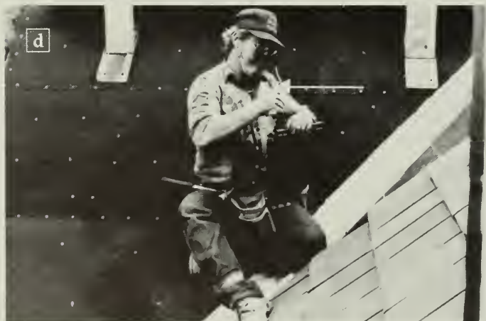
Figure 12. When constructed in Frankfort, Kentucky, in 1900, the Colonial Revival-style Berry Hill Mansion, and its 1912 Music Room addition were both roofed with "Imperial" tiles manufactured by Ludowici-Celadon (a). In 1992 the entire roof was replaced because of deterioration and surface spalling of many of the tiles (b). It was not possible to reproduce the original tiles due to budget limitations, thus Ludowici-Celadon's stock "Classic Interlocking" Shingle tiles were selected as replacements which could provide a close, if not exact, match. After tearing off and removing the old tiles, 30 lb. roofing felt was laid over the existing wood sheathing, new lead gutters and valleys were installed, and 90 lb. roll roofing was laid, on which the new tiles were laid. Although most of the field tiles were simply attached by 2 nails to the substrate (c), many of the tiles that had to be cut to fit hips, valleys and dormers were left with only one hole, and had to be wired and then nailed in place (d-e). The exact color and glaze of the original tiles also could not be duplicated because the coloring material is no longer available; however, the new hipped roof terminus for the Music Room roof was custom-made and the replacement field tiles are very similar to the originals (f). The original ridge tiles were designed to "nest" and fit perfectly over the field tiles beneath them whereas the new ridge tiles simply overlap one another, but this is barely perceptible when viewed from the ground. Photos: Edwin C. Krebs, AIA.
