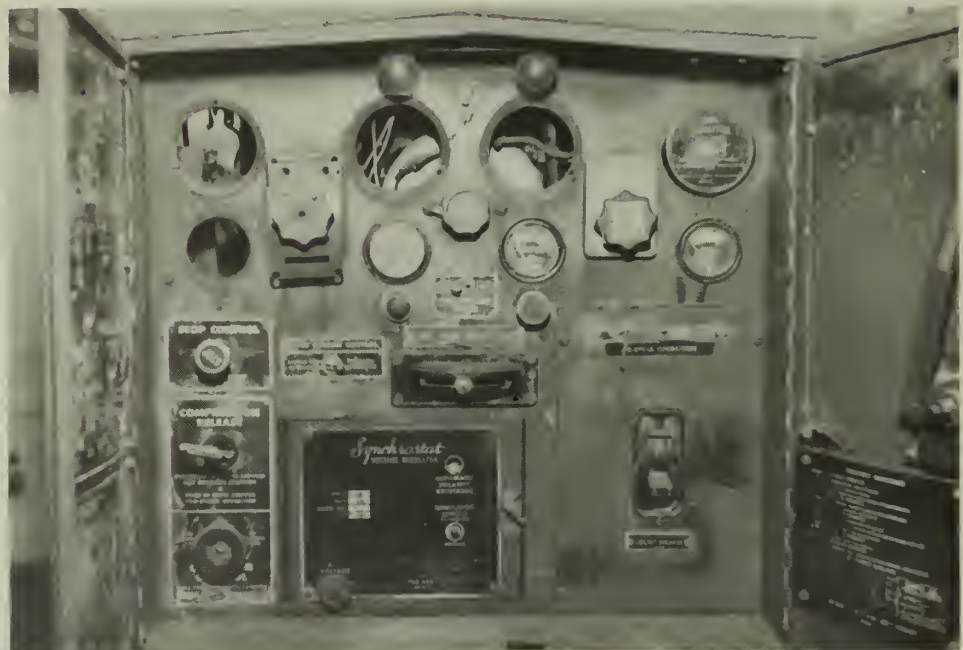
41. Room 104- Synchrostat voltage regular, inside front doors (#8)
