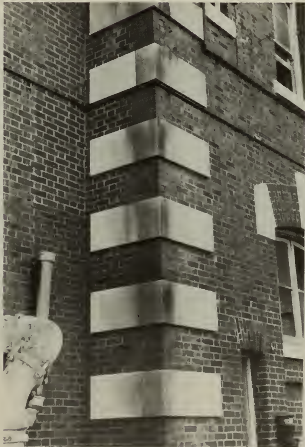
30. Copper staining at quoins, south pavilion, west elevation.
