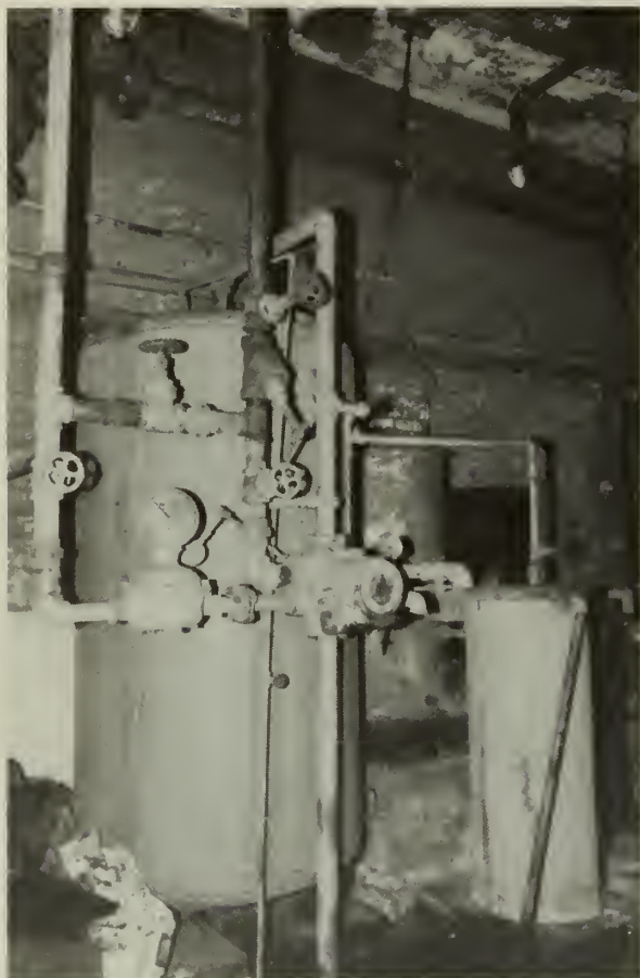
63. Room 106- water softener, west wall. 64. Room 106- west wall. "Permutit"- brine rinse.
