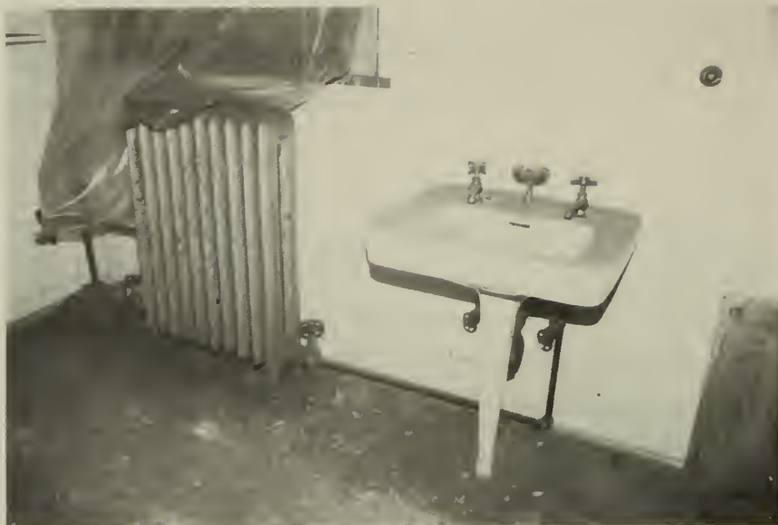
1. Room 208, sectional radiator and square pedestal sink.
