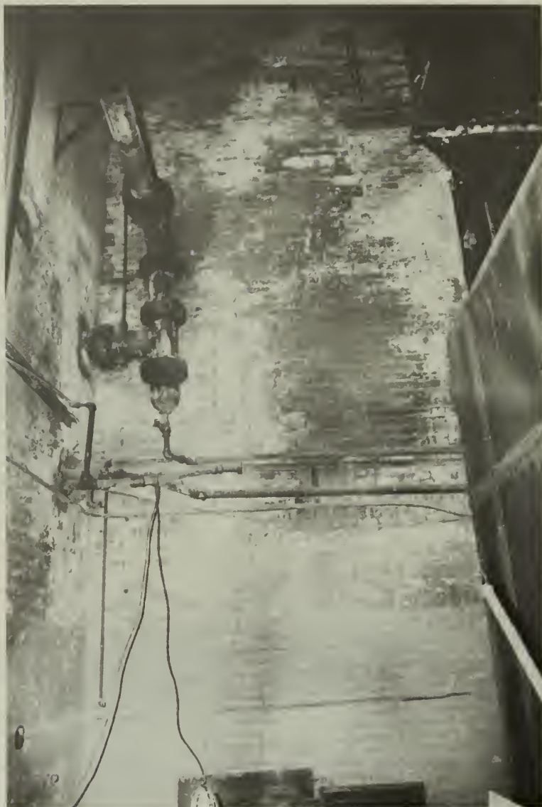
10. Typical example of cracking of main stack lower shaft
