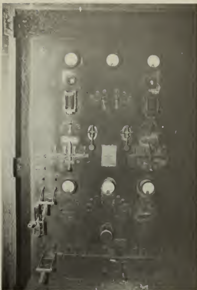
47. Faraday alarm system-inside panel (#10)
