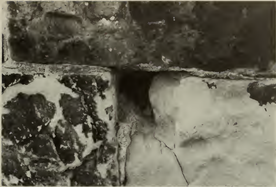
29. Loss of material, granite base, west elevation.
