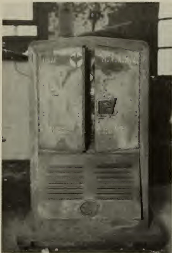
42. Synchrostat voltage regulator- front doors- (#8)
