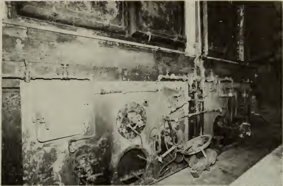
8. Room 105, boiler #4 and 5 (1917). Converted from coal to oil-fired in 1932 and further altered in 1947. Steps down to "firing trench" in front
