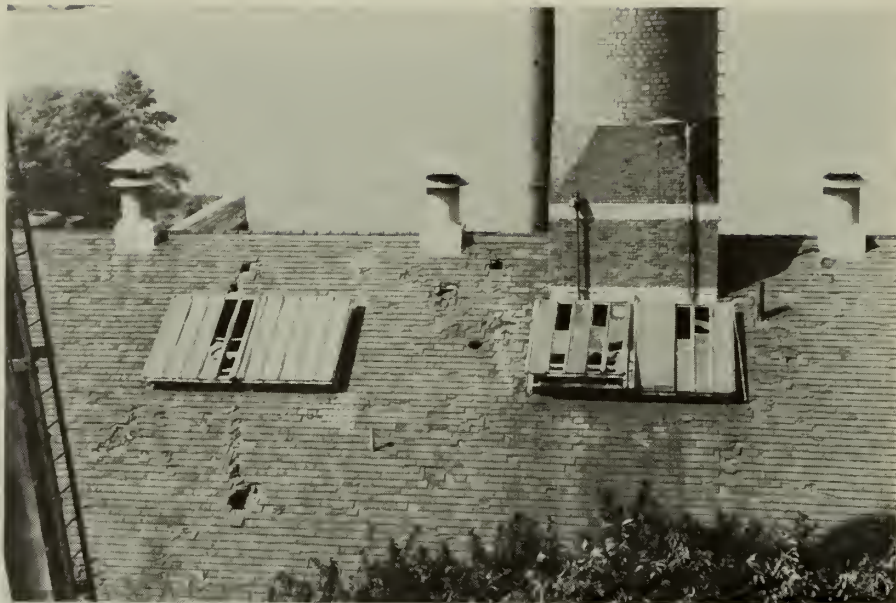
35. East side of roof; holes and broken tiles, view west.
