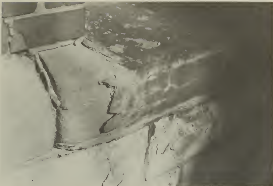
25. Exfoliation, bluestone water table, east elevation.
