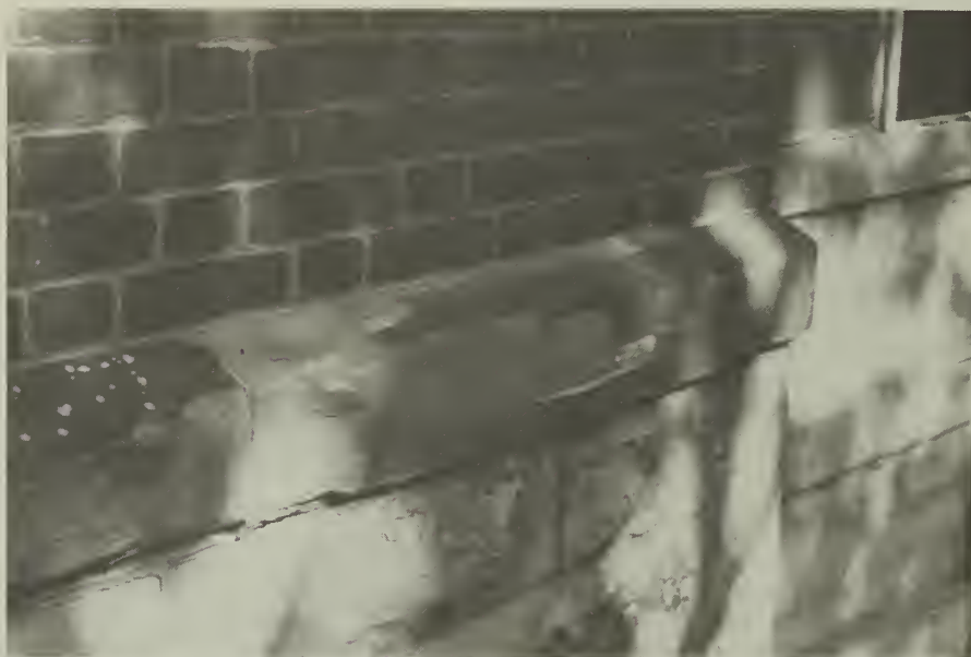
24. Exfoliation, bluestone water table, east elevation.
