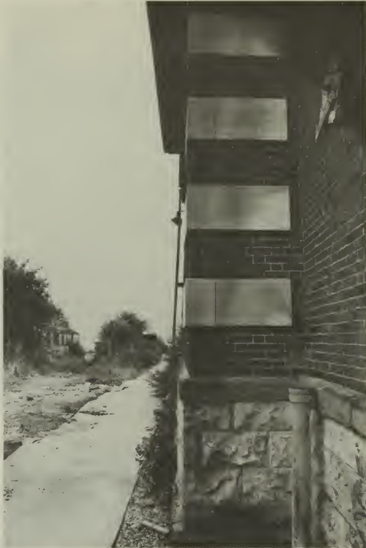
5. View of the bulging of the exterior bearing wall. As photograph 4
