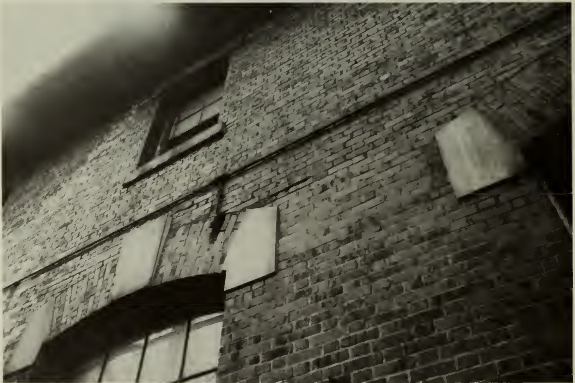
3. Typical example of cracking of exterior bearing walls
