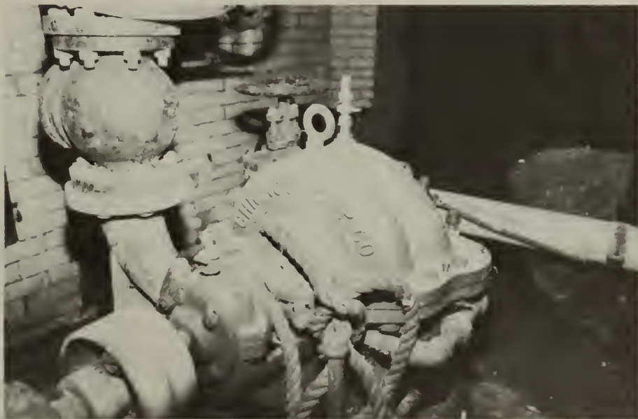
17. Room 105, boiler feed pump, "Chicago Pump Co." Section of piping located behind (east) of above photo.
