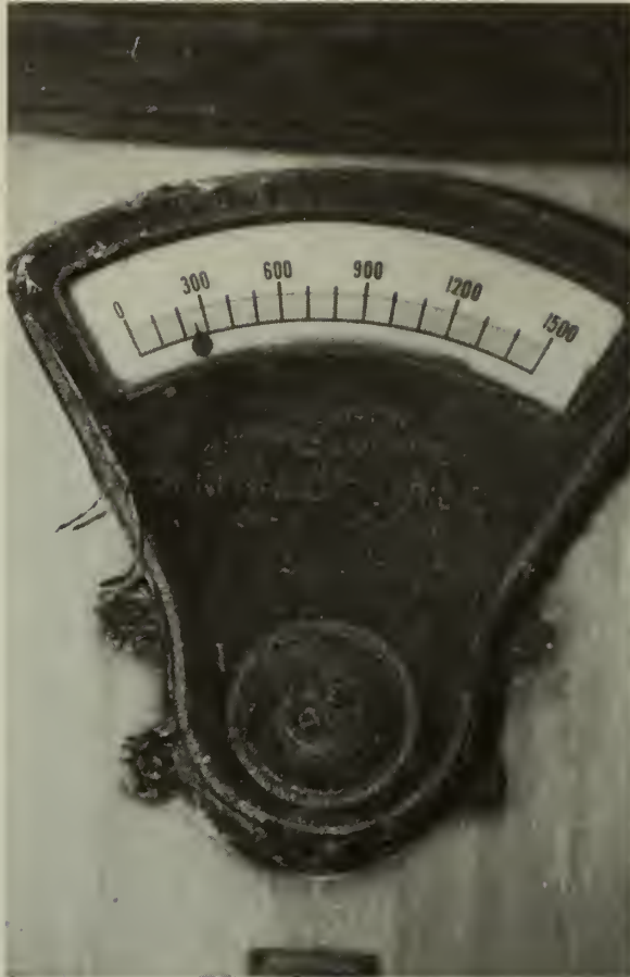
23. Room 104- Top surviving panel of marble switchboard, "Thomson Astatic Ammeter" General Electric Co.
