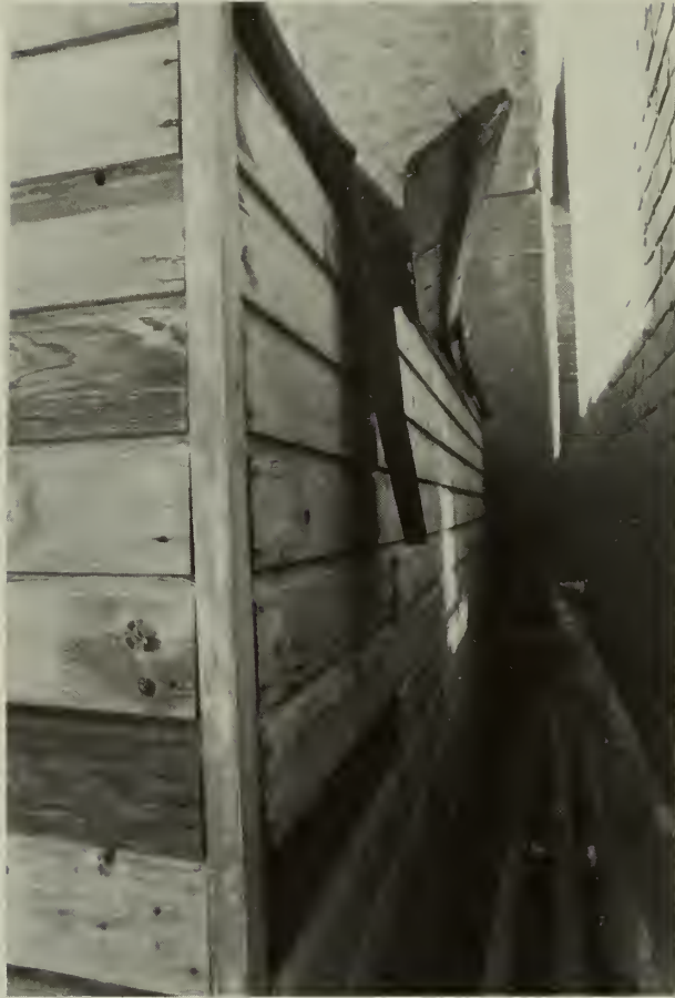
39. Wood siding separating, west elevation of shed, view south.
