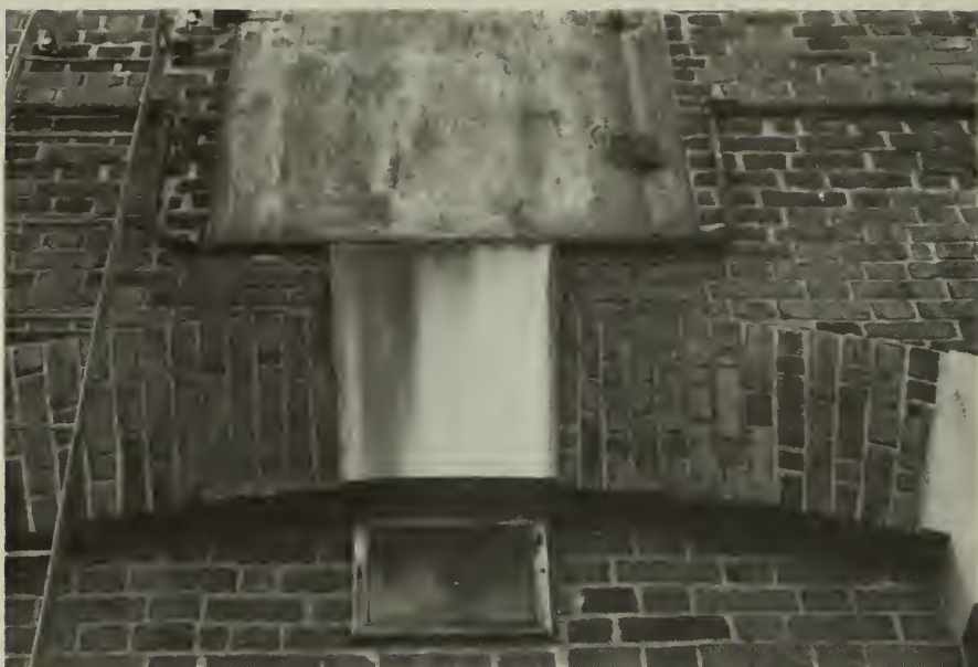
31. Iron staining at keystone, west elevation.
