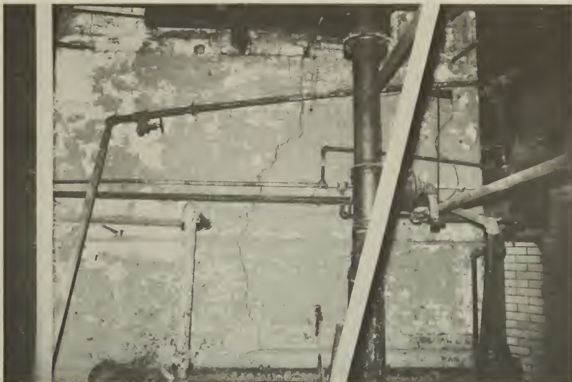
11. View showing severe cracking of the lower shaft of the main stack
