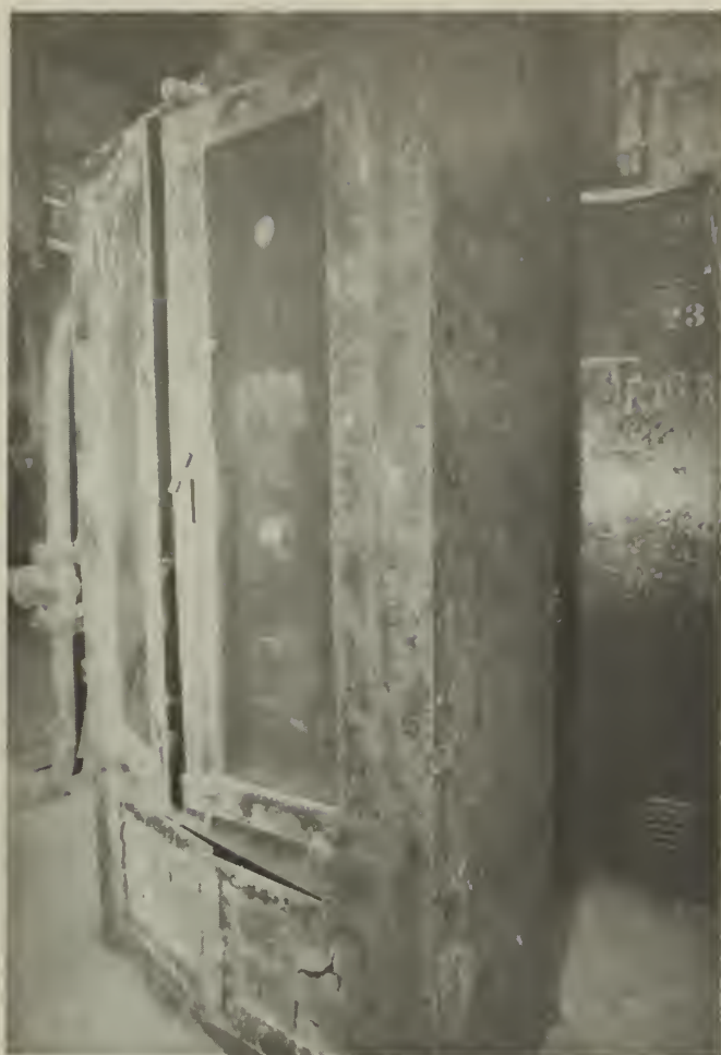
46. Faraday 28-station fire alarm panel (#10)
