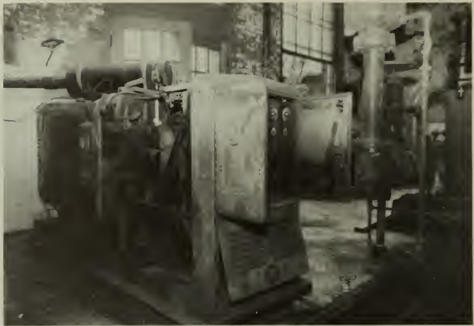
40. Room 104- Synchrostat Voltage Regulator (#8)
