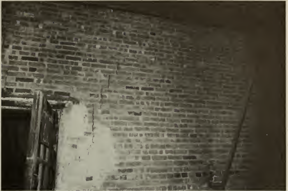
8. View showing cracking of interior bearing walls. As photograph 7
