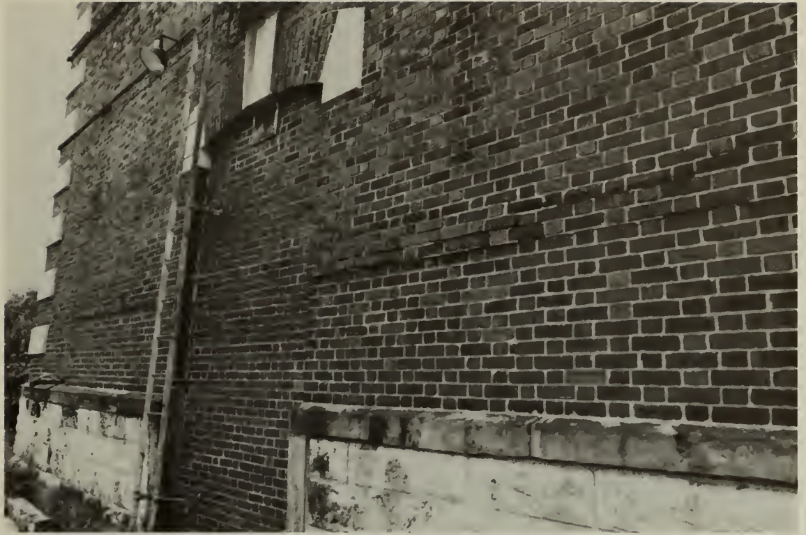
4. View showing bulging and cracking of exterior bearing walls in the area of the northwest corner of the oil tank room due to corrosion of embedded angles
