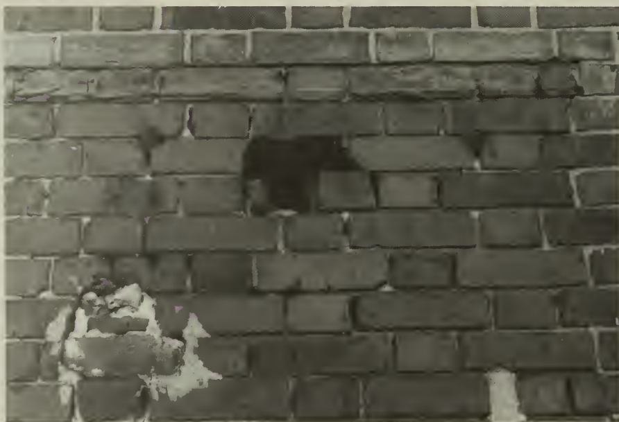
28. Loss of brick, deteriorating mortar, spalling, and patching, west elevation.
