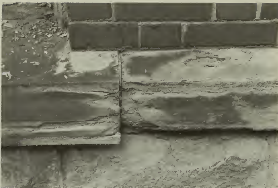
23. Exfoliation, bluestone water table, east elevation.
