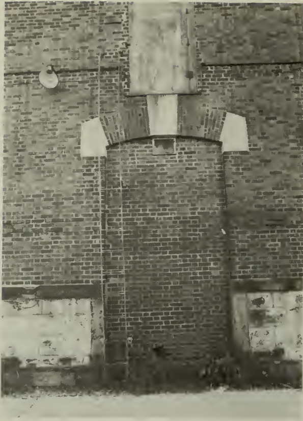
19. North pavilion entrance filled in with brick, west elevation.
