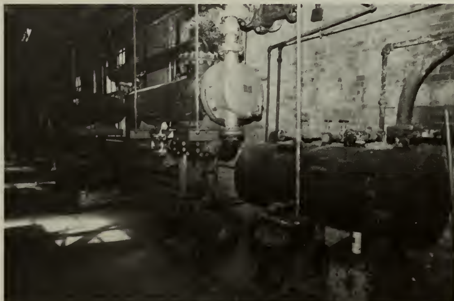
54. Room 106- east wall, two Warren tanks-ceiling suspended, at left, (#9), at right- "Machine Works" barrel, (#11).
