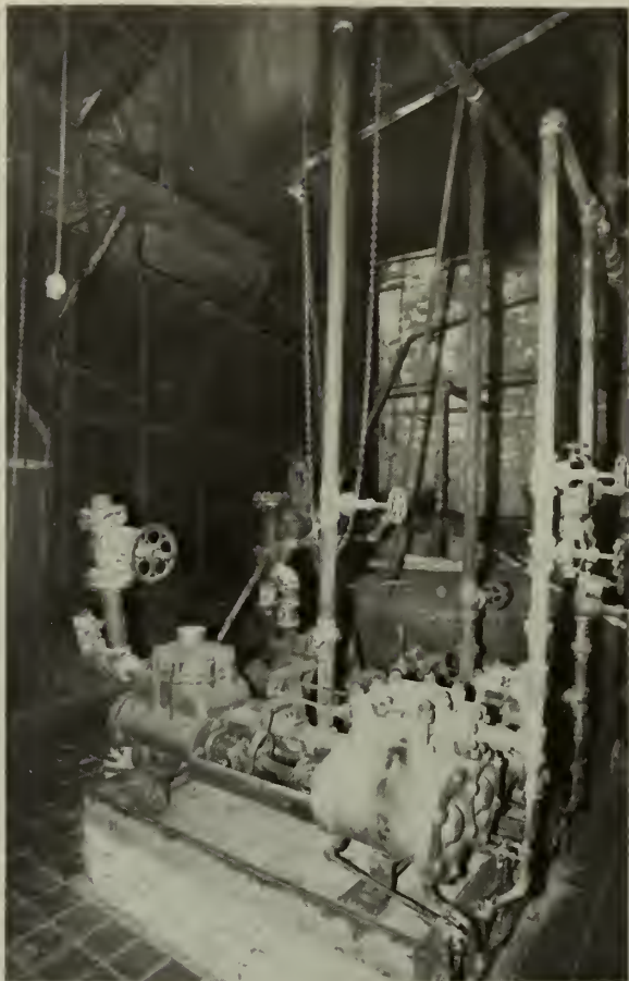
14. Room 105, steam-driven pumps in foreground and drip tank and brick base of stack in background.
