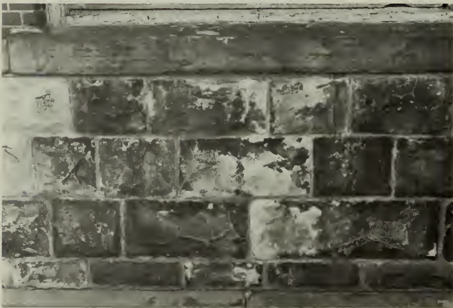
32. Black crust at base, west elevation.
