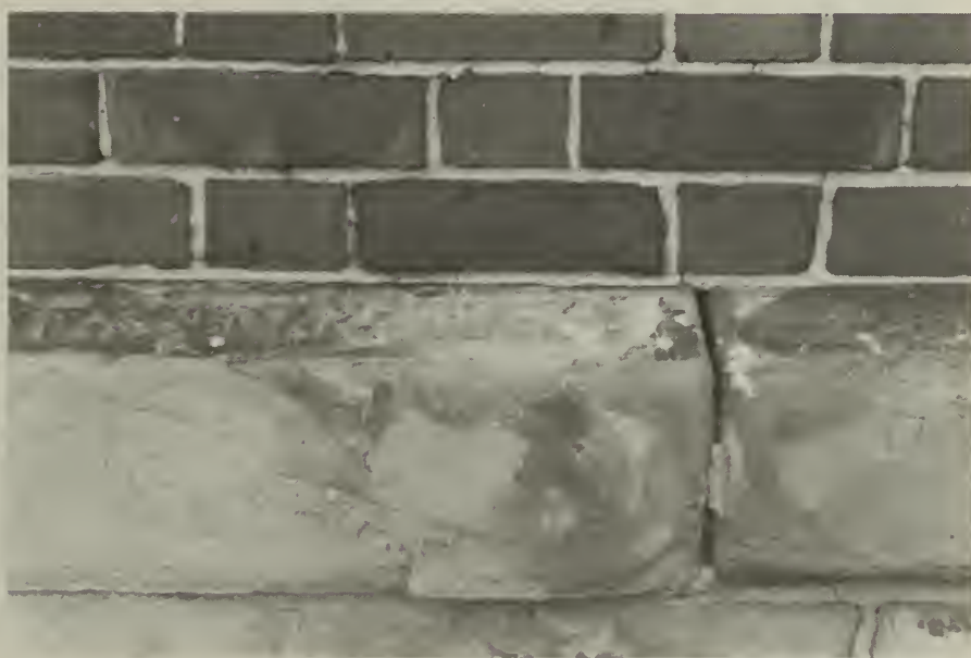
26. Exfoliation, bluestone water table, west elevation.
