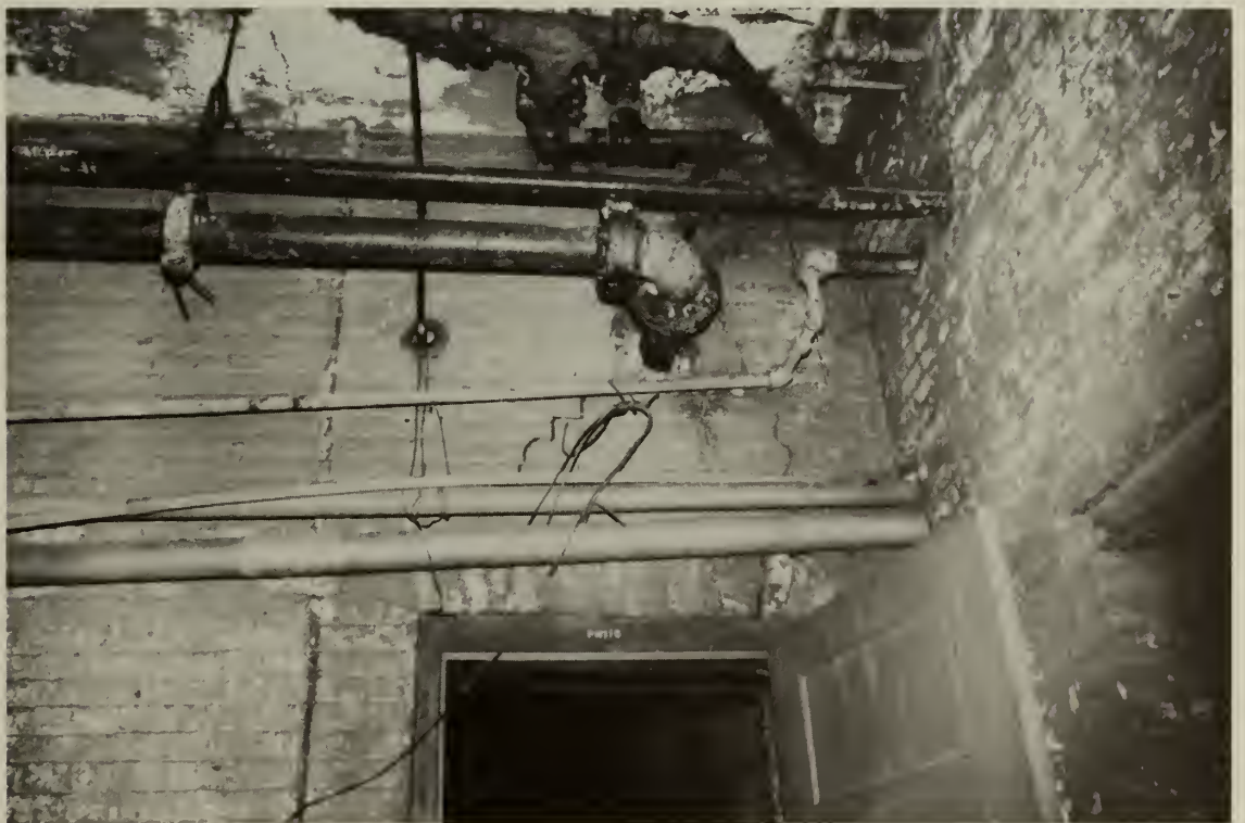
9. View showing cracking of interior bearing walls. As photograph 7
