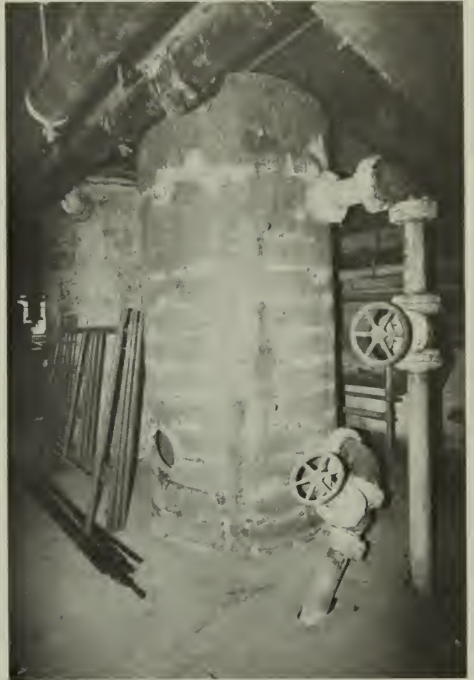
55. Room 106- cold water condensation return tank (#2) 56. Room 106- salt water tank (#3)
