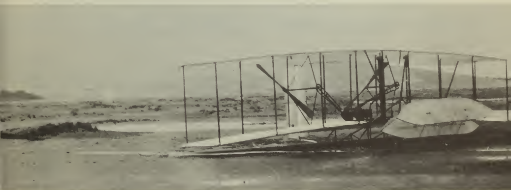
Close-up of 1903 machine at end of last flight, rudder frame broken in landing. Courtesy, Smithsonian Institution.
