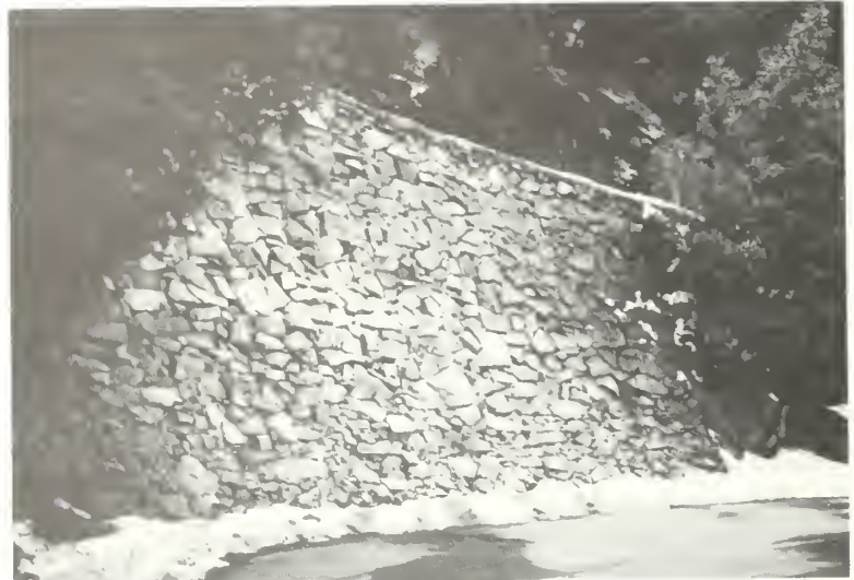
Typical CCC rubble dry-laid walls in the switchback and big tree areas
