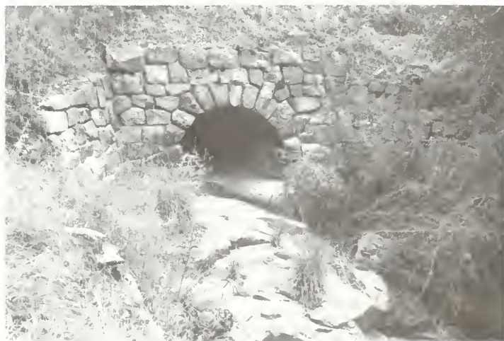
Another CCC culvert headwall today, after 50 years.
