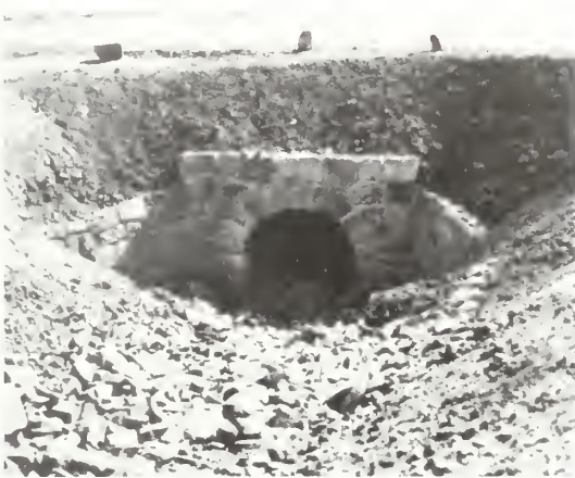
Historic photo of culvert headwall constructed by the CCC.
