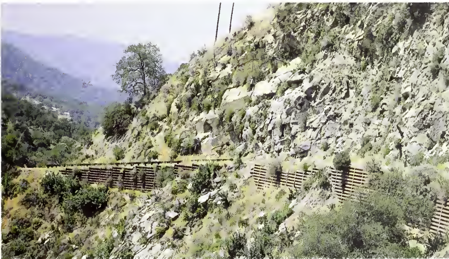
Weathering-steel bin wall in Kaweah Canyon area
