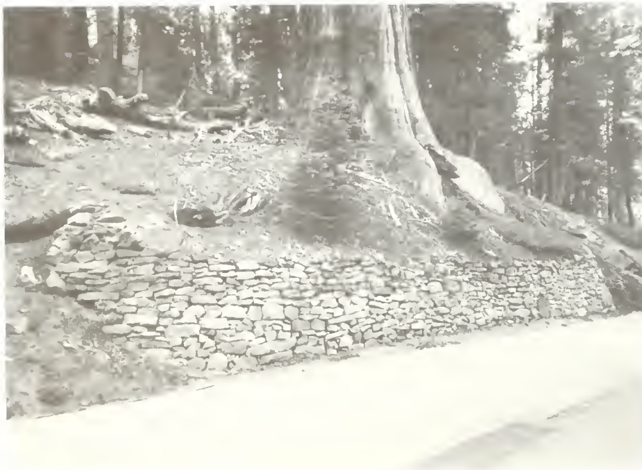
Typical CCC rubble dry-laid walls in the switchback and big tree areas
