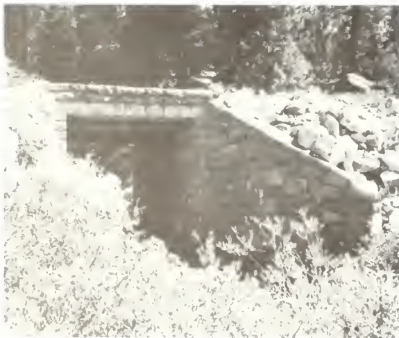
Box culvert with rock veneer wing walls.
