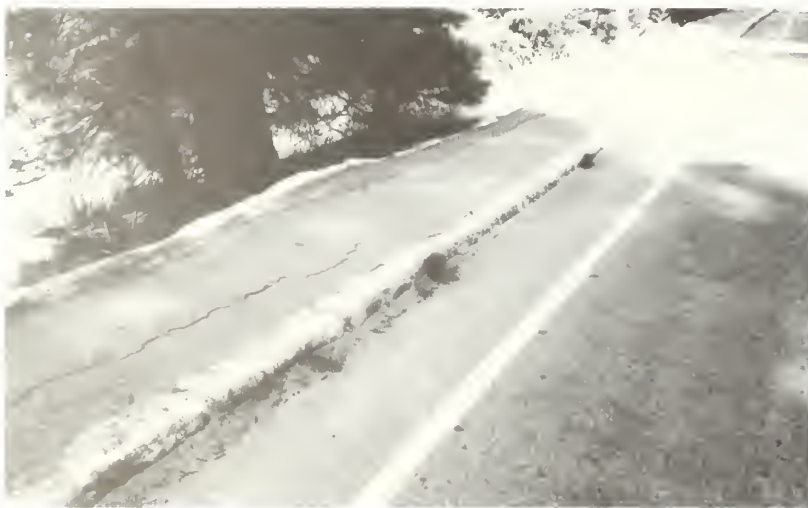
Asphalt sidewalk along Generals Highway in Giant Forest showing deterioration
