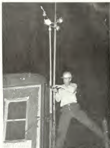
The anemometer is mounted which provides wind data that is crucial to forest fire suppression.
