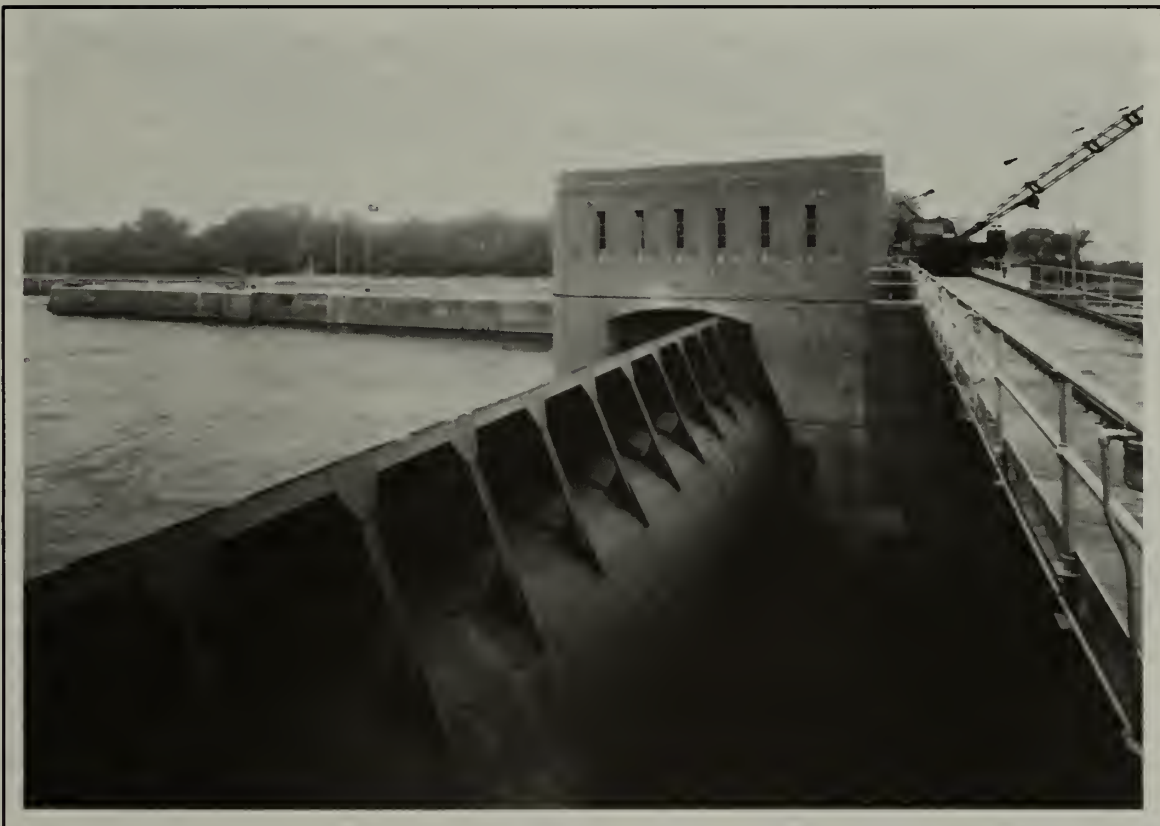
An early improvement to roller gate design was the attachment of a curved steel apron to the side of the gate, which reduced the required drum diameter and formed a more reliable and waterproof seal. Dam No. 5A. (Clayton B. Fraser, Fraserdesign)
