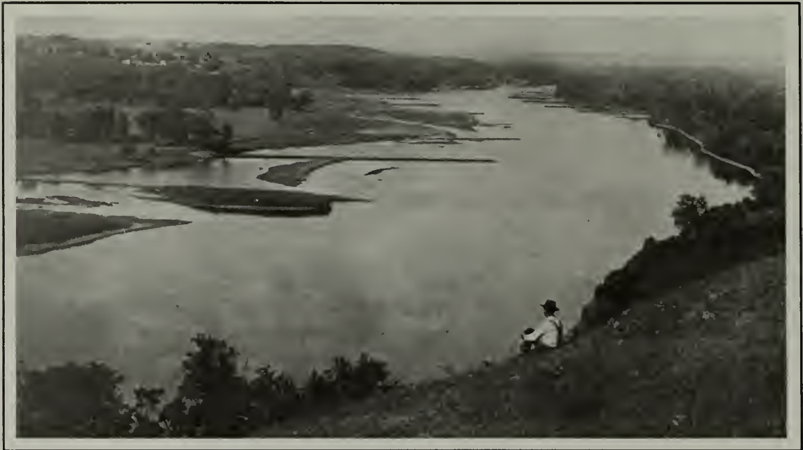
Wing dams, the fingerlike extensions seen on both sides of the river in this historic photograph, constricted the river's flow, thereby speeding the current and providing a clear channel. From "Wingdams Below Ninninger, Minn., 1891," one of a series of photographs of the Mississippi River taken by H. Bosse, draughtsman with the Corps of Engineers, 1883-1891. (U.S. Army Corps of Engineers, St. Paul District)
