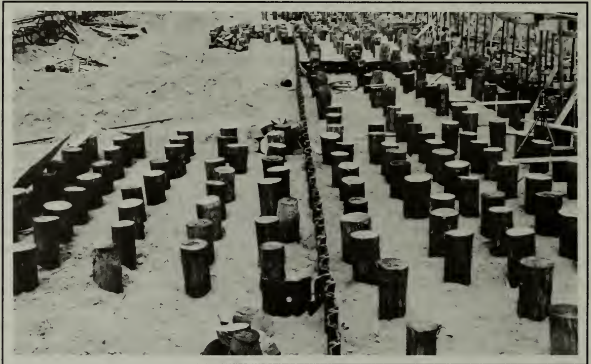
The Corps conducted numerous tests to determine the load-bearing capacity of pile-founded structures. The results of those tests often resulted in the redesign of the lock and dam structures, as was the case at Lock and Dam No. 25. Driven Pilings at Dam No. 25, May 1938. (U.S. Army Corps of Engineers, St. Louis District)
