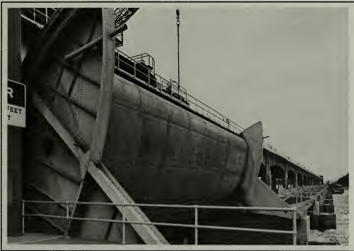
Dam No. 24, Submersible Elliptical Tainter Gate. The shields on the ends of the gate prevent water from seeping between the gate and the piers. Typical of later gate designs, the gate armature on Dam No. 24 is solid. Earlier designs, such as Dam No. 8 pictured on the opposite page, featured open framework. (John P. Herr, John Herr Photography)
