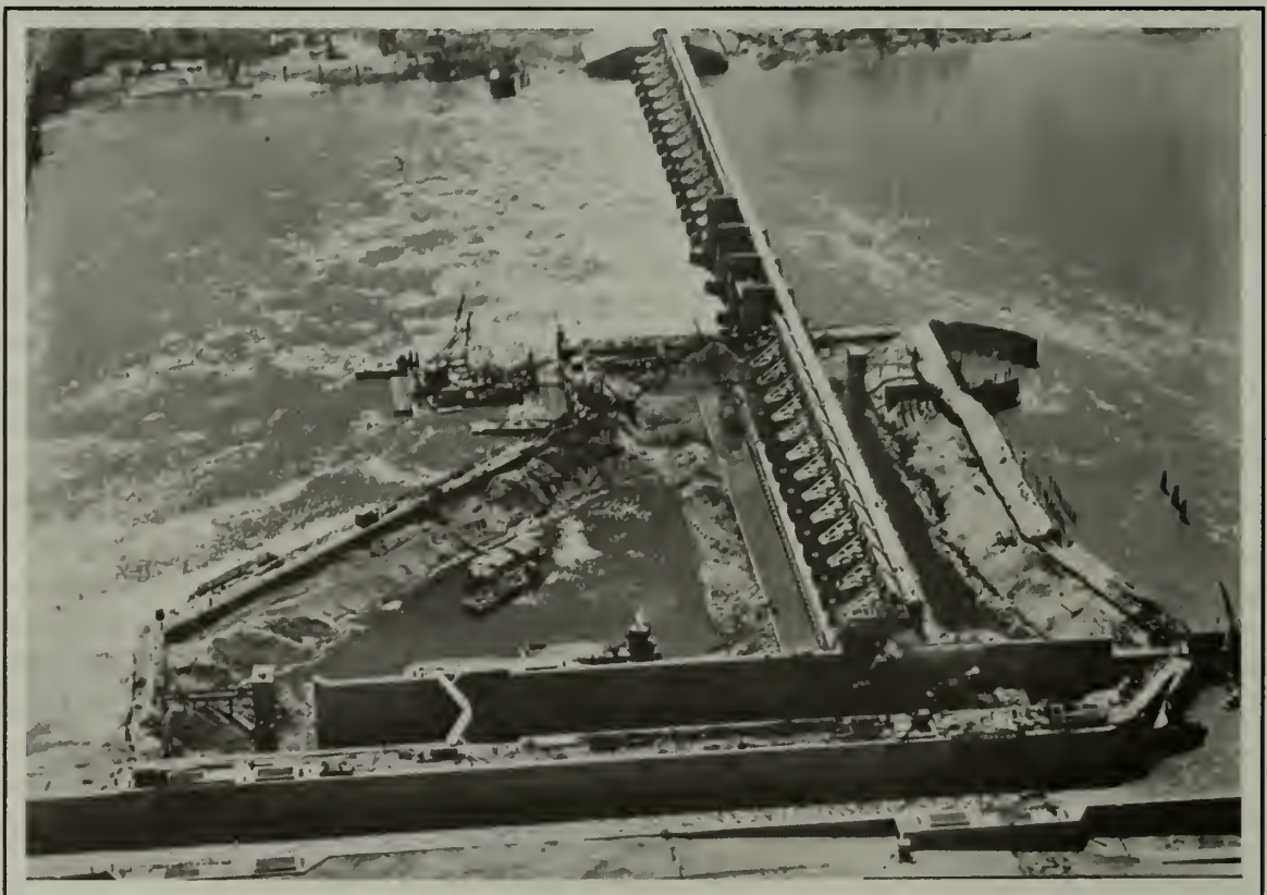
(Above) Tainter Gate Assembly on Dam No. 26, December 1935. (Below) Aerial view of cofferdam surrounding Dam No. 26, August 1937. (Both photographs: U.S. Army Corps of Engineers, St. Louis District)
