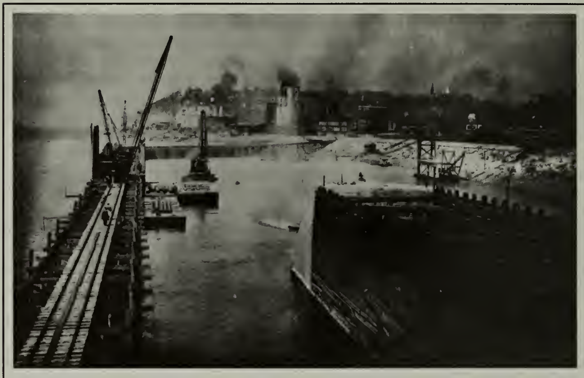
A cofferdam walls off a portion of the river, providing a dry work site. Each contractor was responsible for the design of his own cofferdam. Griffiths & Son, the contractor for Main Lock No. 26, began by building a trestle along the center line of the cofferdam site. The trestle supported derricks and cranes that aided in construction and the delivery of materials. Cofferdam Construction for Main Lock No. 26, March 1934. (U.S. Army Corps of Engineers, St. Louis District)
