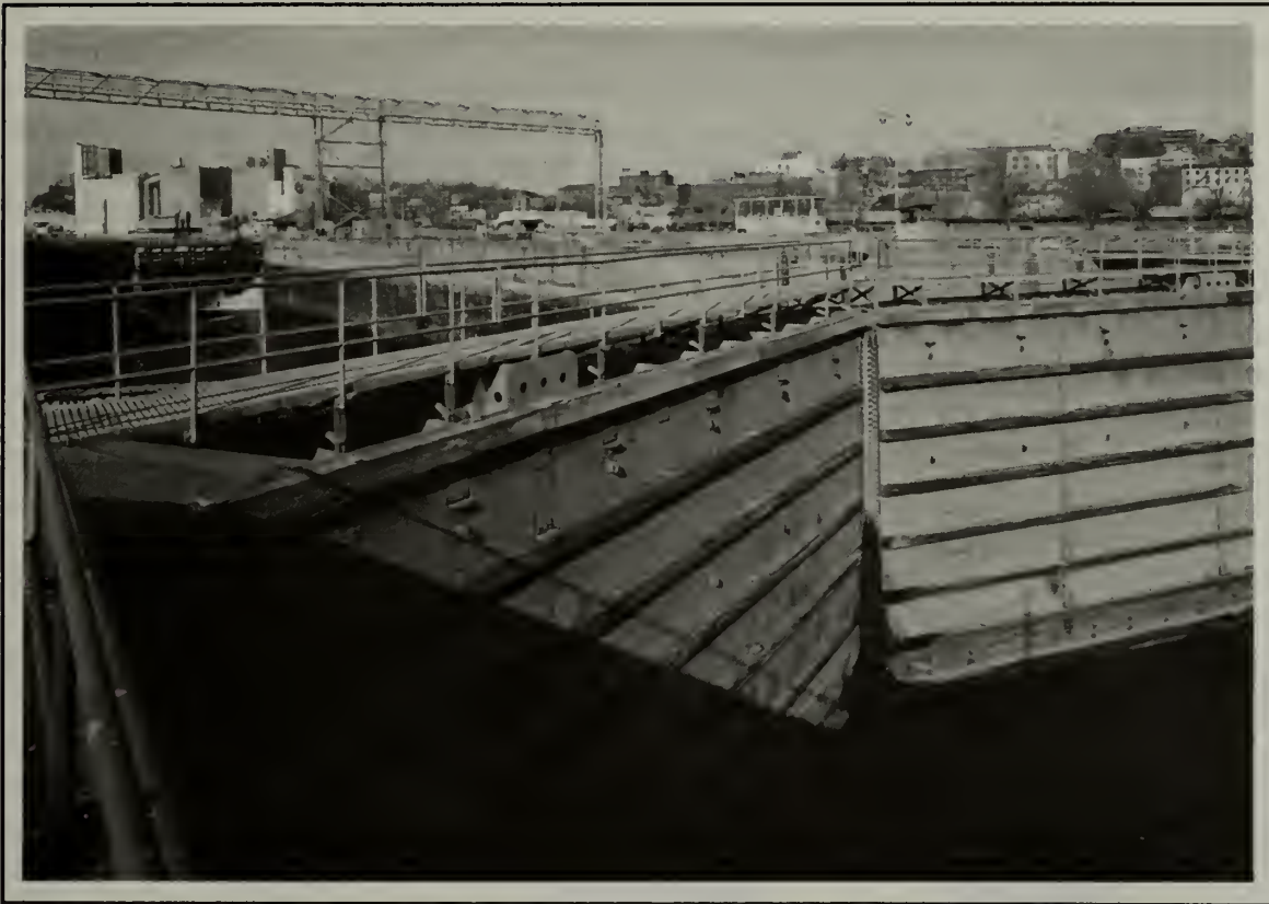
Miter gates are electrically operated. Motor assemblies housed in machine pits in the lock walls power the arms and gears which open and shut the gates. The lockmaster controls each pair of gates independently by switches located in weather-proof cabinets on the lock walls. Miter Gate on Auxiliary Lock No. 26. (John P. Herr, John Herr Photography)
