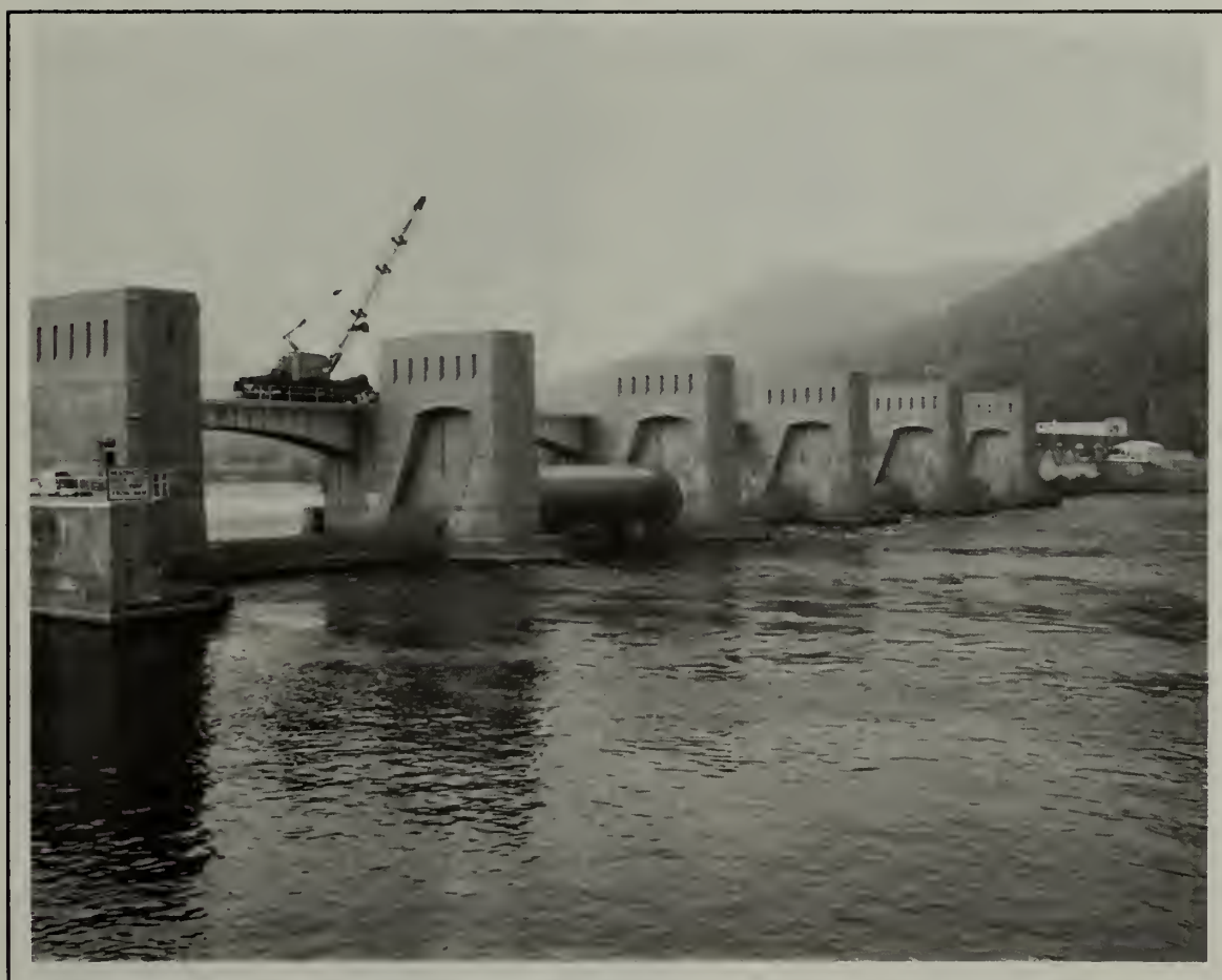
The pier houses of the Moderne, post-1936 structures are incorporated into the overall pier design of the dam structure. The roofs are flat, and the buildings have slit, three-pane windows. Dam No. 5A. (Clayton B. Fraser, Fraserdesign)
