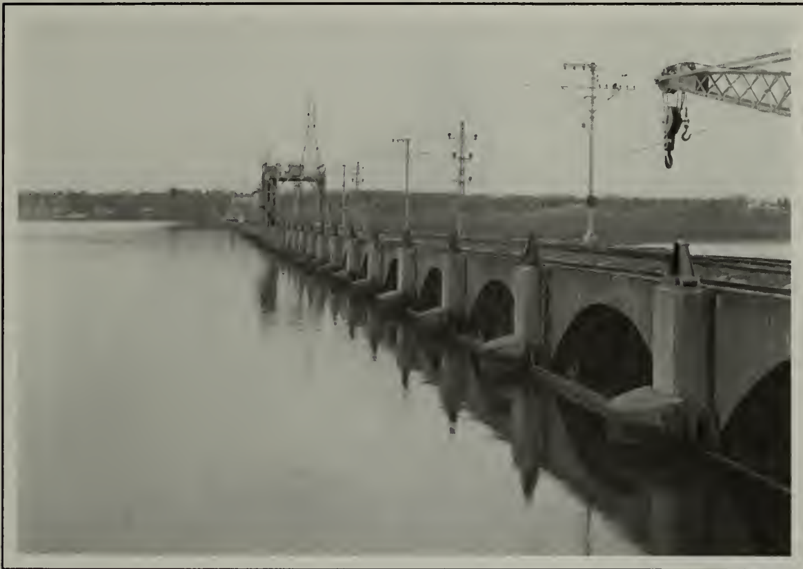
The Keokuk dam, which is privately owned, has 119 rectangular sliding gates, located between 120 piers on 36-foot centers. (Peter A. Rathbun)
