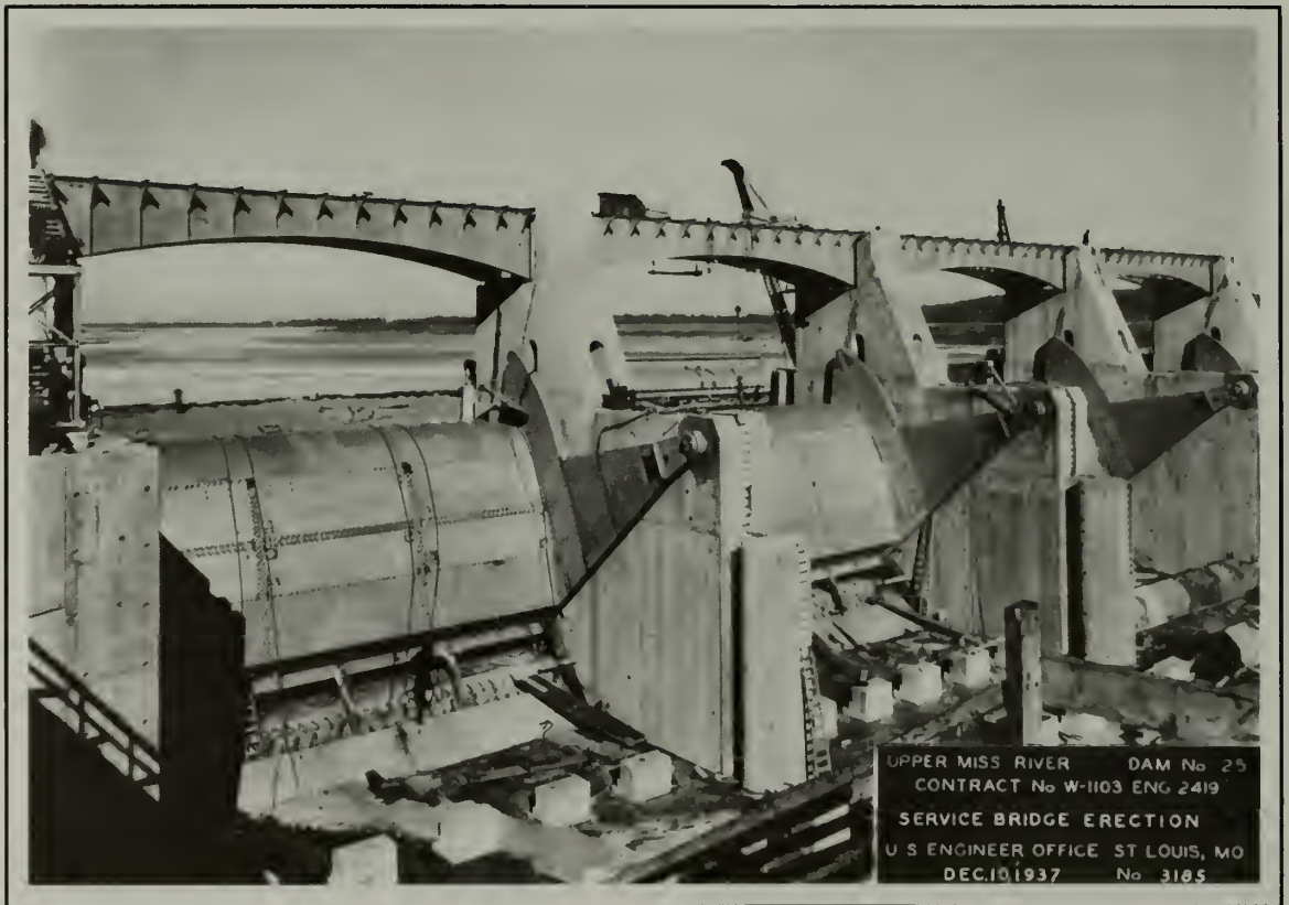
The construction of Dam No. 25, which has truncated elliptical Tainter gates, December 1937. (U.S. Army Corps of Engineers, St. Louis District)
