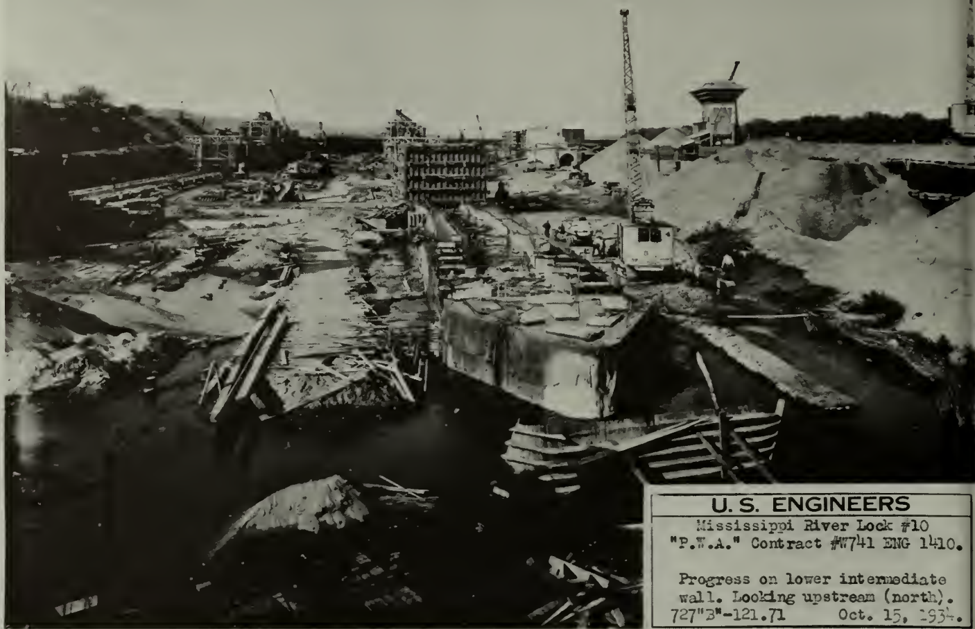
(Above) Construction of Lock Wall, October 1934. (U.S. Army Corps of Engineers, St. Paul District)
