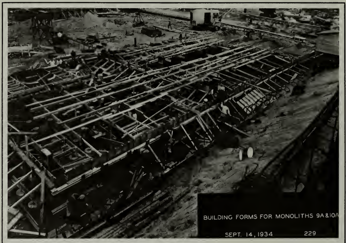
After the piles were driven, workers began building the monolith forms used for concrete placement of the lock walls. Construction of Main Lock No. 26, September 1934. (U.S. Army Corps of Engineers, St. Louis District)
