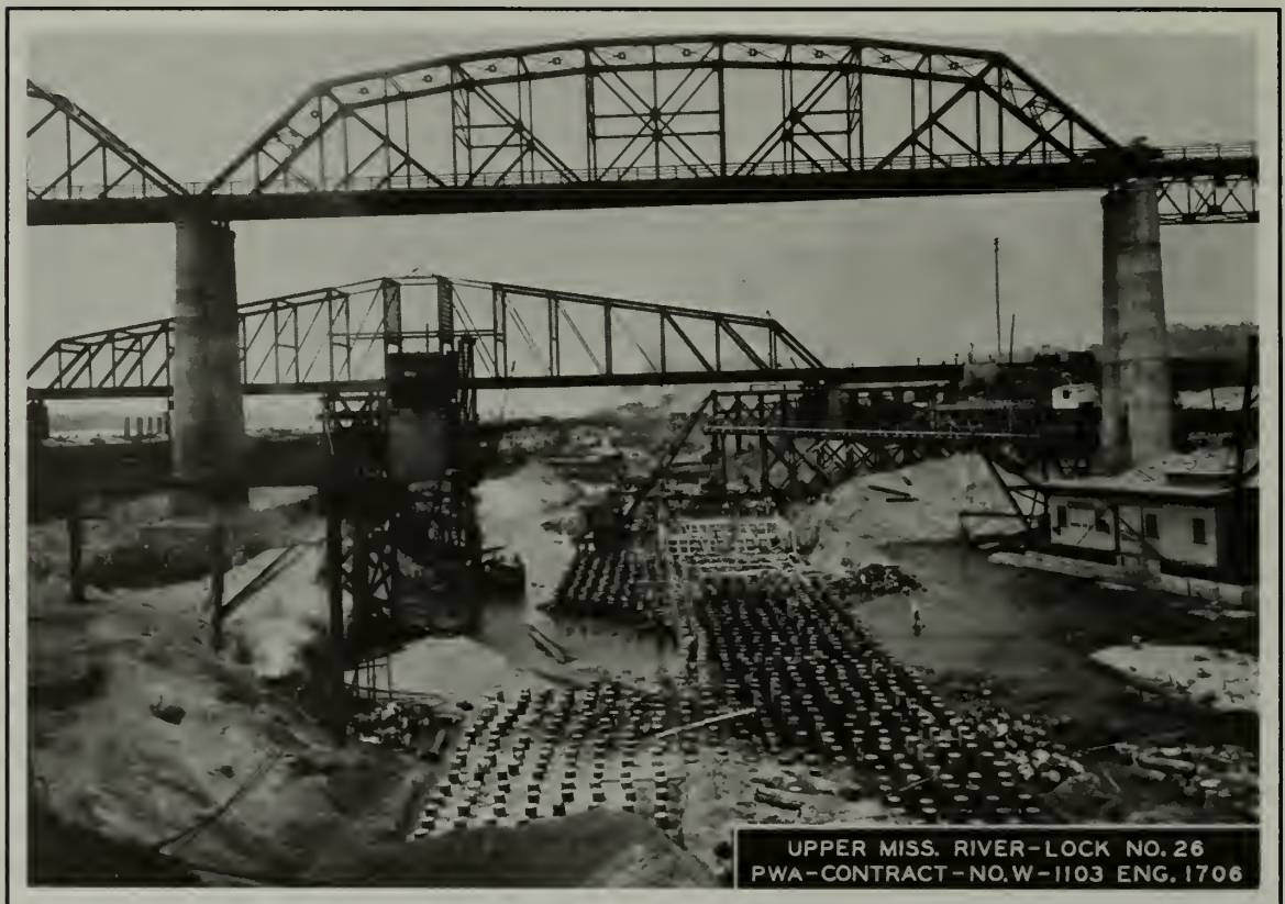
The contractor began draining the cofferdam in May 1934; pile driving began the next month. By the end of October, all pile driving was completed. View upstream from cofferdam, October 1934. (U.S. Army Corps of Engineers, St. Louis District)
