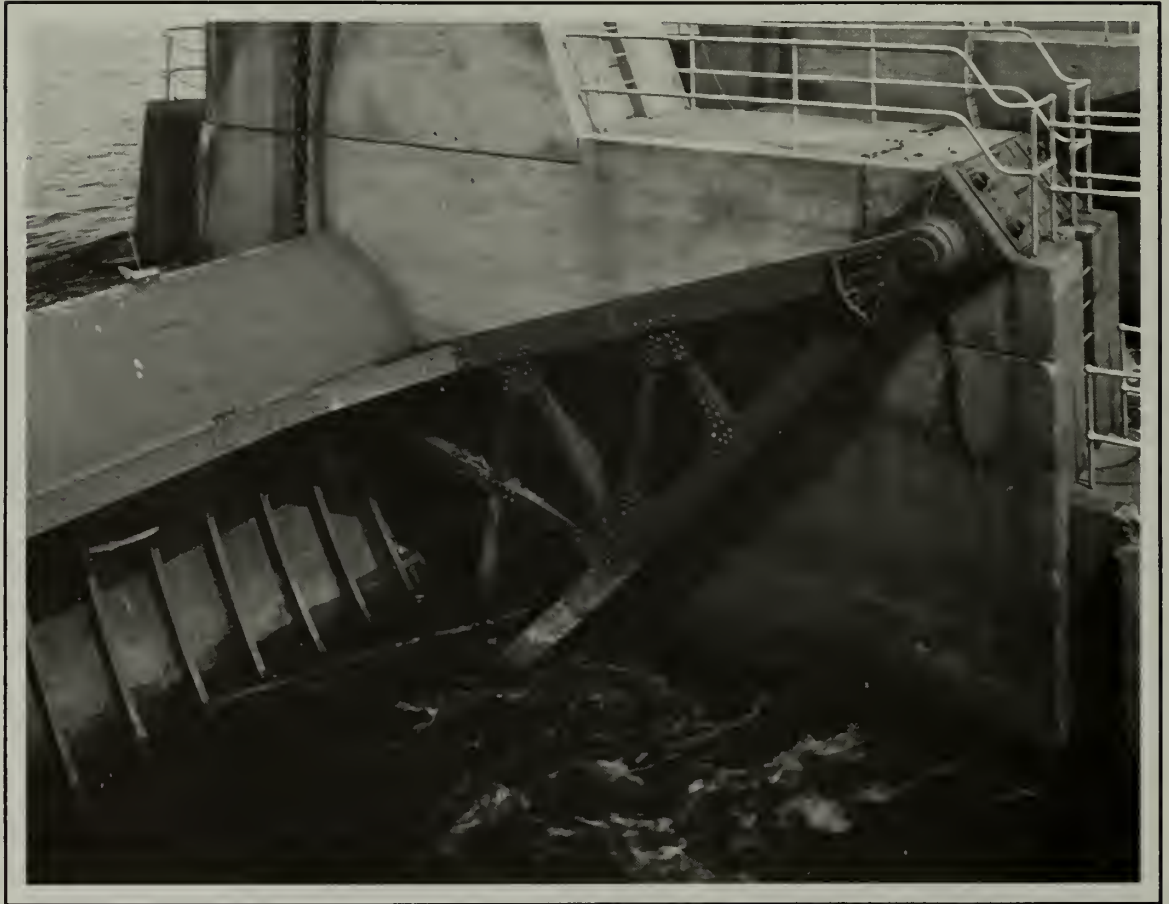
The first form of Tainter gates used on the 9-foot channel had steel plating only on the water-side face of the gate. A submersible gate, such as this one on Dam No. 8, can be distinguished by the additional overflow plate on the top of the gate, which provides a streamlined surface for breaking through the water. Dam No. 8, Submersible Tainter Gate. (Clayton B. Fraser, Fraserdesign)
