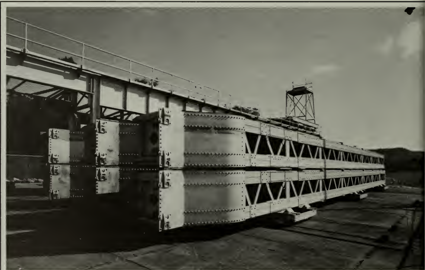
(Below) Roller Gate Bulkheads, Dam No. 6. The individual gate bays on the dam can be closed off with bulkheads and then drained for repairs. (Clayton B. Fraser, Fraserdesign)
