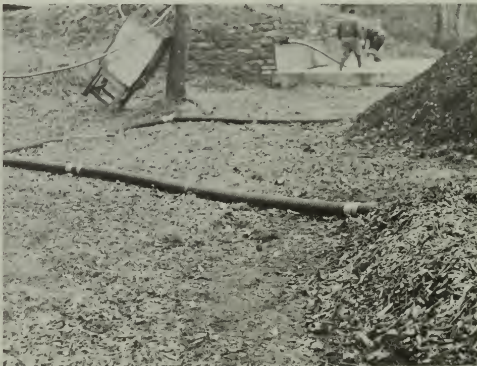
Perforated piping and the mattress are in place at the right, while the solid (non-perforated) piping connects perforated piping of the pile.
