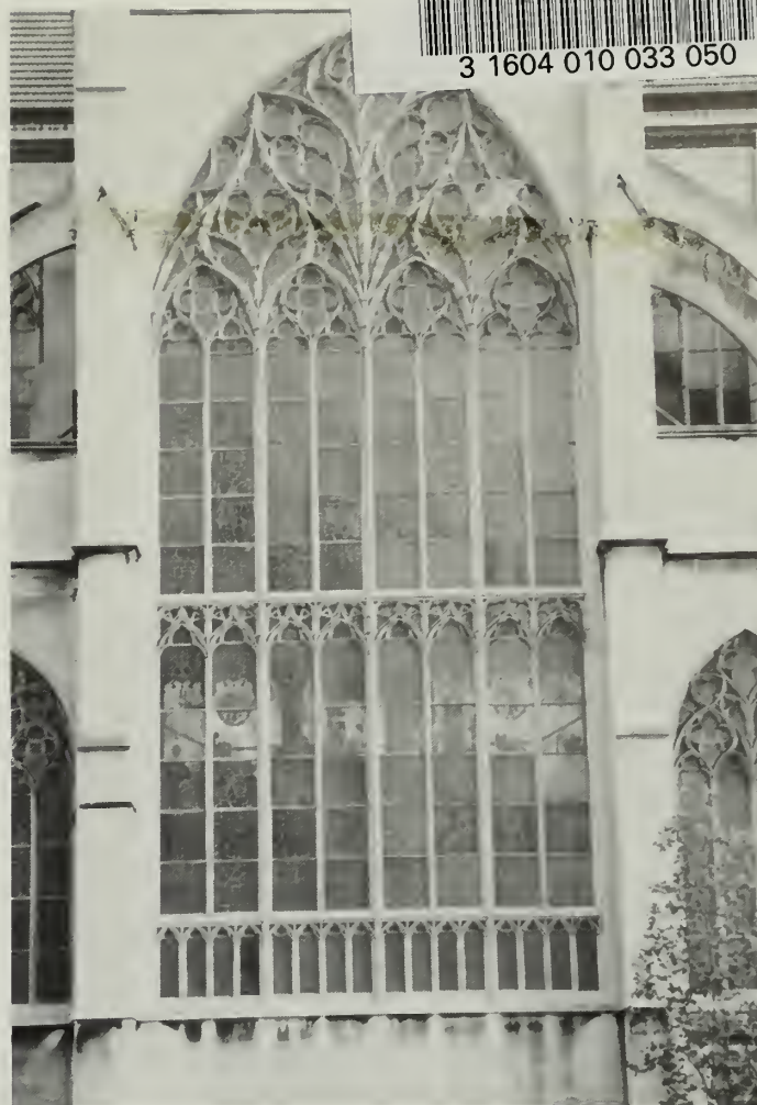
Figure 20. (a) The aluminum frame grid used for protective glazing totally disregards the original tracery of this Neo-Gothic church. The grid mars the appearance of the window inside and out. It also impairs the overall historic character of the building. (b) Protective glazing in this instance preserves both the appearance of the window and its contribution to the building. The latter building is the Cathedral Basilica of the Assumption (St. Mary's Cathedral), Covington, Kentucky (1895-1910). The window, 67' x 24' (20.4m x 7.3m), is among the largest stained glass windows in the United States. Photos: Neal A. Vogel.
