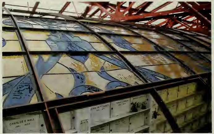
(b). Before repairs began on the vaulted glass ceiling below, a new diffusing skylight was installed to correct recurring leaks. Catacombs (ca. 1920), Cypress Lawn Memorial Park, Colma, California. Photo: Neal A. Vogel.
