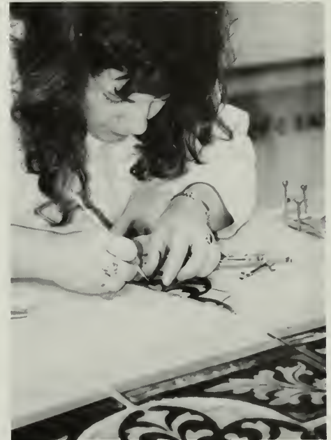
Figure 15. New stencils are used to produce matching replacement glass for repetitive stenciled patterns in a ca. 1870 window. Photo: Neal A. Vogel.
