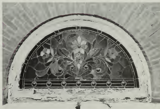
Figure 5. Stained glass is an exterior feature as well as an interior one. As part of any preservation project, stained glass should be photographed from the outside as well as the inside. The frame of this Aesthetic Movement window (circa 1880) needs repair. Photo: Neal A. Vogel.
