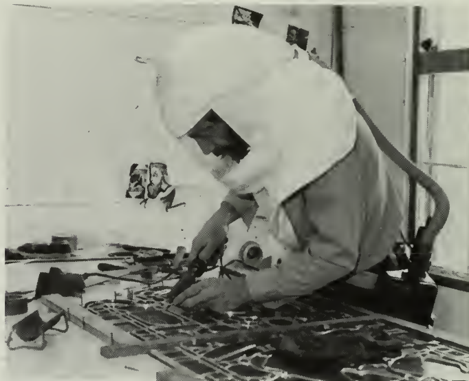
Figure 18. A craftsman releads a window. The full hood offers protection from lead fumes. Photo: Neal A. Vogel.
