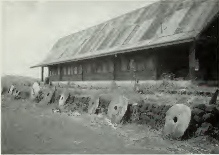
Tomil Pebai. This is a traditional structure called a pebai, built with non-traditional materials. The walls are of concrete block, the floor concrete. The Yap Cultral Inventory Group found that the structure itself has no traditional importance to Yapese. Non-Yapese may find it surprising that the Yap Cultural Inventory Group found that the site of this pebai, a stone platform lined with Yapese rhuul or "money" is of no traditional importance to Yapese. (photograph, Yap Culture Inventory Group, 1989)
